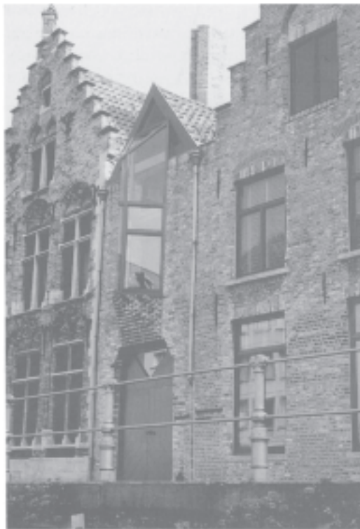
Fig. 1.6 Bruges in Belgium is a successful example of urban conservation. Most of the historic architecture has been restored and modern buildings successfully incorporated into the historic fabric.
