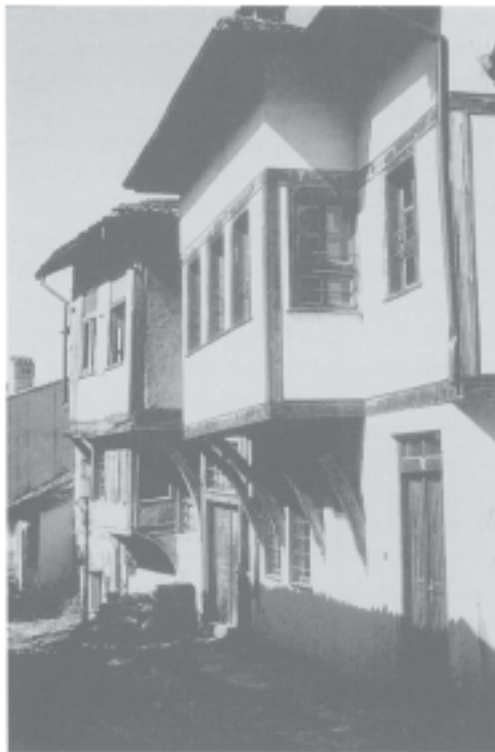
Fig. 4.1 In Plovdiv, Bulgaria, it was the former Communist government who took on, paid for and controlled the immaculate restoration of the historic fabric, which also involved the decision to relocate residents.
