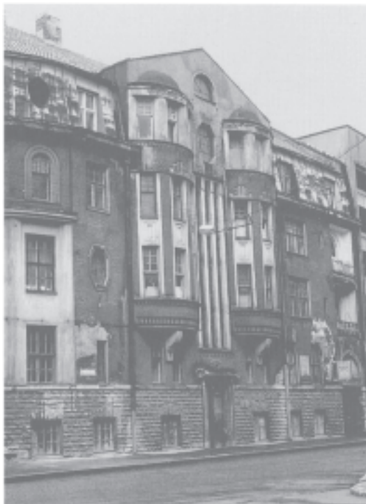
Fig. 1.8 An entire quarter of Art Nouveau buildings are rapidly decaying in Tallinn, Estonia, while ownership disputes and severely limited finances curtail the work of architecture and planning departments.
