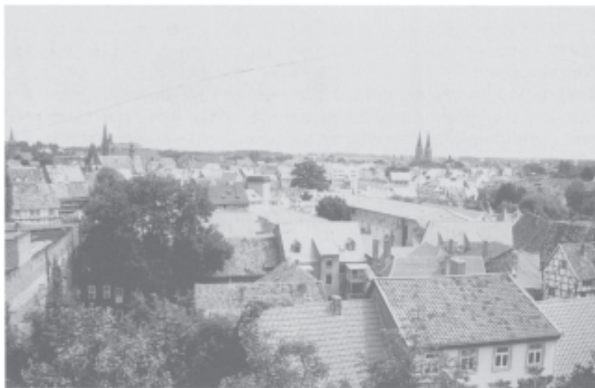
Fig. 2 For many visitors, the first view of Quedlinburg is from the Schloßberg. The local authority advocates the retention of the characteristic steep roofscape.
