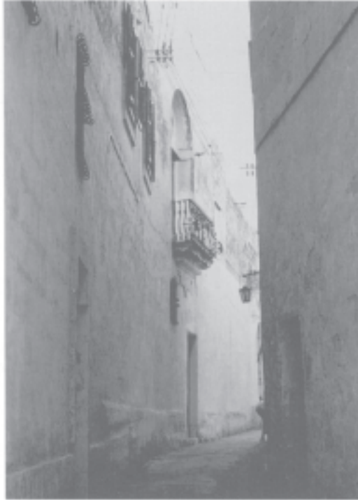
Fig. 1 (a) and (b) Mdina is still a typically Islamic town in its urban morphology, with high walls and narrow winding streets.
