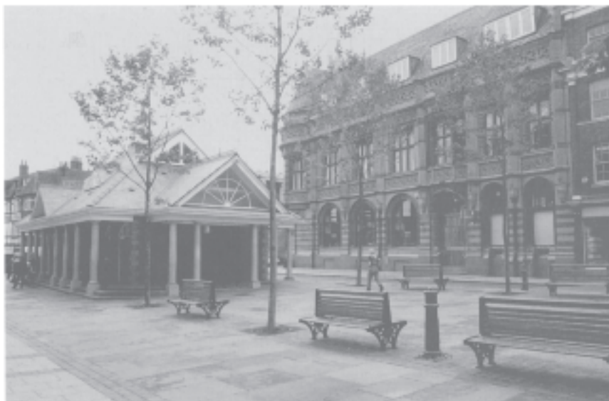
Fig. 6.15 Visitor facilities like these public toilets in York do not have to use an 'historical' stylistic language.
