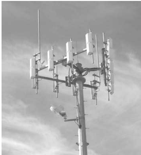
Figure 16.5 Sectorized base-station antenna.
