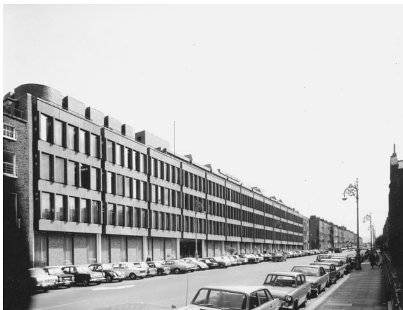
Fig. 4.2. Exterior of ESB headquarters, Fitzwilliam Street. Image courtesy of Norman McGrath.
