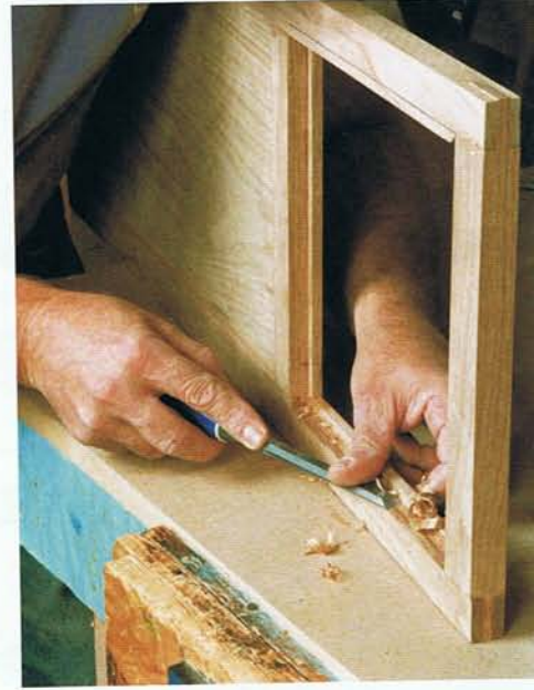
Rear wall of groove is removed to accept glass (above).
