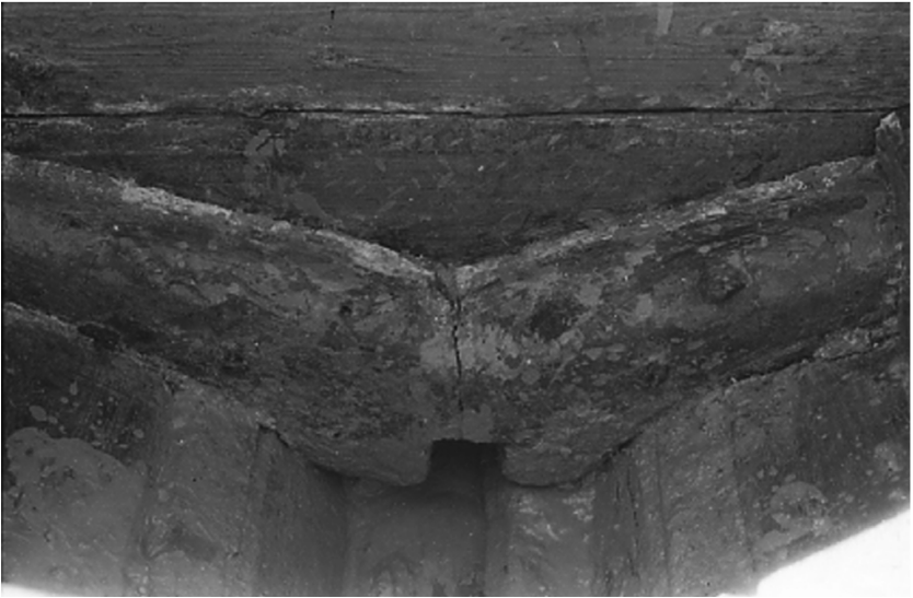
Figure 4.17. Top view of bulkhead no. 1, which has original half frames ( top ). Large half frames were attached to the bulkheads ( bottom ). (New photo [top] by author; older photo [bottom] courtesy of Museum of Overseas Communication History)
