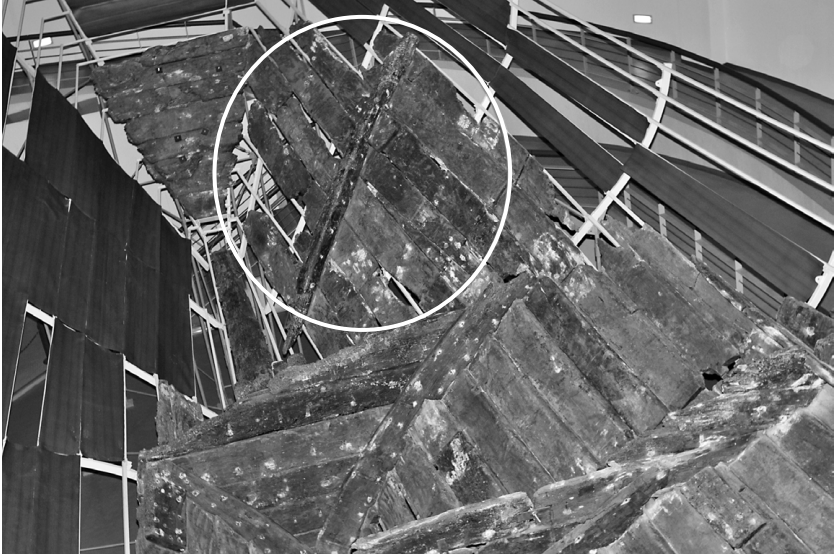
Figure 5.7. Baulk on the inside at the starboard bow. (Photo by author)
