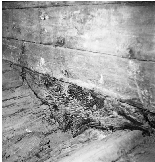
Figure 4.15. Bilge boards (or bottom ceiling planks) and the degraded bottom bulkhead plank. (New photo [above] by author; older photo [right] courtesy of Museum of Overseas Communication History)
