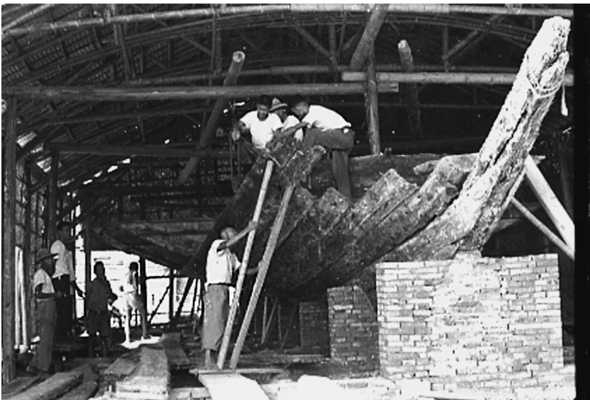
Figure 4.3. Reconstruction of the dismantled hull of the Quanzhou ship at the Kaiyuan Temple. (Courtesy of Museum of Overseas Communication History)
