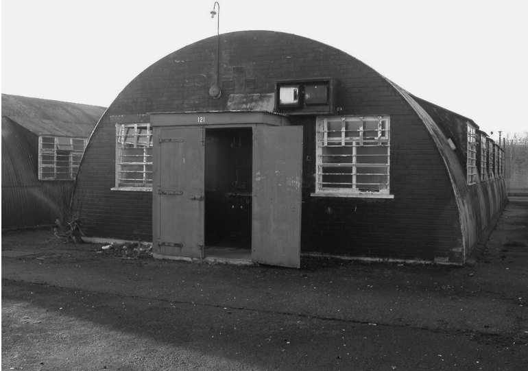
Figure 5.3 The exterior of a Nissen hut from the Compounds, c.2005.
