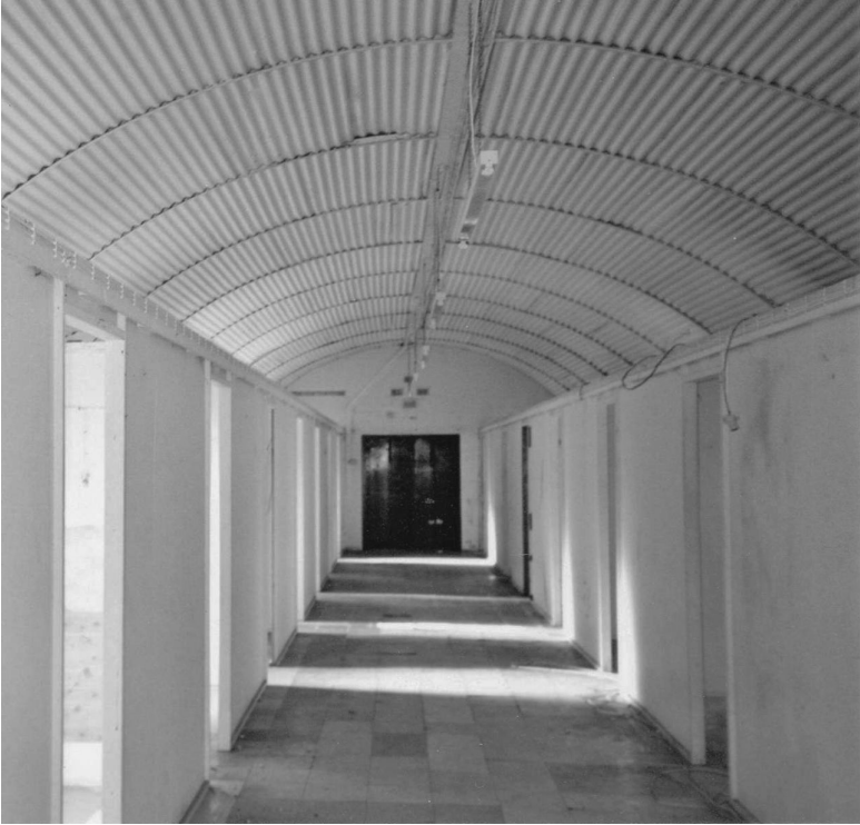
Figure 5.4 Image of interior of Nissen hut with partitions in place.
