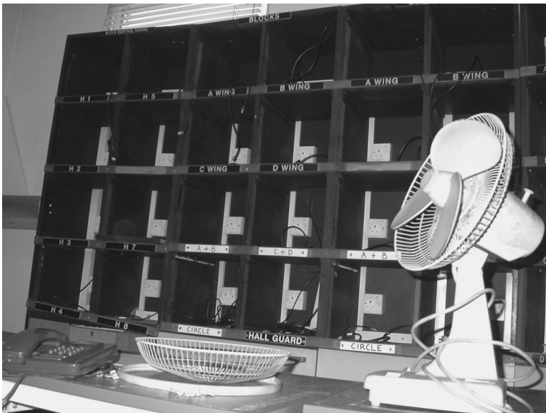
Figure 4.9 Central Observation Room of H-Block Administration Block, c.2006.
