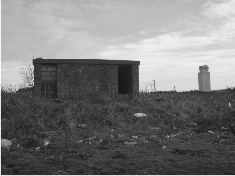
Figure 5.2 Dilapidated shed, site of Long Kesh/Maze, c.2005.
