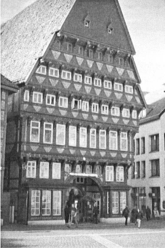
Figure 7.9 This property replicates one that once existed on the site, but Hildesheim was largely destroyed in World War 2, and the rebuild did not include this building. When the site became vacant in the 1980s local people were consulted and this replica was executed. One problem is that finding timber of sufficient quality is now very difficult, and the beams are badly cracked.
