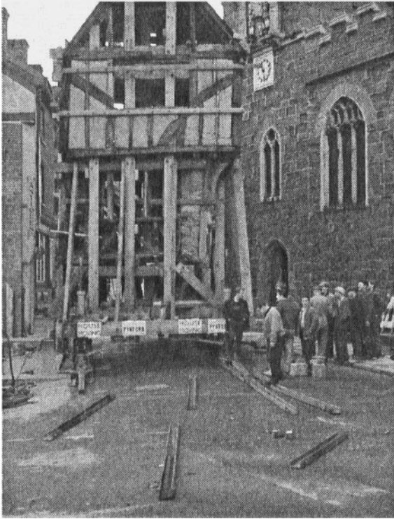
Figure 8.10 This building stood in the way of a new road, so it was moved to a new site, bodily, in 1961. Some material authenticity may be retained, but that of place has been lost.
