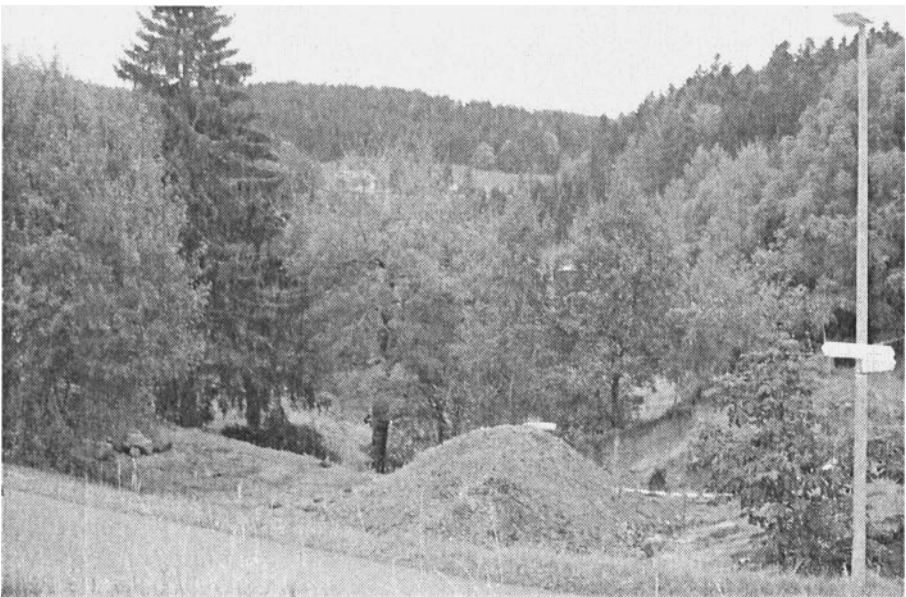
Figure 6.10 In Germany many people follow rivers to their sources, hence their source springs have particular significance. In this case there is no fresh spring but a rather boggy area caused by water welling up, so a new spring is being dug out and constructed.
