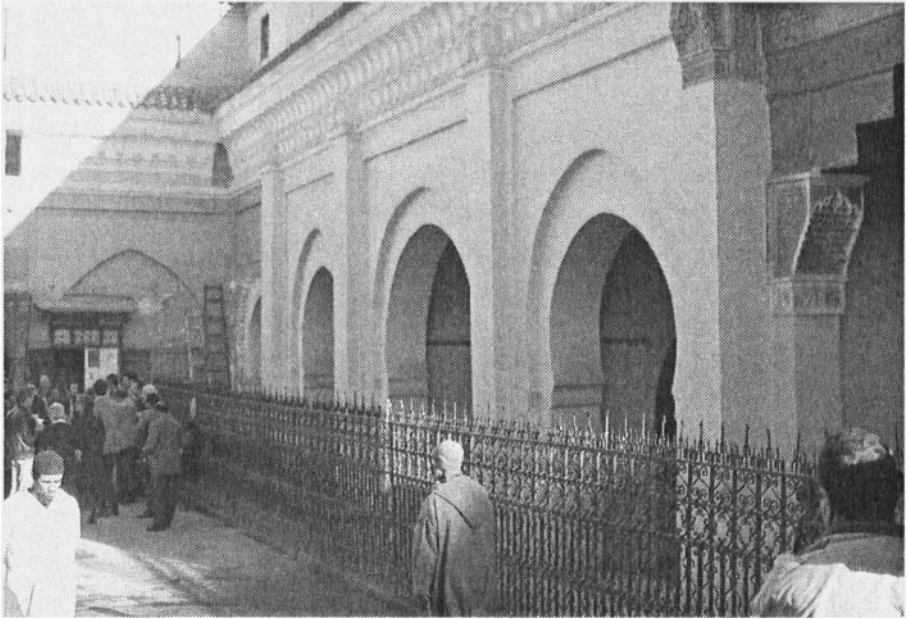
Figure 8.16 A beautifully restored fountain, yet the fence ensures that people are unable to approach it and use it for its original purpose.
