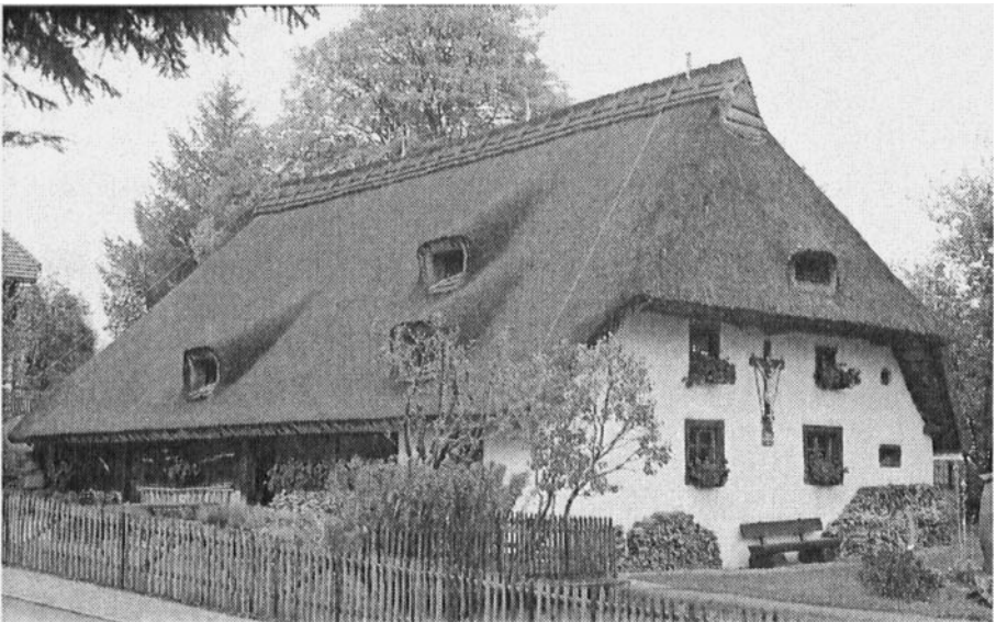
Figure 8.9 This vernacular property in the Black Forest has been restored as a museum, though in situ . Problems of modern living, health and safety are thus circumvented. Few people today would tolerate living where the smoke from the fire simply finds its way through the thatch, curing the sausage and bacon en route .
