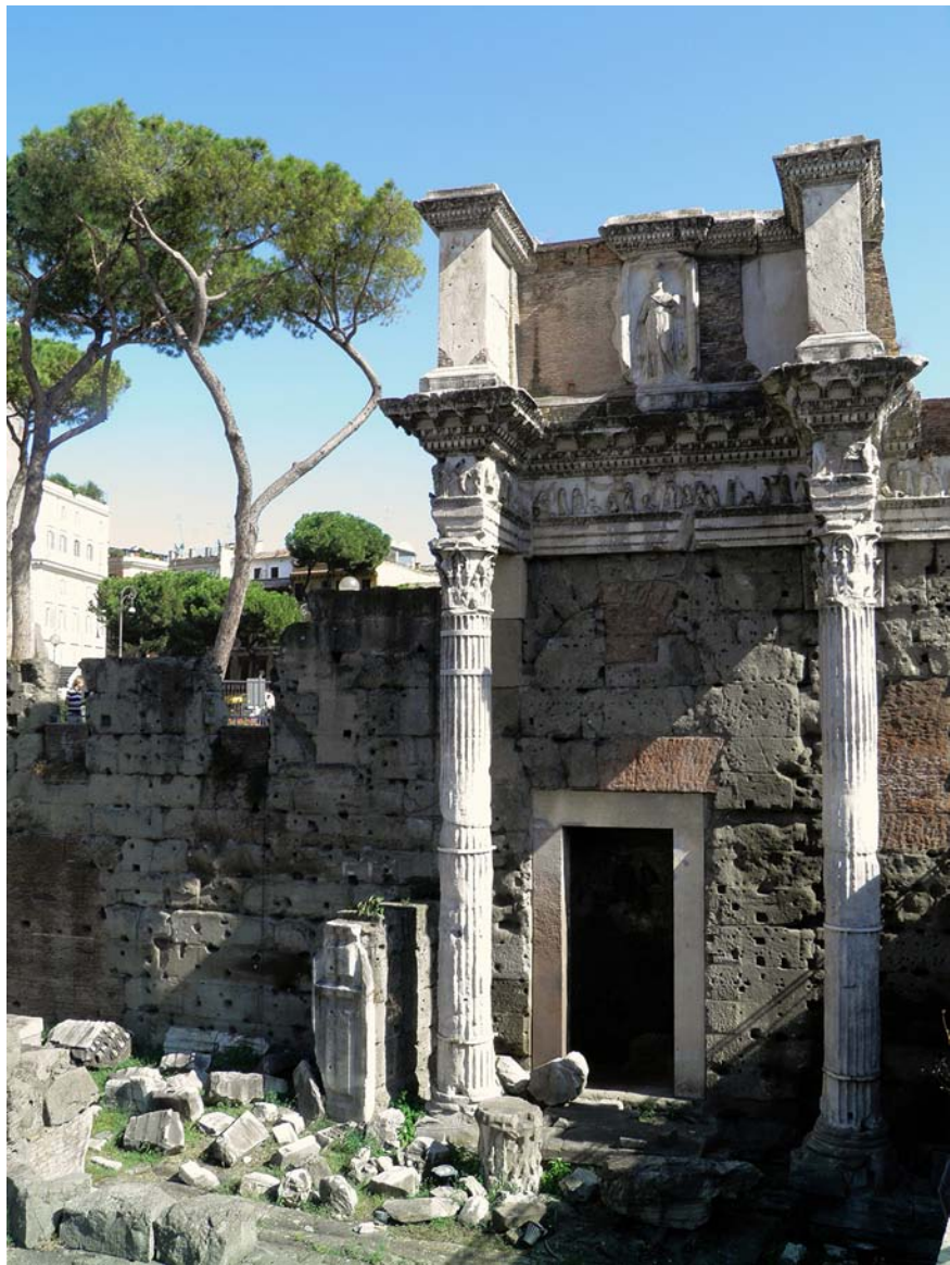
FIGURE 6.1 Rome, Forum of Nerva, section of the South colonnade known as le colonnacce.
