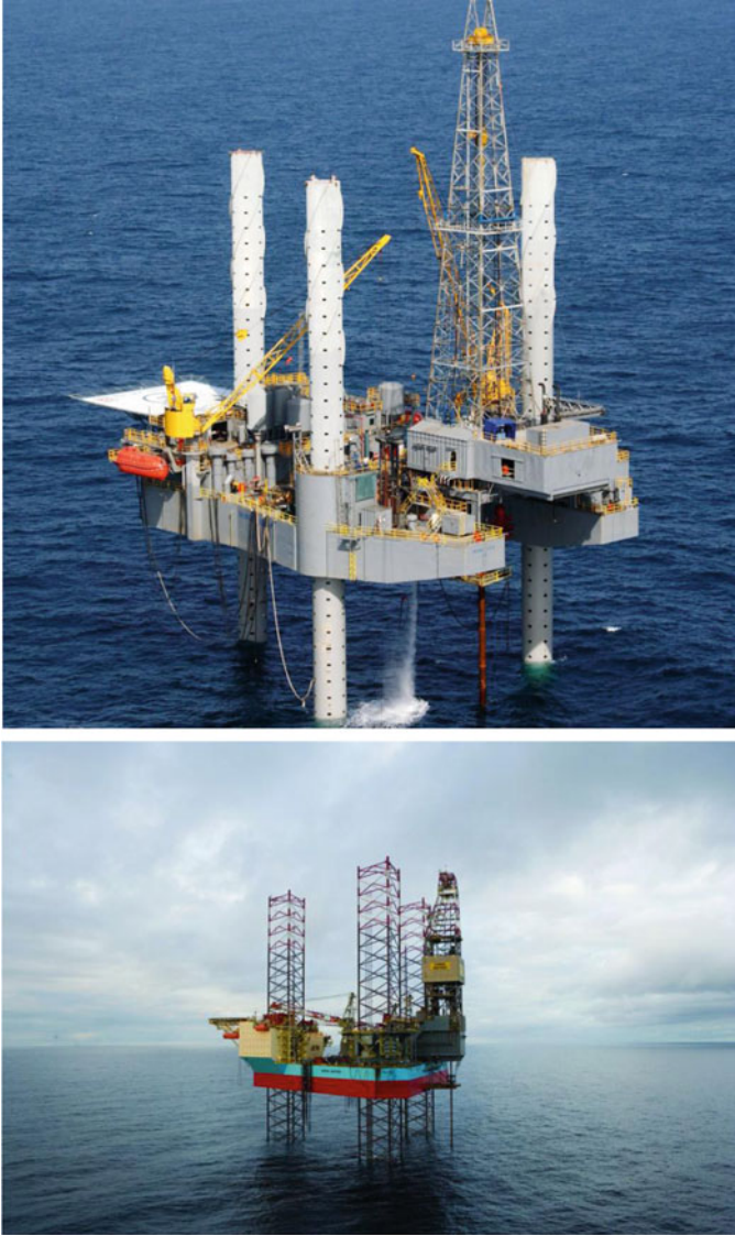
Fig. 10.7 Cylindrical and trussed legs on the Bethlehem MS-225 Spartan 202 and Gusto MSC CJ 70 Maersk Inspirer (Source: Spartan Offshore; Maersk)
