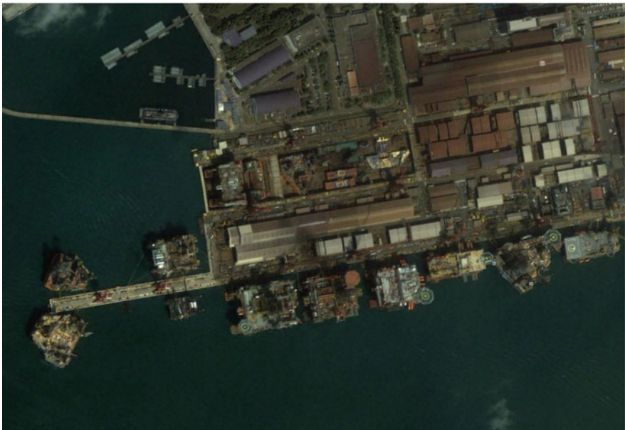
Fig. 9.5 Keppel's Pioneer shipyard layout and satellite view circa 2011. In the satellite view, three jackups, five semis, and one liftboat are in quays (Source: Keppel, Google)
