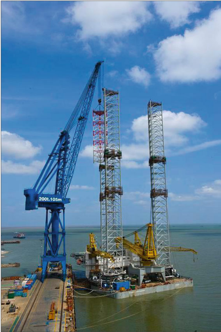
Fig. 11.9 Top section of F&G Super M2 leg installed (Source: Remedial Offshore)
