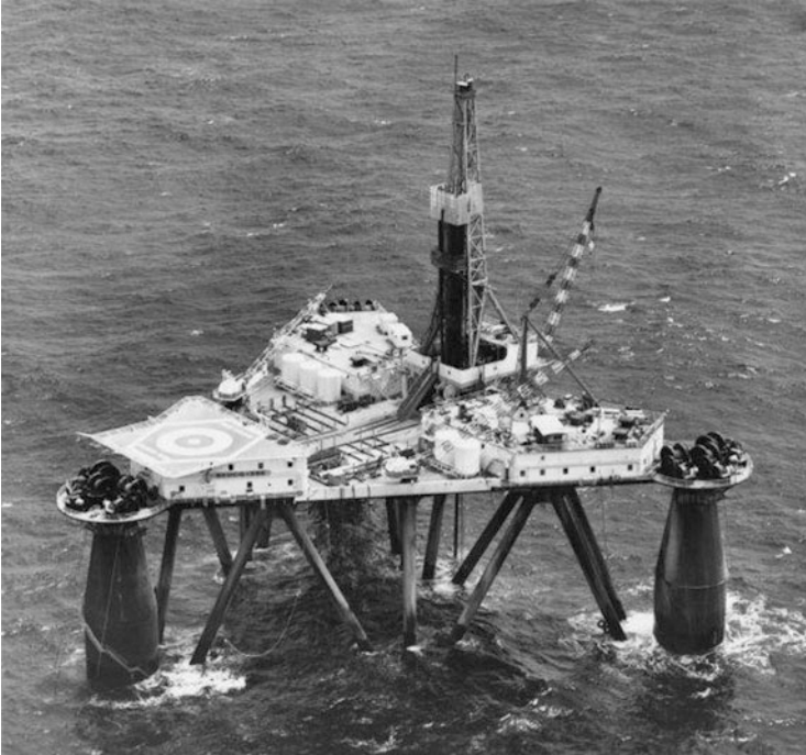
Fig. 1.14 The SEDCO 135-E , a first generation semisubmersible built in 1967 (Source: National Library of Australia)
