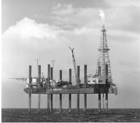
Fig. 10.5 Early jackup rig Sea Gem in 1964 (Source: O. Buggee)
