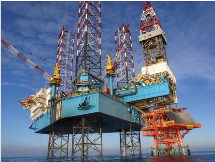
Fig. 10.12 Cantilever drilling rig operating over a fixed platform (Source: JDC)
