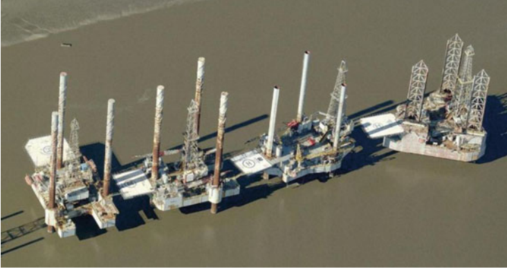
Fig. 1.23 Four cold-stacked rigs in Sabine Pass, Louisiana (Source: Microsoft)
