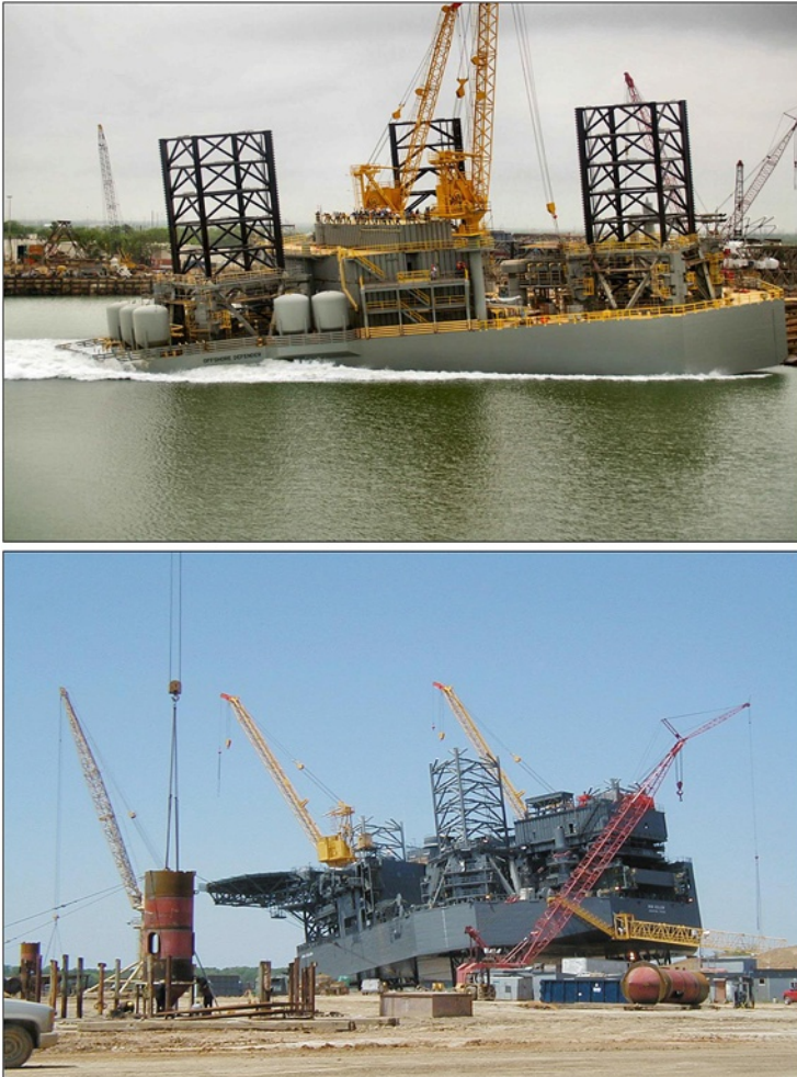
Fig. 11.8 Launching rigs at the AmFELS shipyard ( top ) via slipway and the LeTourneau shipyard ( bottom ) via walking (Source: Keppel; Pitts)
