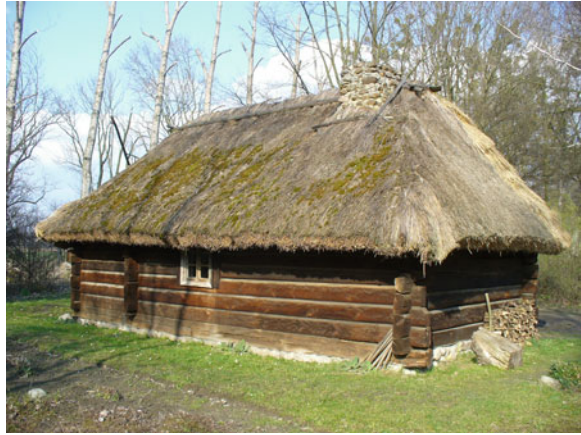
Fig. 3.17 Traditional type of log construction
