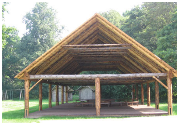
Fig. 3.29 Post and beam structural system
