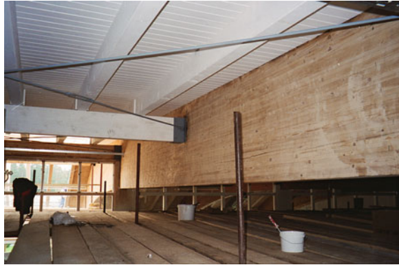
Fig. 3.5 Renovated primary glued-laminated beams in the smaller thermal pool
