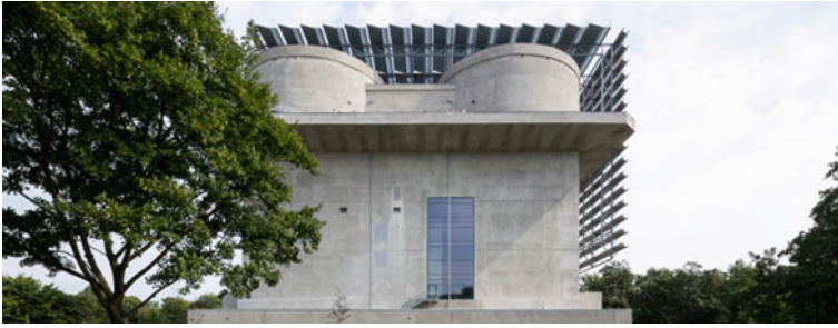
Fig. 3 Wilhelmsburg Energie Bunker (Source Special knowledge pool: www.special.eu )
