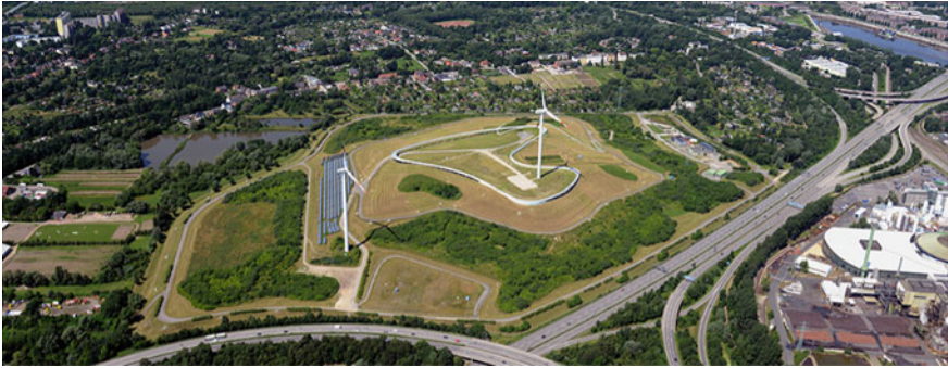
Fig. 4 Aerial view of Wilhelmsburg Energie Colline Georgswerder (Source Energy Atlas IBA—Hamburg)
