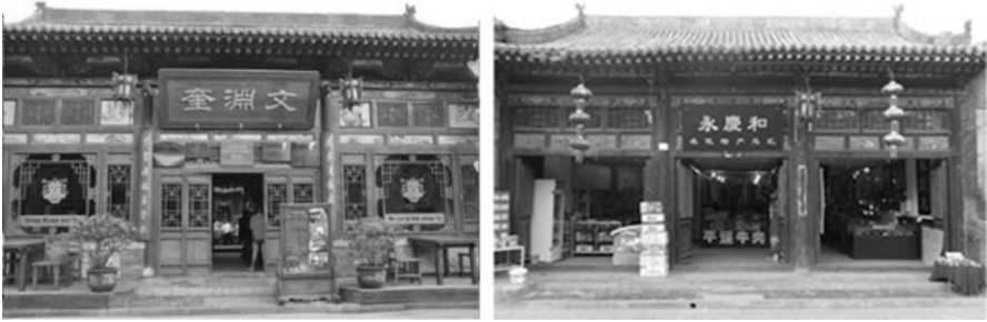
Fig. 3 Compound facade renovation along the streets in Pattern 4 (The first photography keeps the original facade form and expands the windows to show the inner space of the hostel. The second one changes the windows to doors on the facade)
