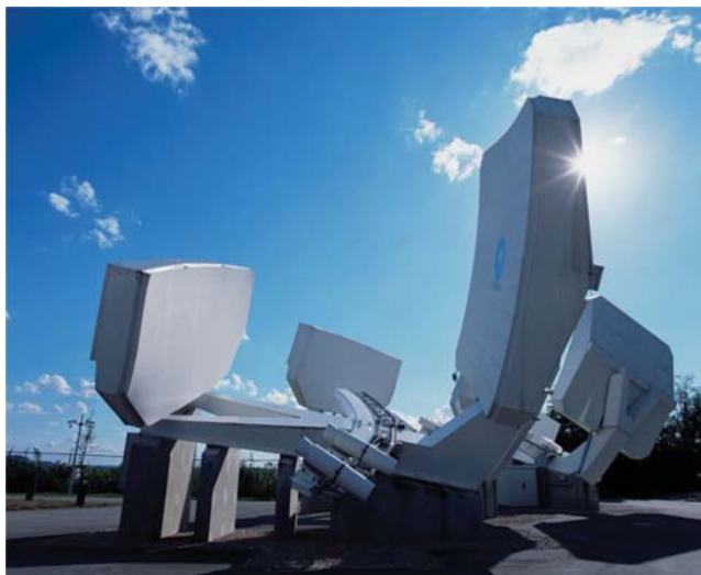
Figure 10.12 Multibeam earth stations at SES-Astra in Luxembourg. Each antenna covers a 40-degree field-of-view of the geostationary satellite arc. Source: Reproduced with permission from SES-ASTRA
