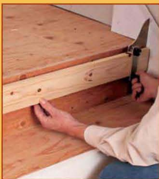
46 | Fitting the Risers and Treads
