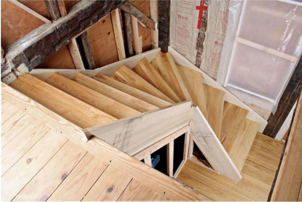
Winders climb rapidly at corners. Making the most of space, winders pack multiple risers into the same space as a landing would take.
