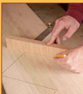
80 | Laying Out the Stringers
