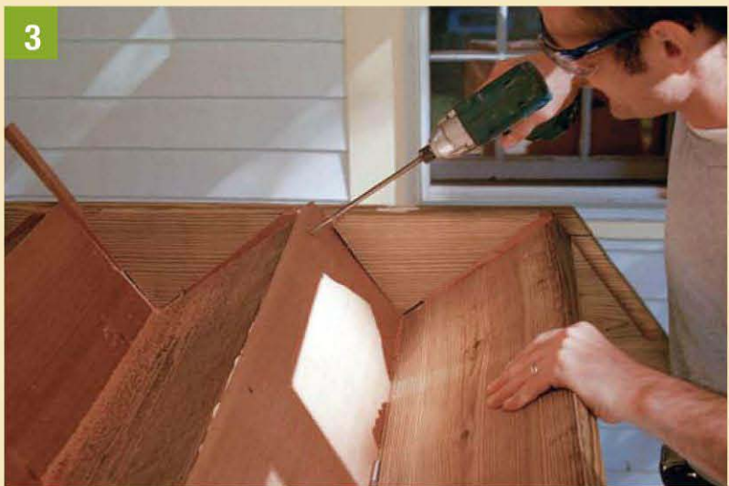
3 Stainless-steel deck screws join the riser to the back of the tread.
