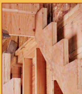
33 | Installing the Stringers
