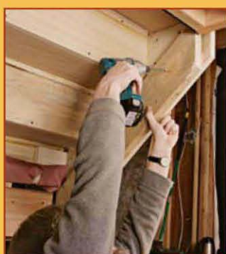
90 | Installing the Stair
