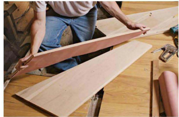
Preventing squeaks. Rosin paper, often used between hardwood flooring and the plywood subfloor, acts as a slip membrane to allow some movement between the subthread and the tread, while minimizing the potential for squeaks.
