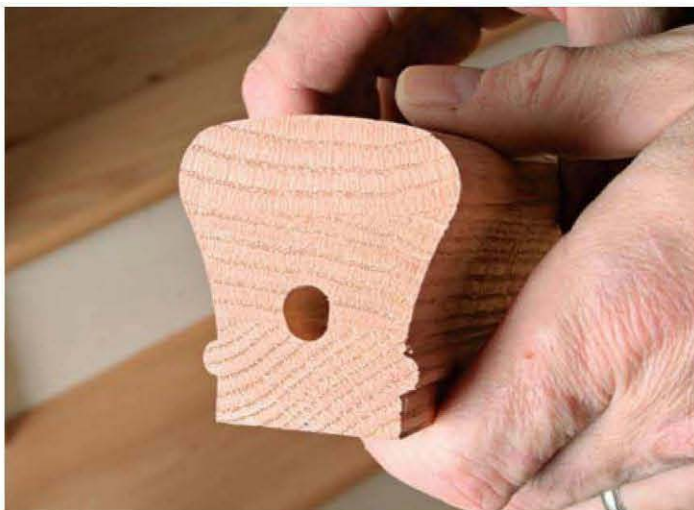
A reamed bolt hole allows proper alignment of railing parts. Using the 3/8-in. bit, drill out the side of the bolt hole that's opposite the direction the rail needs to move.
