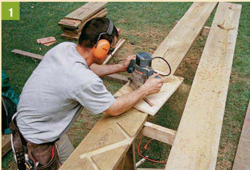
1 Use a plywood jig and a bearing-guided bit to rout mortises in a 2x10 stringer.
