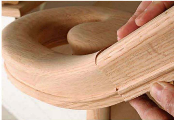
A misaligned rail and fitting is a sign of a misaligned bolt hole. Minor misalignments are to be expected, but this one is too much to fair out.
