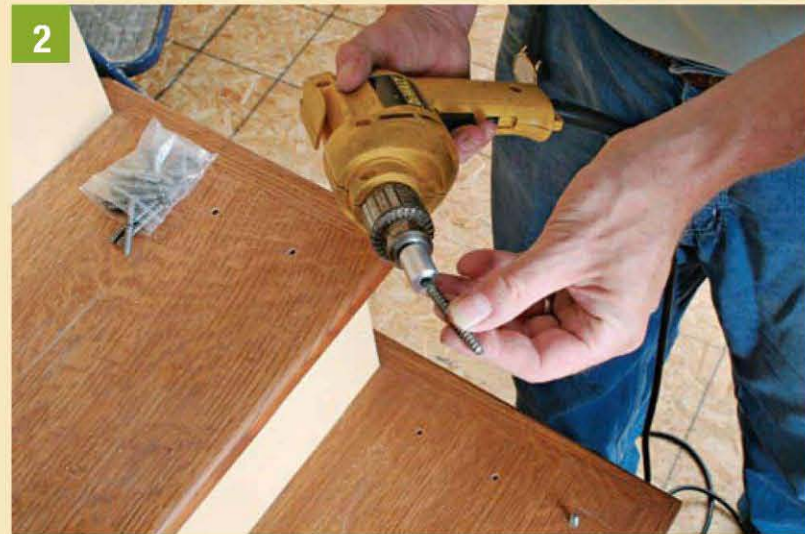
2 Thread an aluminum driver onto the lags.
