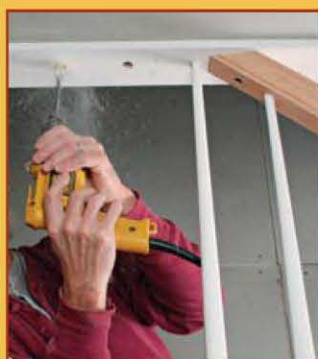
178 | Installing Balusters
