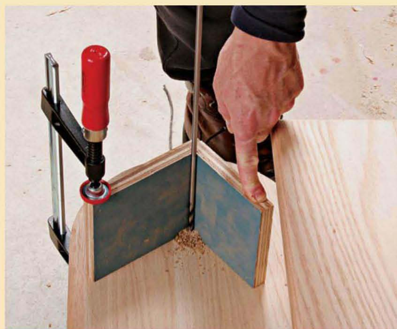
A plywood jig guides a pilot bit. Two pieces of plywood screwed square together and clamped to a level step keep a \frac{1}{4} -in. bellhanger’s bit plumb.
