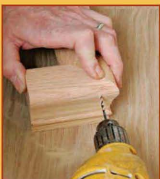
155 | Installing Wall Rails
