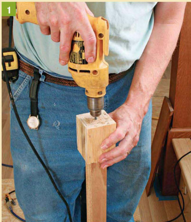
1 Use a plywood jig to center the drill to make pilot holes in the balusters.
