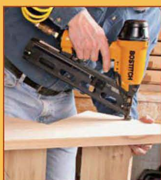
82 | Installing the Treads and Risers
