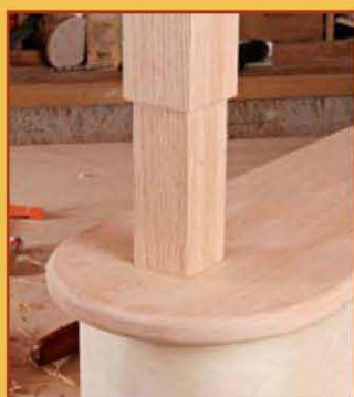
110 | Attaching the Bullnose
