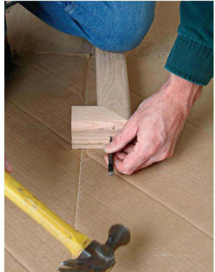
Work several nails at once to prevent the pieces from moving out of alignment. Start the nails into their pilot holes and hammer each one partially home before setting any of them. Five-minute epoxy ensures a long-lasting joint between the returns and the rail.
