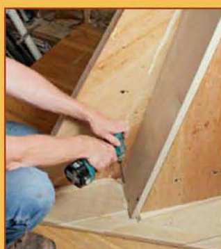
124 | Building the Stair
