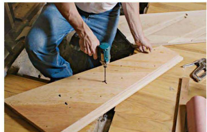
Screws make the connection. Attach the subthread from below using 1 1/2-in. pan-head cabinet screws. These screws should be roughly centered in the slots and set just enough to snug the subthread to the tread.
