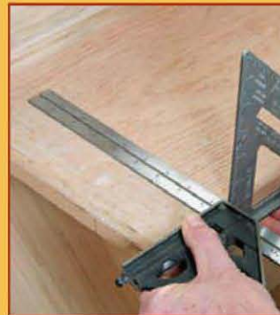
136 | Marking and Notching the Treads
