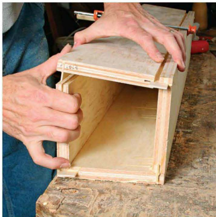
Glue and spline-join the plywood sides. Clamps and a few nails will hold the newel together until the glue sets.
