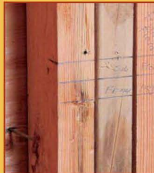
26 | Laying Out the Stair
