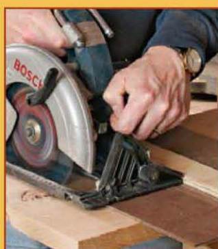
71 | Cutting the Treads and Risers
