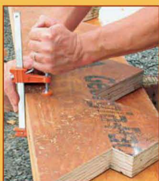
29 | Laying Out the Stringers
