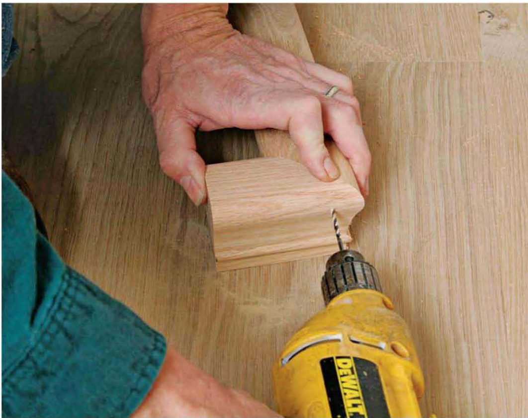
Pre-drill for finish nails. With the rail and the return seated on a flat surface, drill pilot holes. Go slow and hold the parts with your fingers so that the drill doesn't push them apart.
