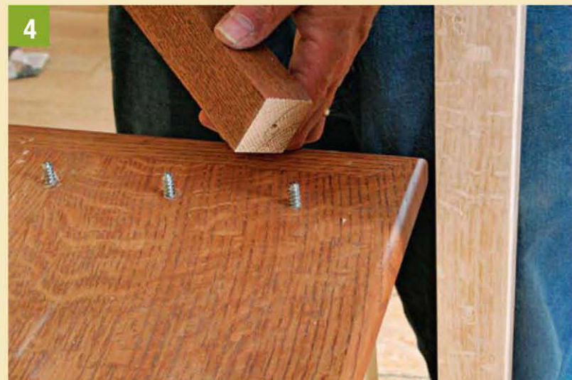
4 Thread the baluster onto the lag by hand.
