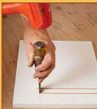
44 | Notching the Inner Skirtboard
