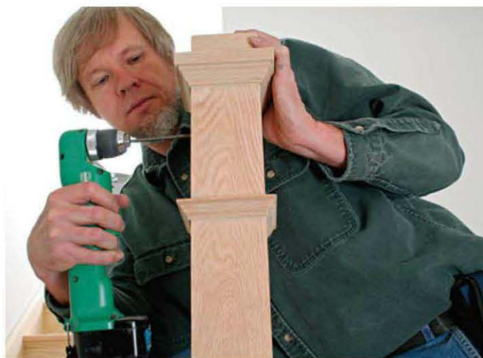
A bolt will affix the level rail to the newel. Drill a pilot hole partway through the newel. Complete the hole from the other side.
