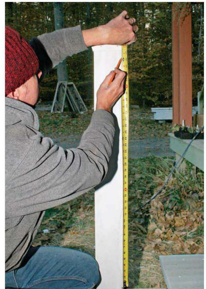
Mark the top of the rail on the newel. Measuring up the desired rail height from the pitch line positions the top of the rail.
