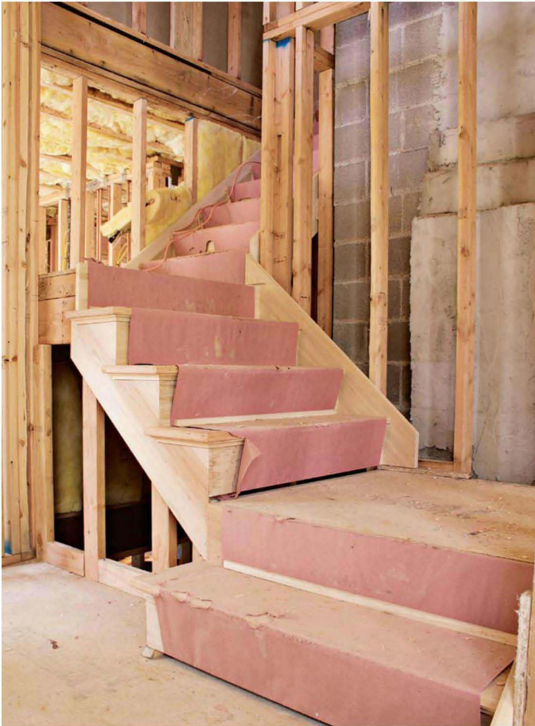
Combination stairs use both notched and housed stringers. The trick to these shop-built stairs, which are commonly used for main stairs, is knowing which assembly techniques to borrow from which type of stringer.
