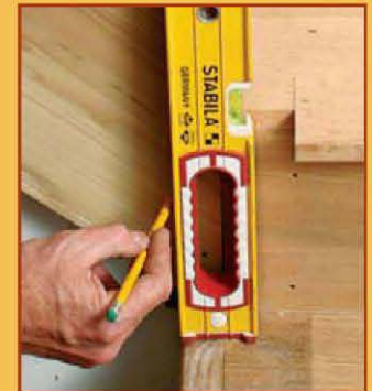
137 | Laying Out the Newel
