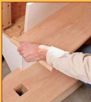
49 | Attaching the Treads and Risers
