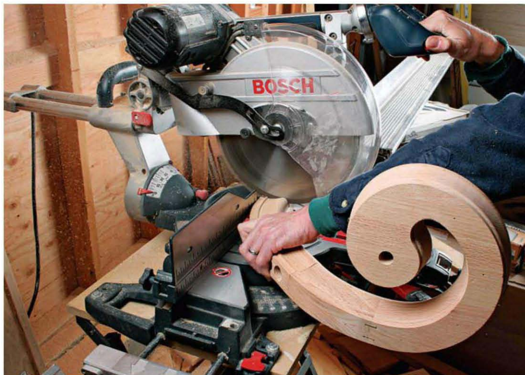
Firmly seat the easing on the saw table so that its entire edge has contact. The bottom of the easing makes a line of contact against the fence; cut slowly.
