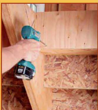
35 | Installing Treads and Risers
