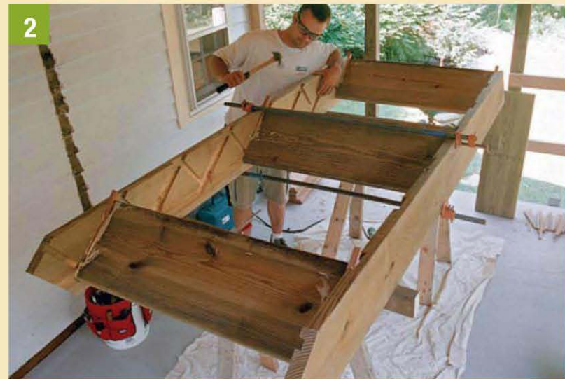
2 The first step in the assembly is to wedge the treads into the mortises.
