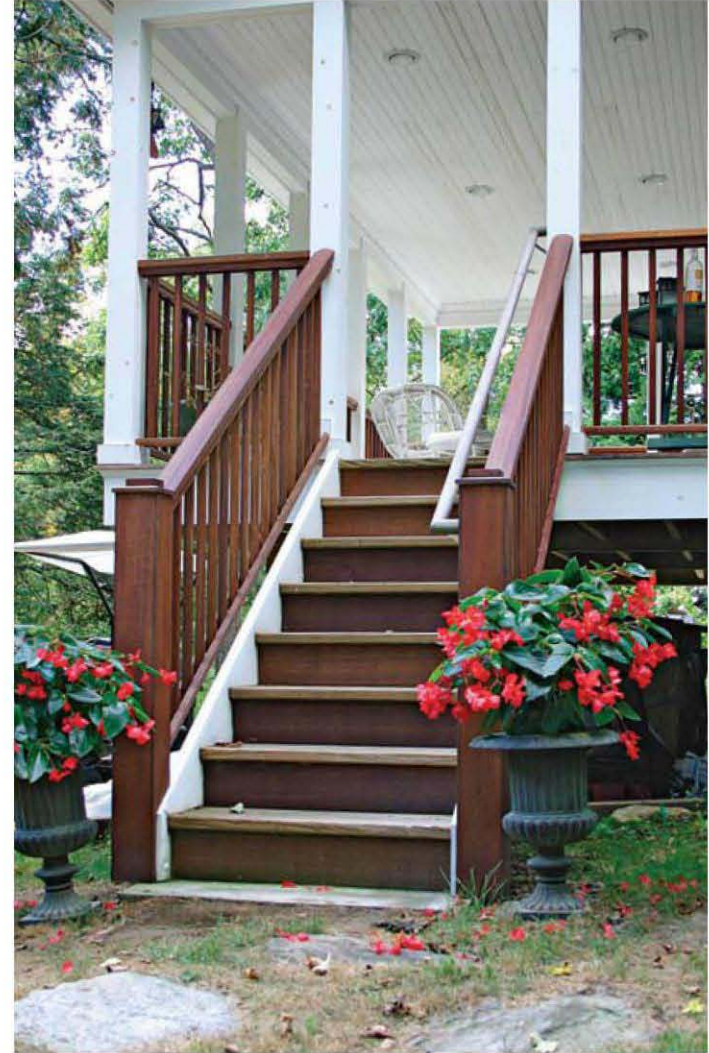
Housed-stringer stairs are a good choice for a large rise because of their overall superior strength.
