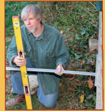
202 | Measuring for the Stair
