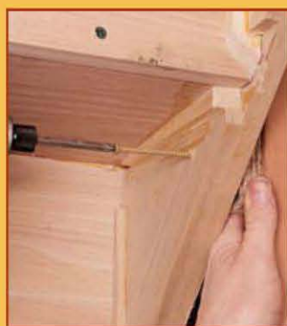
75 | Installing the Stair
