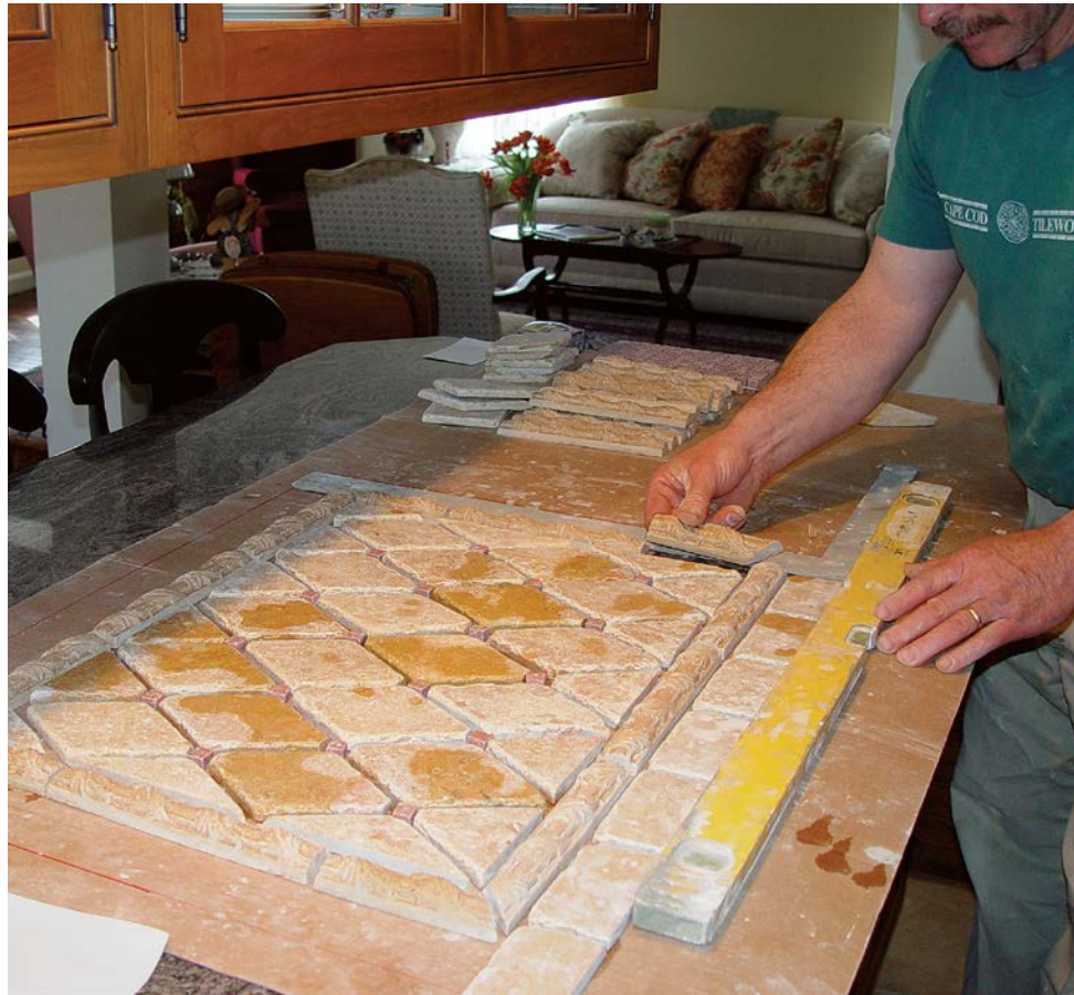
TEST-FIT THE TILES ON A FLAT SURFACE. For the area above the stove, the author first measures the exact dimensions (top left photo). Decorative elements such as the border and the square accent tiles are cut and fit (bottom left photo). Then he transfers them to a sheet of cardboard, where all the tile is dry-fit (right photo).
