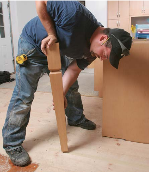
ATTACH THE LEGS TO THE FLOOR. After drilling a hole in the center of the leg, fasten the leg to a 2½-in. drywall screw that's been cut off with lineman's pliers (left). This anchors the leg in place without visible fasteners (below).
