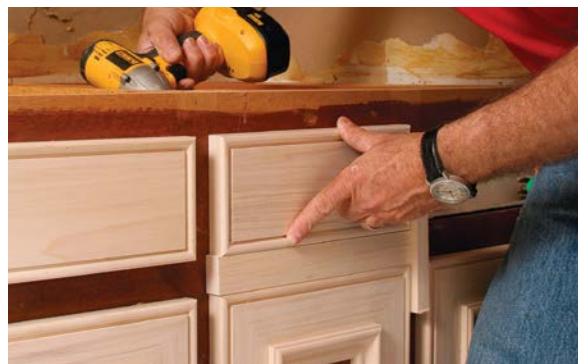
USING A SPACER JIG to establish a consistent height above the cabinet doors, secure each drawer front from the inside of the drawer box with screws.
