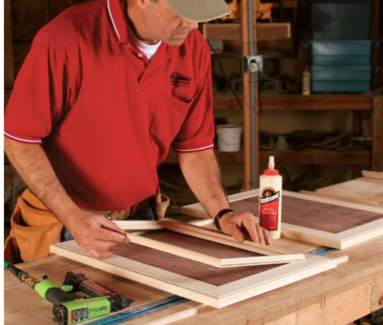
THE PANEL MOLDING , which also gets a shallow rabbet before assembly, is used to secure the panel in place and hide the joint.
