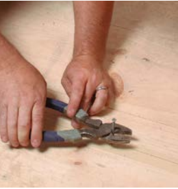
ATTACH THE LEGS TO THE FLOOR. After drilling a hole in the center of the leg, fasten the leg to a 2½-in. drywall screw that's been cut off with lineman's pliers (left). This anchors the leg in place without visible fasteners (below).
