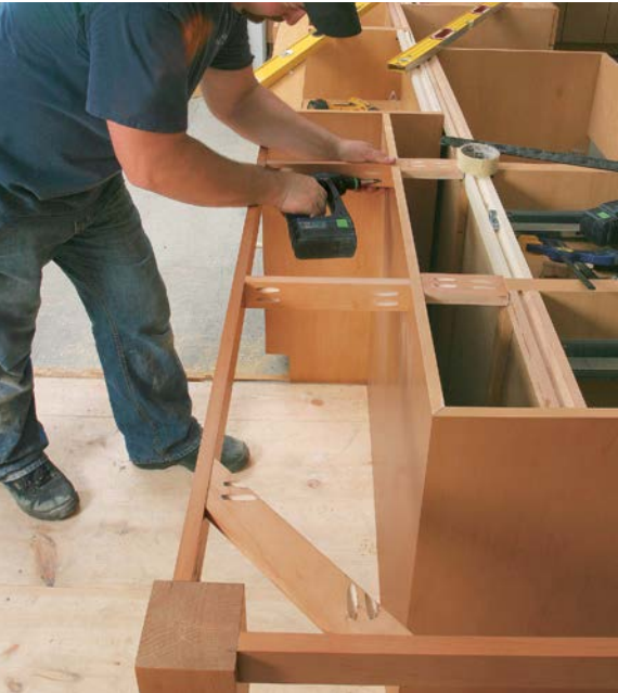
INSTALL AN APRON. Secured with pocket screws, a 2-in.-wide apron under the overhanging countertop supports the legs and provides a finished look. A 6-in. apron on the back of the island holds a receptacle.
