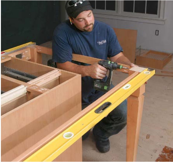
INSTALL AN APRON. Secured with pocket screws, a 2-in.-wide apron under the overhanging countertop supports the legs and provides a finished look. A 6-in. apron on the back of the island holds a receptacle.
