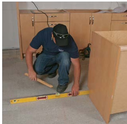
FIND MIDDLE GROUND. Many installers find the highest point of the floor to reference cabinet height, and then shim up the cabinets that sit on low spots. A better option is to find a cabinet at average height and then shim the low cabinets up and plane the high cabinets down. Shimming and planing should be minimal.
