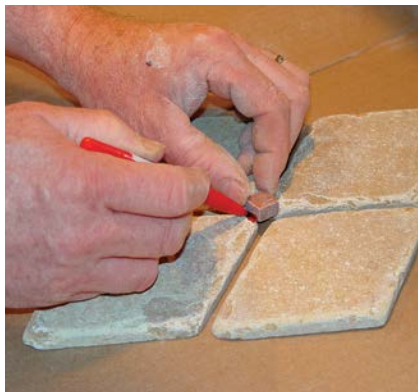
TEST-FIT THE TILES ON A FLAT SURFACE. For the area above the stove, the author first measures the exact dimensions (top left photo). Decorative elements such as the border and the square accent tiles are cut and fit (bottom left photo). Then he transfers them to a sheet of cardboard, where all the tile is dry-fit (right photo).
