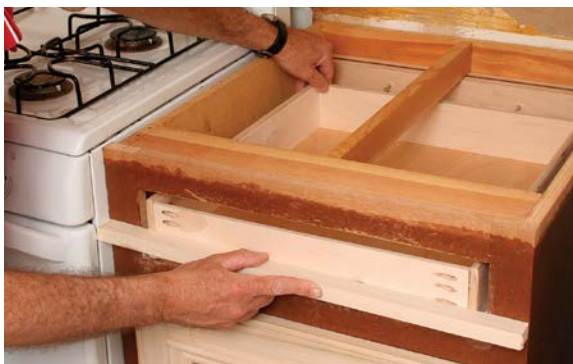
SLIDE THE DRAWER BOX INTO PLACE , and use a straightedge to adjust the slides until the drawer box is flush with the face frame. Then drive the screws to secure the assembly.
