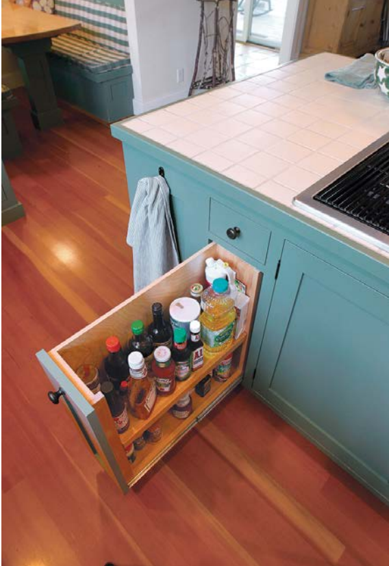
NO LOST CONDIMENTS. A pull out drawer on full-extension slides means your ketchup won't languish in the back of a cabinet.
