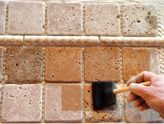
SEAL. GROUT. SEAL AGAIN. Stone tile should be sealed before grouting to prevent the grout from sticking to it (above). After grout is applied (right) and becomes firm, remove the excess with a sponge and dry cloth.
