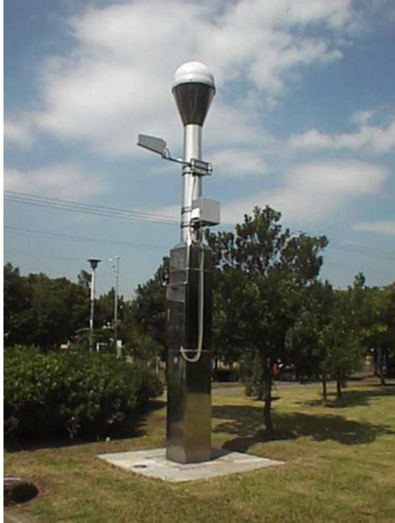
Fig. 9.12 A GEONET GNSS-based CORS station in Japan. Source Geospatial Information Authority of Japan
