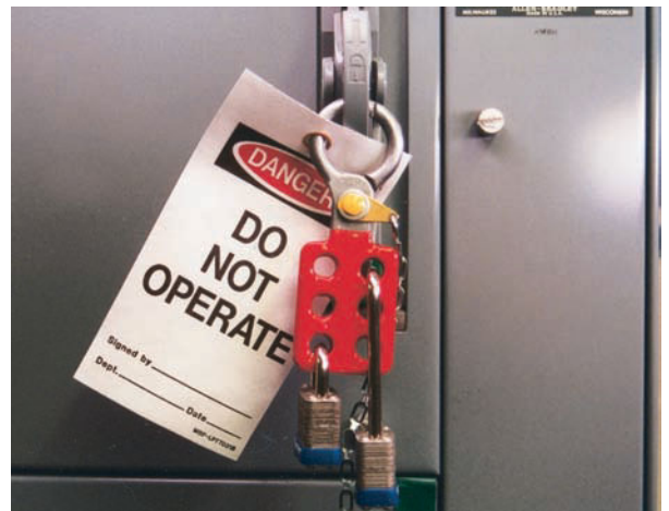
FIGURE S-5 The equipment can be locked out by several different people.
