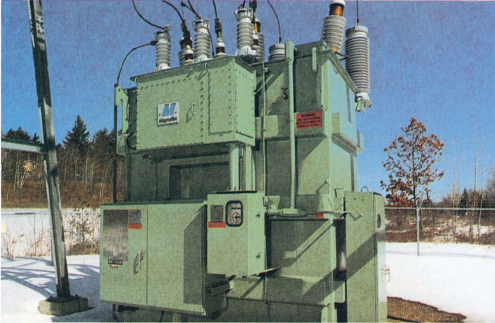
FIGURE 28-43 Three-phase autotransformer. (Courtesy of Waukesha Electric Systems)
