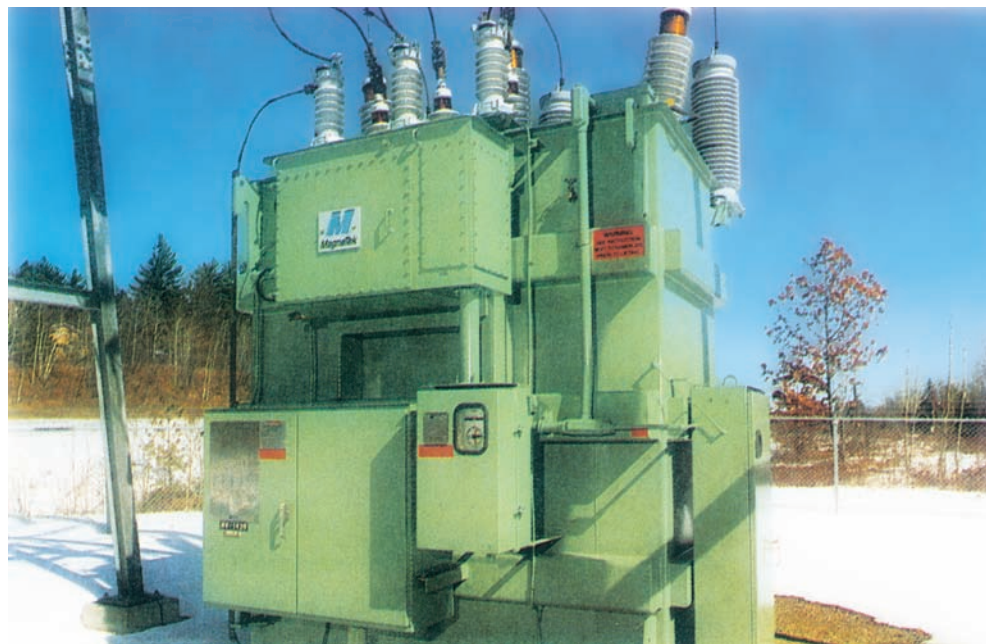
FIGURE 28–43 Three-phase autotransformer.
