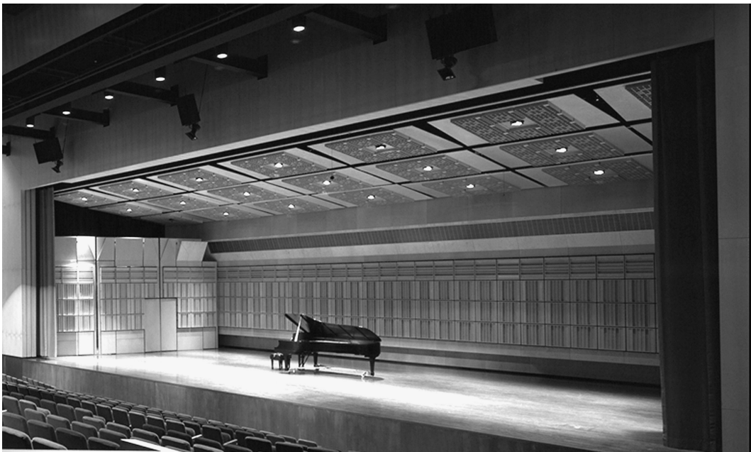
Figure 3.34 Diffusers around the stage of the Corning Glass Center, NY. (Copyright Paul Warchol Photography, http://www.warcholphotography.com .)
