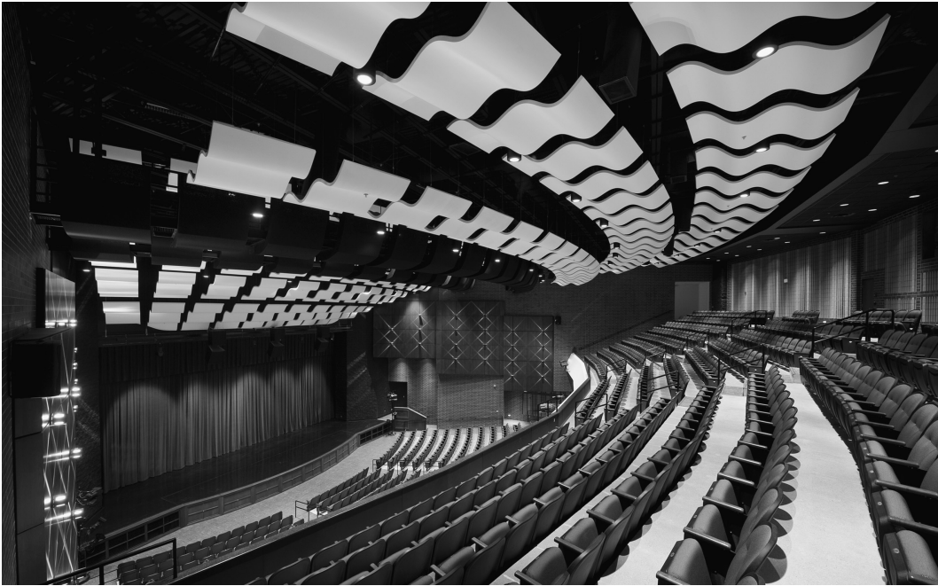
Figure 3.40 Optimized curved audience canopy (Waveform Spline) in Northridge High School, Middlebury, IN. Architect: Moake Park Group, Inc. Acoustician: dBA Acoustics. (Courtesy of dBA Acoustics.)
