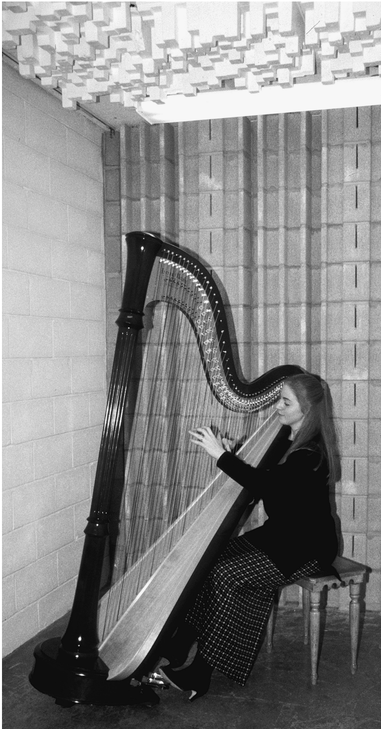
Figure 3.19 A music practice room treated with diffusers (Skyline® on the ceiling 20 and DiffusorBlox® on rear wall 21 ) and absorbers. (Courtesy of D'Antonio, P., Cox, T.J., Appl. Acoust. , 60, 113–142, 2000.)
