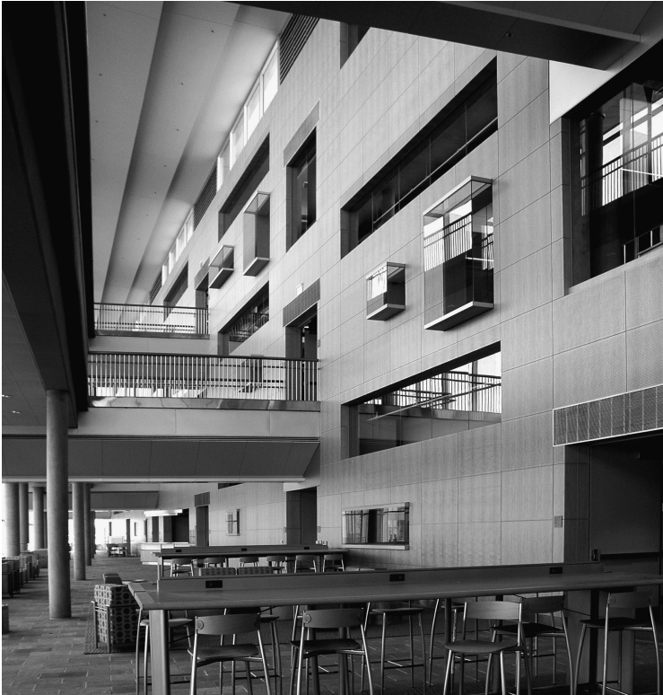
Figure 2.2 Perforated, absorptive wood panelling covering the entire feature wall opposite an exterior glass wall (out of shot) in Morgan State University in Baltimore, MD. Acousticians: Shen, Milsom, and Wilke, Ballston, VA. (Courtesy of RPG Diffusor Systems, Inc.)
