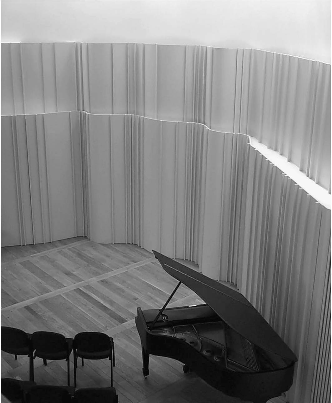
Figure 3.39 Optimized curved surface (Waveform) in the Edwina Palmer Hall. Acoustician: Raf Orłowski. (Courtesy of Arup Acoustics.)
