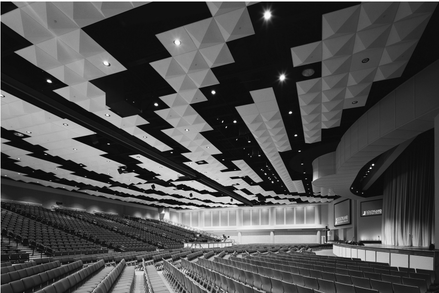
Figure 11.19 Pyramid ceiling treatment at Southland Christian Church, Nicholasville, KY, Acoustician: Michael Garrison Associates. (Courtesy of Michael Garrison Associates.)
