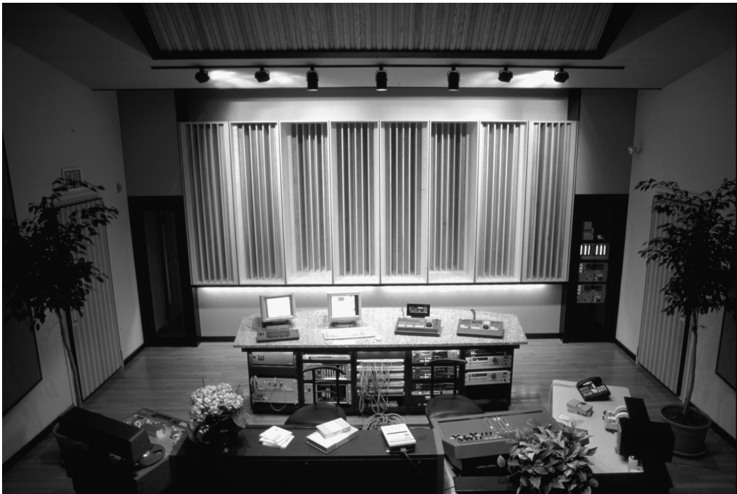
Figure 3.12 Gateway Mastering, Portland, ME, showing a fractal diffusing rear wall (DiffRACTAL®). (Courtesy of Gateway Mastering + DVD.)
