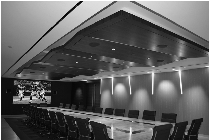
Figure 2.3 Custom microperforated (Perfecto®) angled ceiling cloud at the NFL Conference Room, New York. (Courtesy of RPG Diffusor Systems, Inc.)
