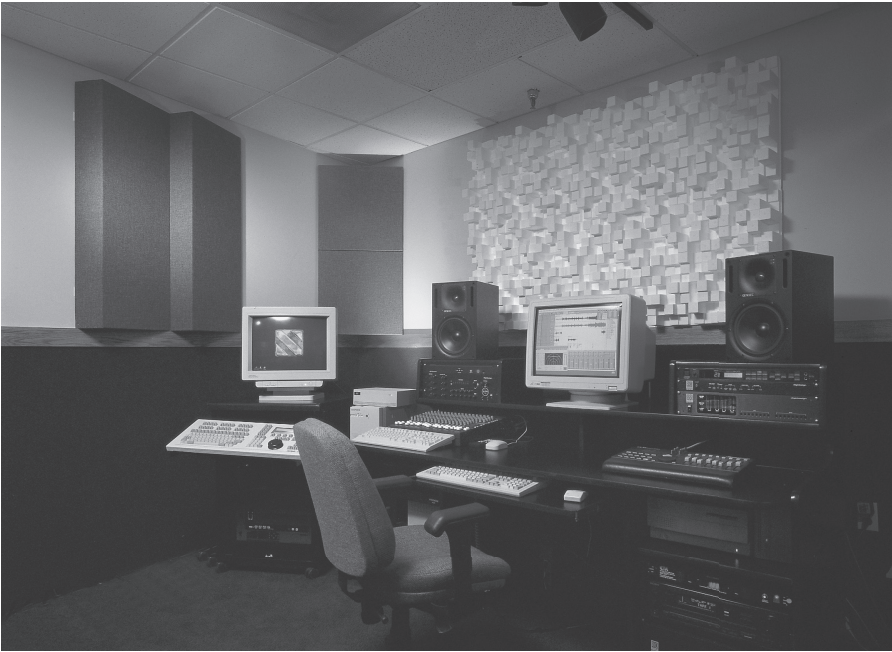
Figure 7.3 (a) — Measured and — predicted normal incidence absorption coefficient for a commercial membrane absorber (Modex™). (b) A typical installation in a small reproduction room; the resonant absorber is in the corner of the room. (Courtesy of RPG Diffusor Systems, Inc.)
