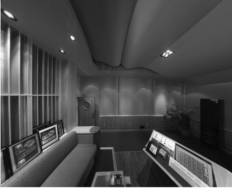
Figure 12.3 A curved hybrid diffuser applied to the ceiling and side walls of SonyMI, New York. Acoustician: Harris Grant Associates. (Courtesy of Paul Ellis of The M Network Ltd.)
