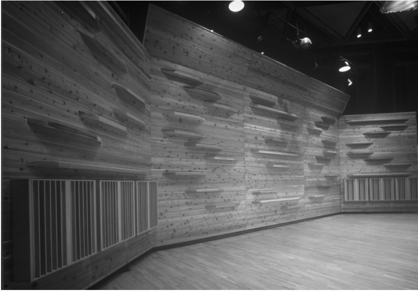
Figure 11.15 The upstage wall at Nicholas Music Center, Rutgers University, showing an array of protruding shelves to provide corner cube reflections back to the musicians for support. (Courtesy of RPG Diffusor Systems, Inc.)
