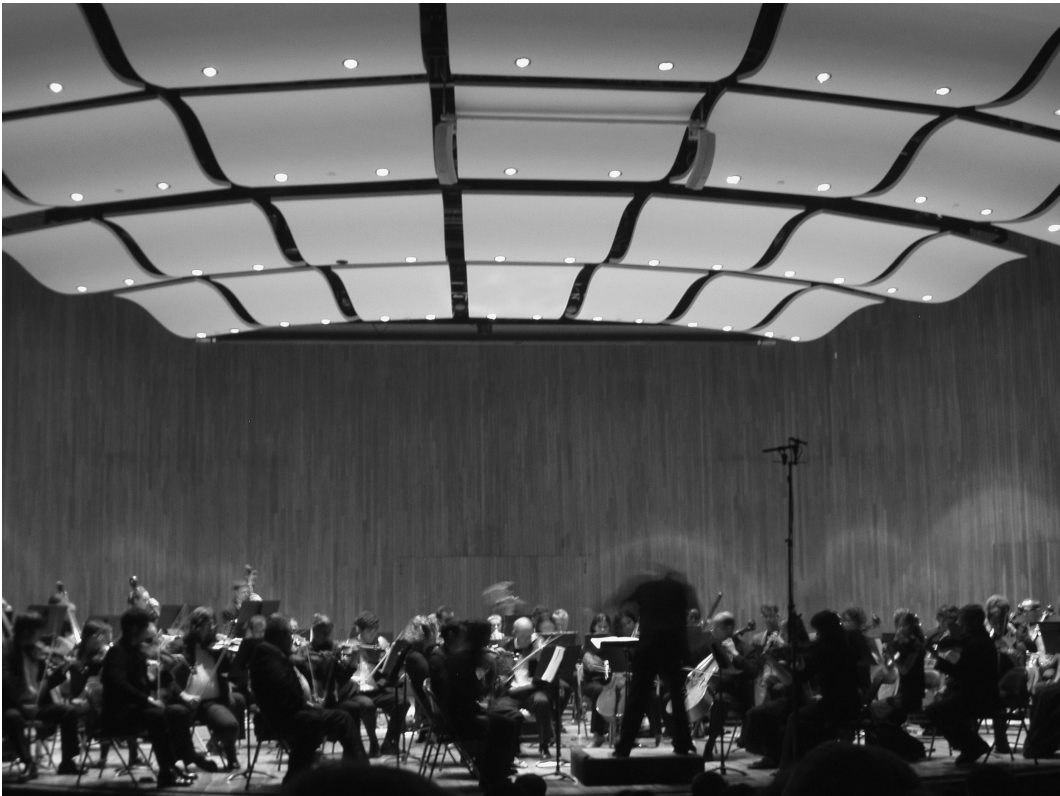
Figure 3.27 Overhead stage canopy (Waveform) at Kresge Auditorium, Boston, MA. Acoustician: Rein Pirn, Acentech, Boston. (Courtesy of Daderot, commons.wikimedia.org/wiki/File:Kresge_Auditorium,_MIT_(interior_with_concert).JPG.)
