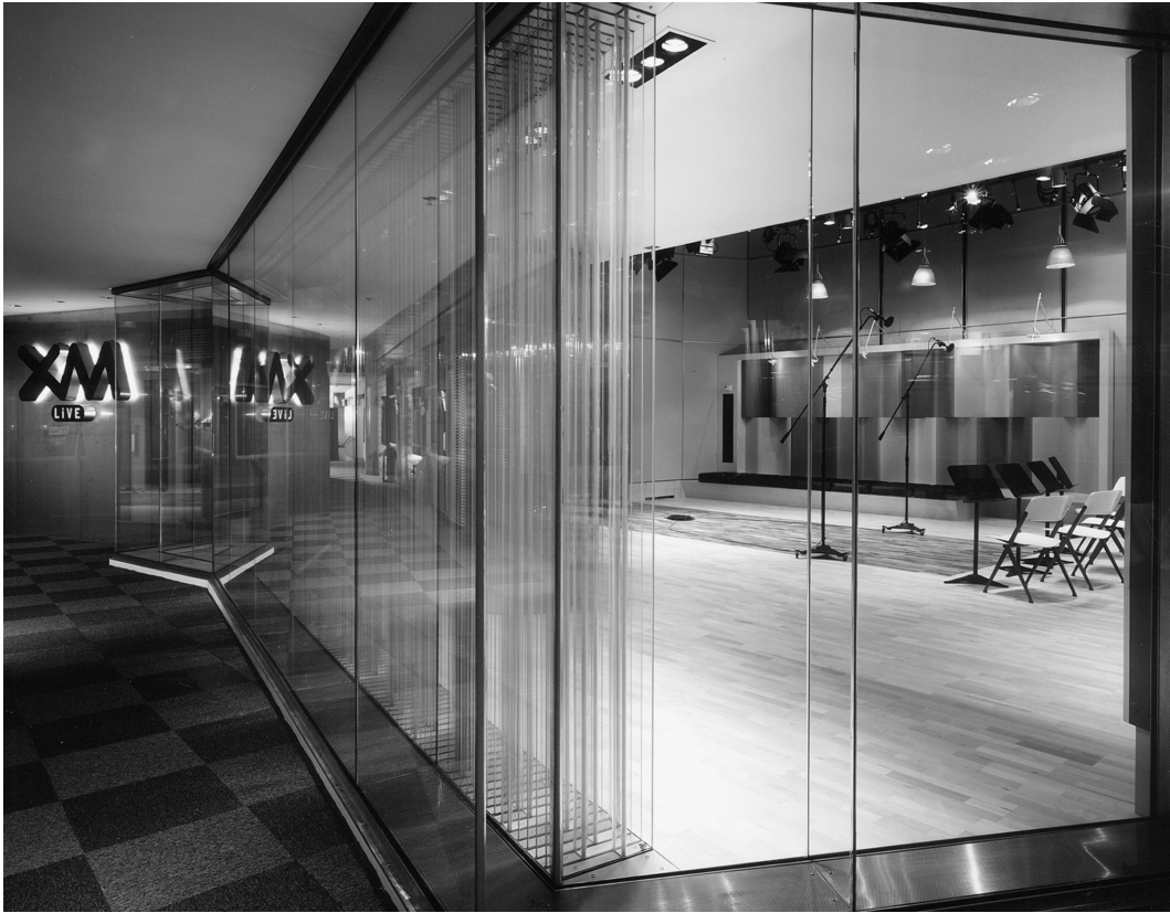
Figure 3.18 A live performance studio seen through a glass Schroeder diffuser. The opposite wall features Waveform® Spline, an optimized curved diffuser. XM Satellite Radio, Washington, DC. Acoustician: Francis Daniel Consulting Alliance. (Courtesy of Michael Moran Photography.)
