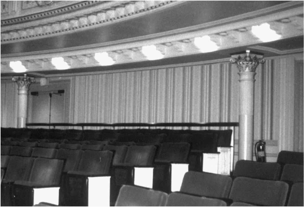
Figure 3.1 Schroeder diffusers (QRDs) applied to the rear wall of Carnegie Hall to prevent echoes. (Courtesy of D'Antonio, P., Cox, T.J., J. Audio Eng. Soc. , 46, 955–976, 1998.)
