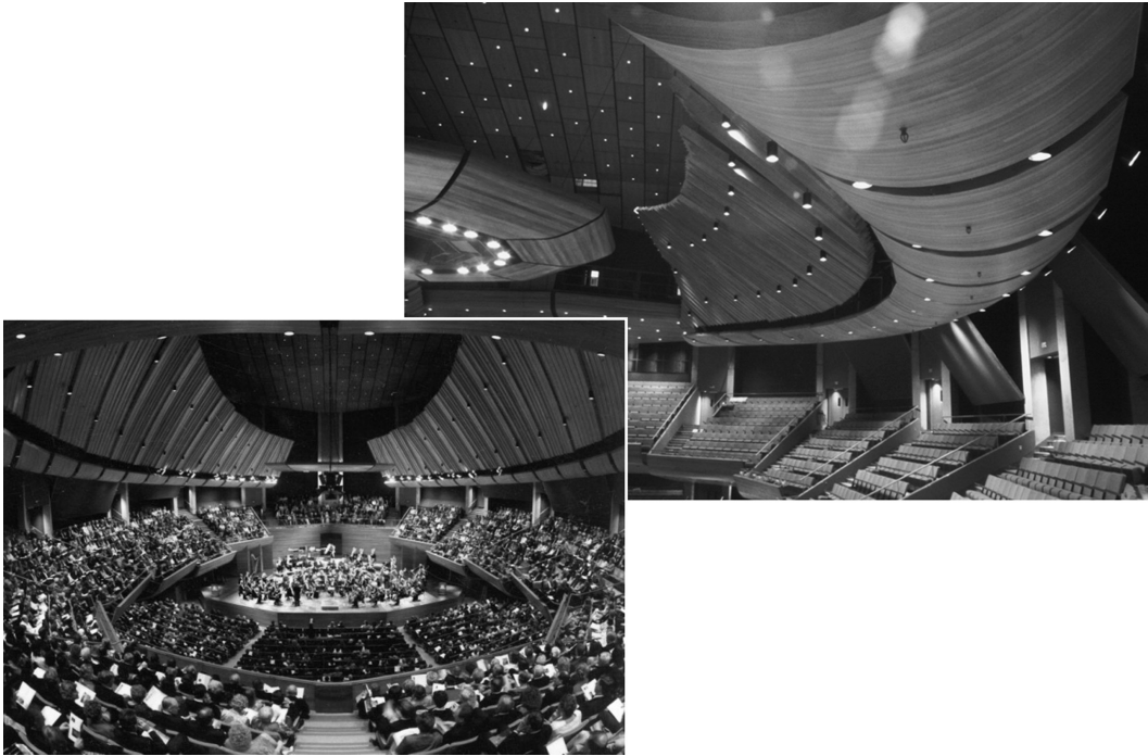
Figure 3.25 Schroeder diffusers in the Michael Fowler Centre, New Zealand. (Courtesy of Dr. Harold Marshall of Marshall Day Acoustics.)
