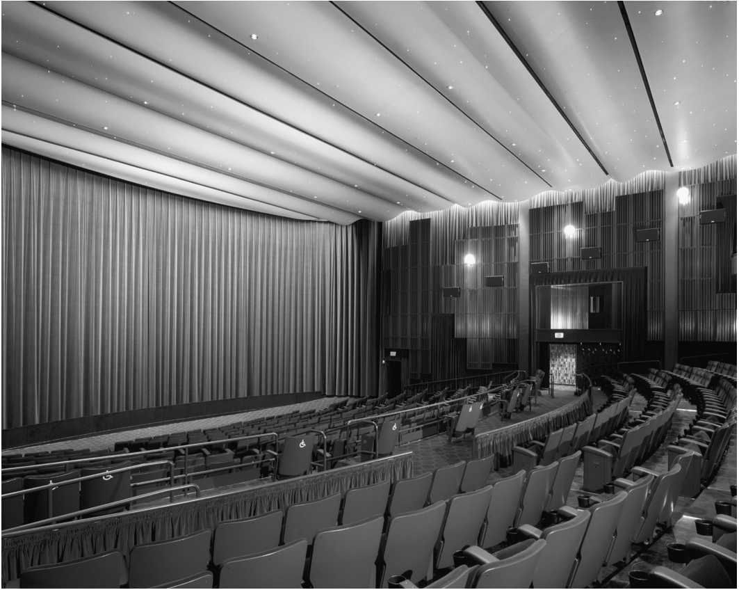
Figure 3.26 Cinerama Theatre, Seattle, WA, with a diffusing ceiling (OptiCurve). (Courtesy of University of Salford.)
