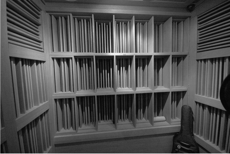
Figure 12.5 A hybrid diffuser made from slats in front of porous absorbent as applied in a recording room. (Courtesy of Bogić Petrović and Zorica Davidović.)
