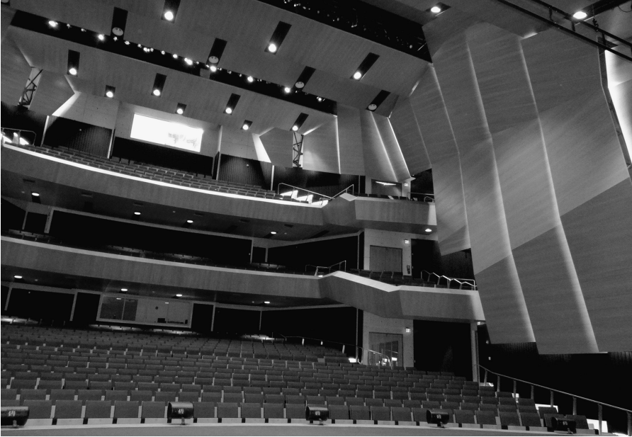
Figure 11.8 Angled side wall panels at Centro de Bellas Artes Humacao, Puerto Rico, Acoustician: Jorge Rocaforte Consulting. (Courtesy of Jorge Rocaforte Consulting.)
