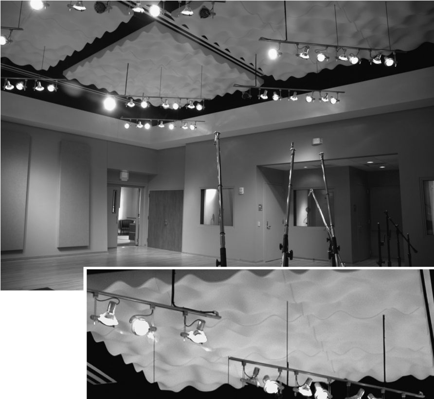
Figure 11.41 Modulated curved diffusers used in the ceiling of a radio production studio at KTSU, Texas Southern University, Houston, TX. Acoustician: HFP Acoustical Consultants. Insert shows close-up of ceiling.
