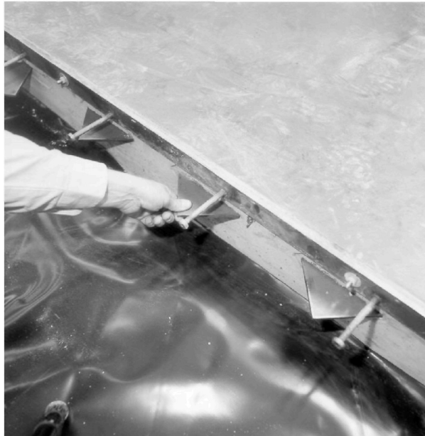
Figure 2 Detail of a day or construction joint with armoured steel aris to protect against degradation caused by wheeled handling equipment
