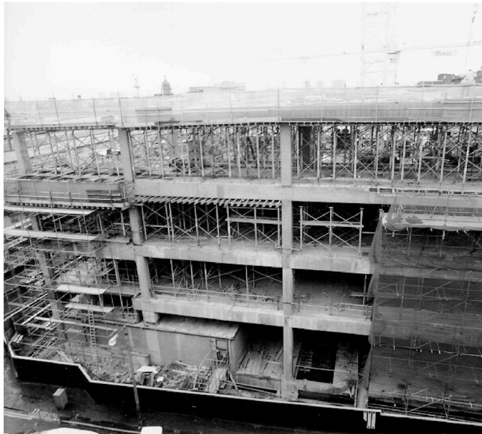
Figure 4 Table form falsework system for fast construction process
