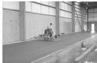
Figure2 Ride on power trowel, long strip
