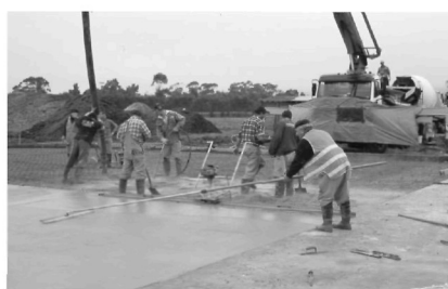
Figure 12 Power float & scraping straight edge
