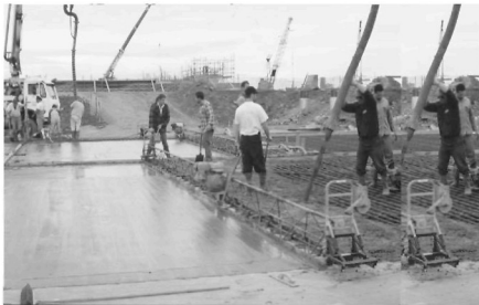
Figure 3 Removable rails, double width strip Figure 4 Initial trowelling with panfloats
