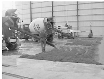
Figure 6 Direct concrete placement
