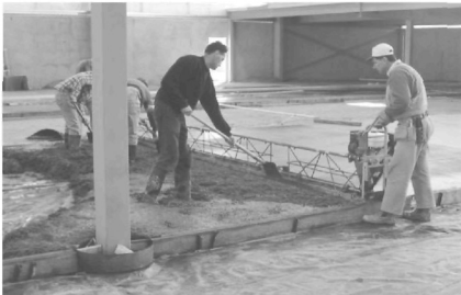
Figure1 Truss vibrating screed, FRC slab
