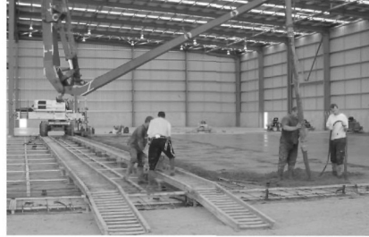
Figure 10 Ladder tracks & concrete pump
