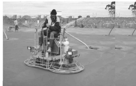
Figure 3 Removable rails, double width strip Figure 4 Initial trowelling with panfloats
