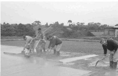
Figure 11 Power float with spot levels
