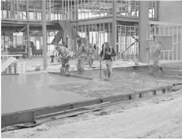
Figure 7 Power float, long strip pour Figure 8 Walk behind helicopter power trowels
