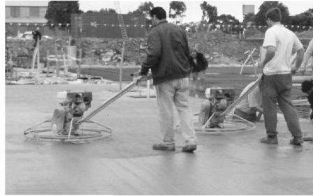
Figure 7 Power float, long strip pour Figure 8 Walk behind helicopter power trowels
