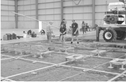
Figure 9 Laser screed on post-tensioned slab
