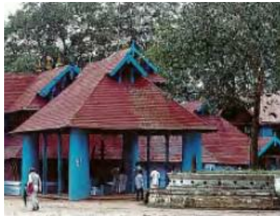
A temple in Trichur, Kerala. Composed of several individual buildings, including the main shrine, the roofs are covered with sloping tiers of terracotta tiles typical of the overhanging Kerala roof, sometimes broken by projecting eaves.
