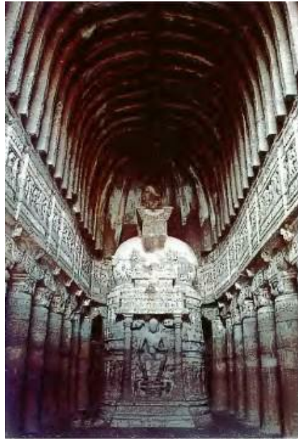
The interior of a chaitya hall at Ajanta, early 8th century AD, with its carved stone imitation of a wooden barrel vault.
