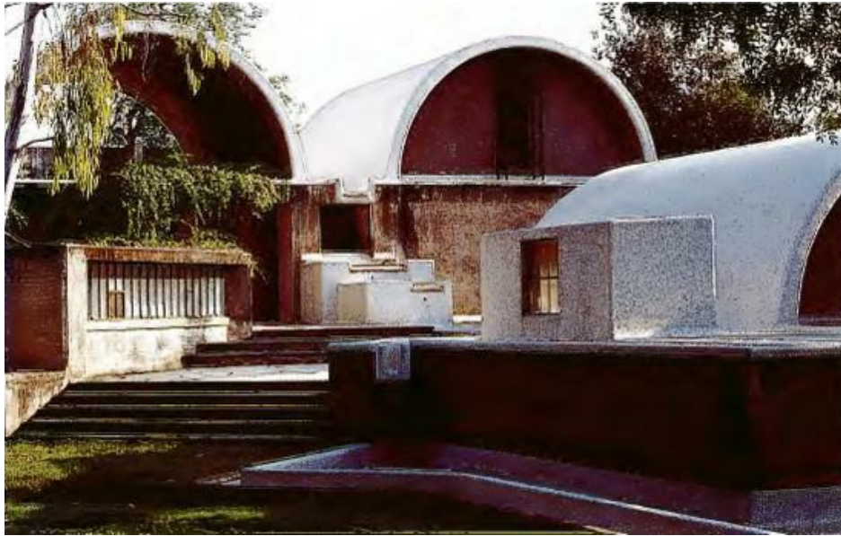
Balkrishna Doshi's own office and research center at Sangath, Ahmedabad, uses earth forms, open terraces and water channels to create an environment that is suitable to both the local climate and ethos.
