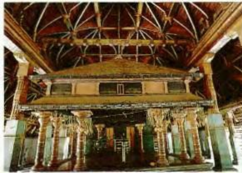
The interior of a kuttambalam , with its wooden ceiling specially designed for good acoustics. The hall is surrounded by wooden pillars and jaalis on three sides to provide ventilation.
