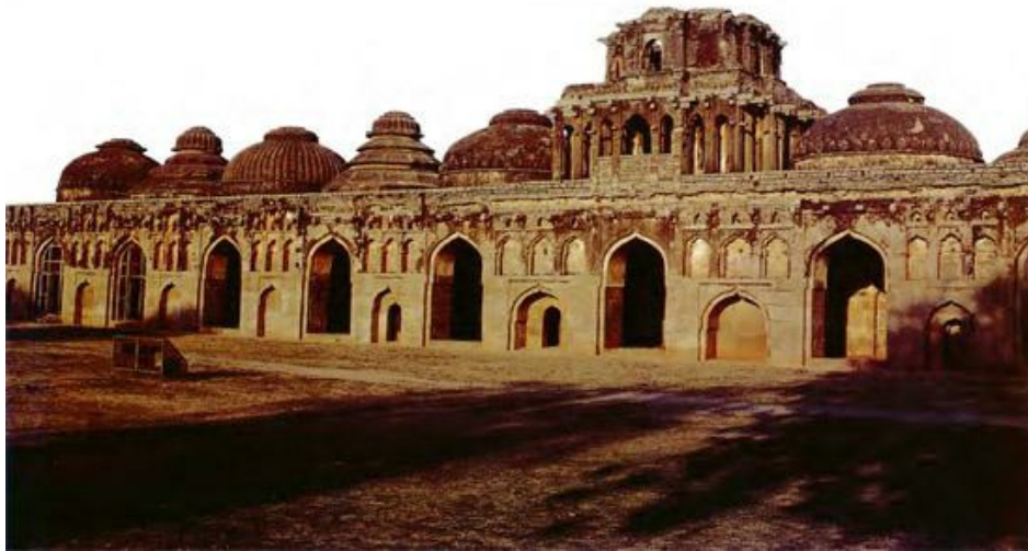
Elephant Stables, Hampi. The elevation displays distinctly Islamic features, such as curved openings, recessed lobed arches and domes. An overhanging eave and parapet surmounts the walls. The tower rising above the upper chamber has now collapsed.
