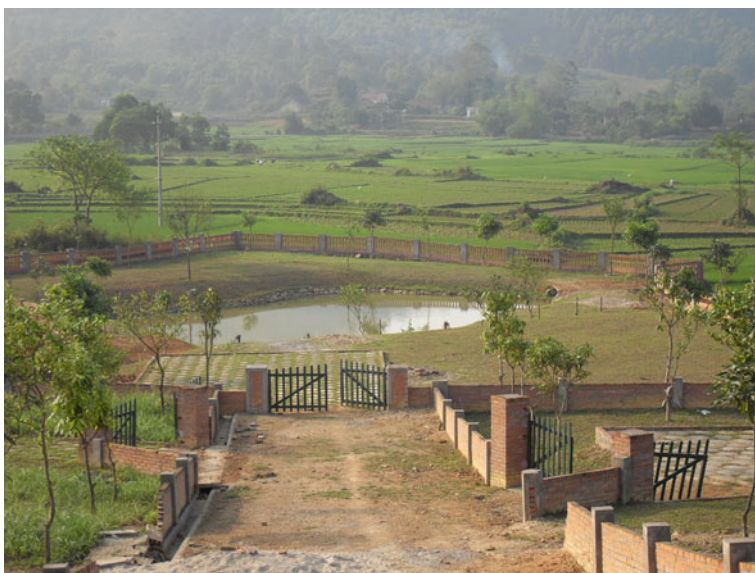
Fig. 9.1 A plot of land ready for construction of a villa
