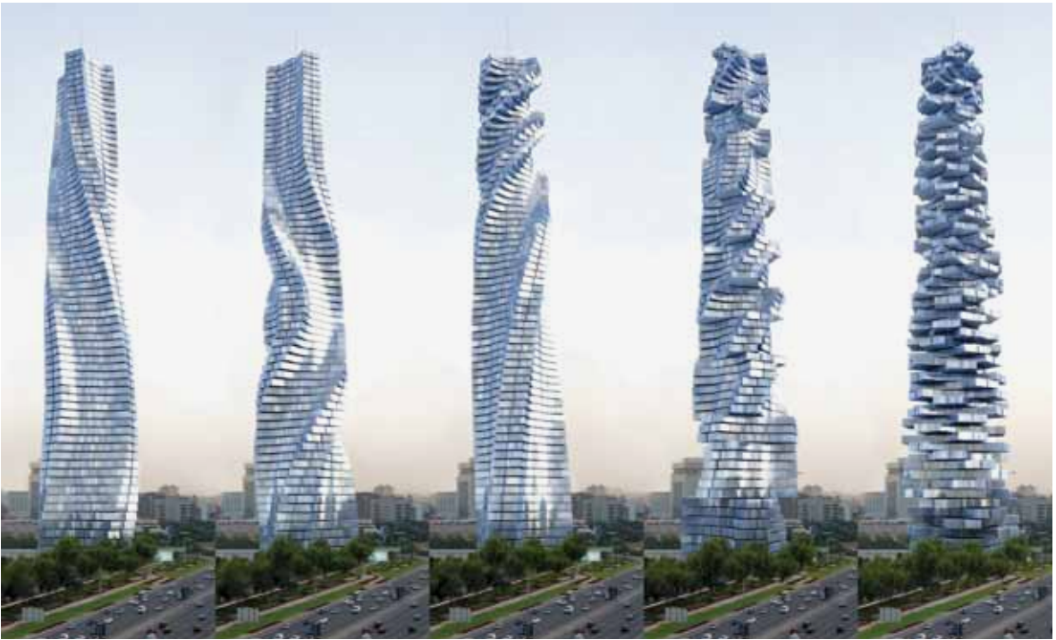
The Dynamic Tower concept by Dr. David Fisher is an example of incorporating high-tech solutions in a visible way. Each floor rotates separately, powered by wind turbines between the floors. The design also envisions that the building be entirely prefabricated, enabling rapid assembly.
