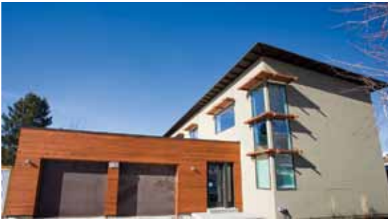
The Breezeway House (2009) in Utah, designed by Brach Design Architecture, is a certified Passive House.
