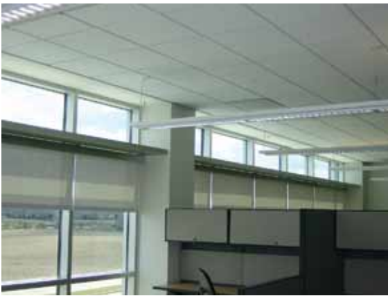
The light shelf placed at the upper portion of the windows reflects daylight up to the ceiling, providing illumination deep into the space.
