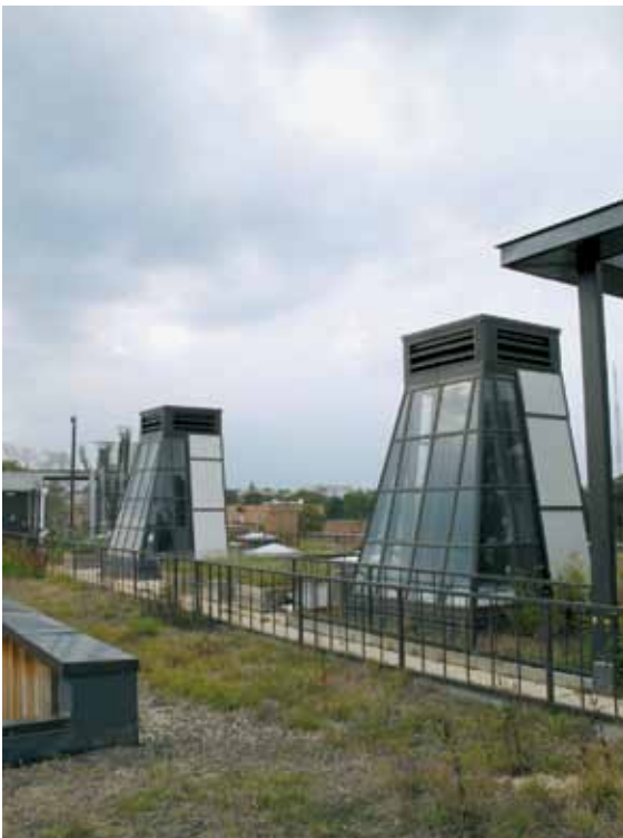
Solar chimneys at the Sidwell Friends School. Note the extensive green roof surrounding the chimneys.
