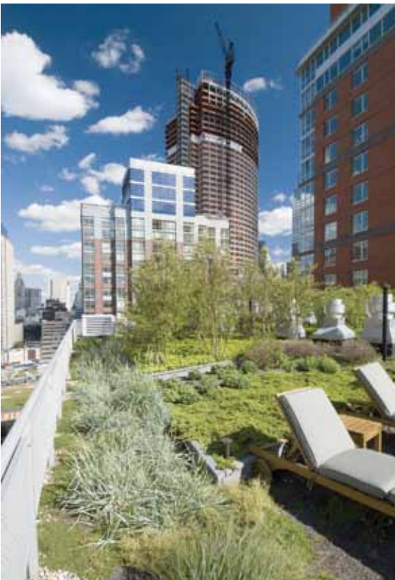
Extensive green roofs (top) have shallow rooted plants and weigh less than intensive green roofs.
