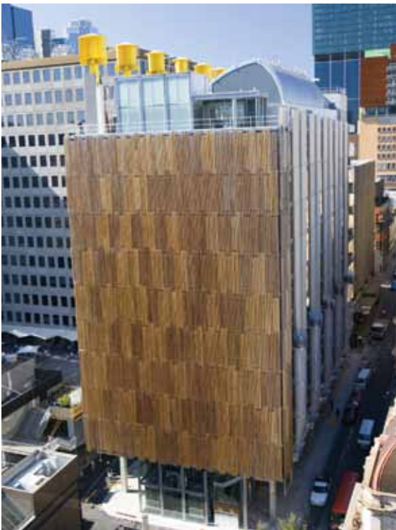
Council House 2 (2006) in Melbourne, Australia, designed by Mick Pearce, employs a ventilation system derived from the termite mound concept.
