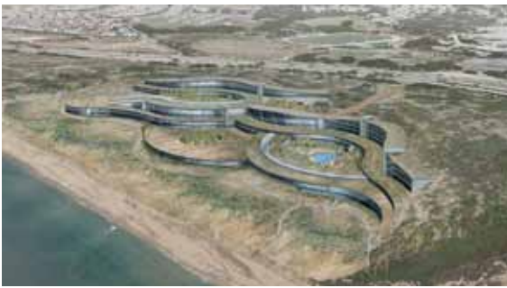
The proposed Monterey Bay Shores Ecoresort, designed by Bull Stockwell Allen, combines earth-bermed design with many other ecodesign principles, such as green roofs and regenerative use of brownfields.
