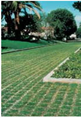
Impervious areas can be replaced with permeable materials and landscaping. This driveway has pervious pavers with grass growing in them.
