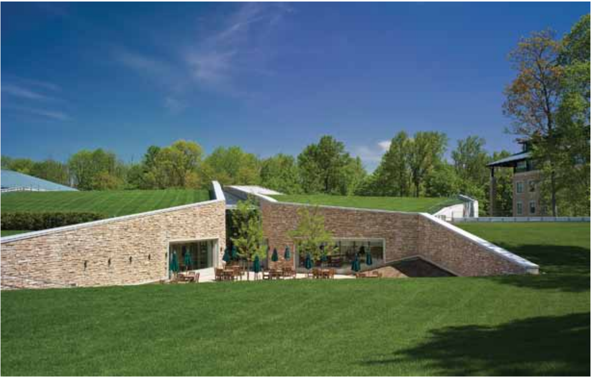
The semi-underground Becton Dickinson Campus Center (2008), designed by RMJM, incorporates thermal mass and vegetated roofing.
