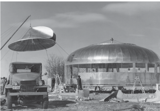
Prefabricated construction has been through several cycles of popularity and economic success: a Sears home (top) and Buckminster Fuller's Wichita House (1946).
