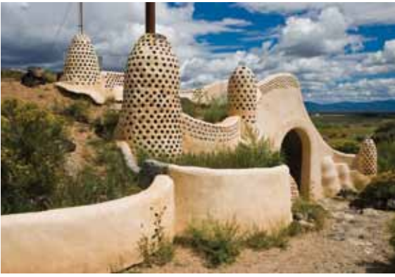
Earthships, passive solar homes made from natural and recycled materials, are an example of early visible green design.
