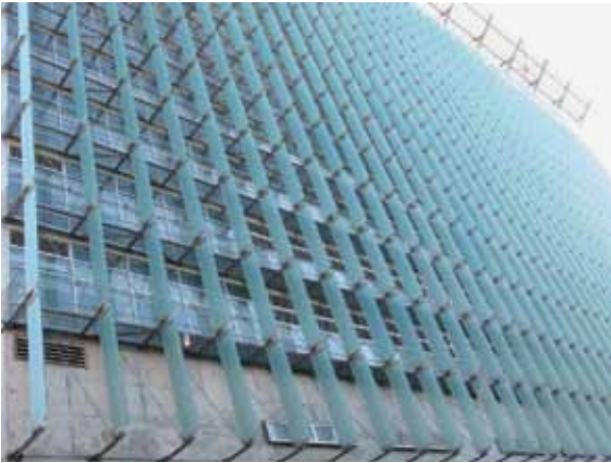
The north and south facades of the San Francisco Federal Building (2007), designed by Morphosis, have distinct designs in response to the differing solar conditions of the two sides.
