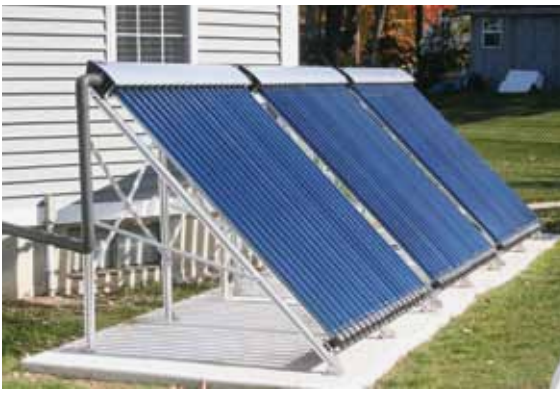
Solar thermal panels may have exposed collection tubes like this or may have the tubes behind a clear covering.
