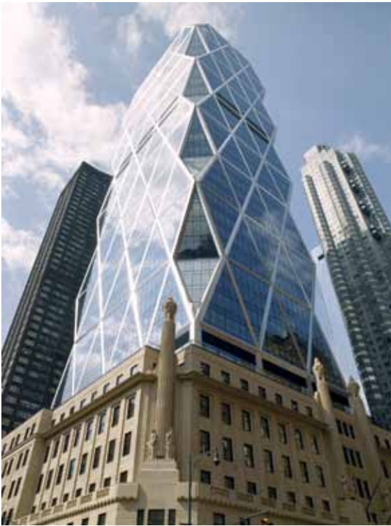
The unusual form of the Hearst Tower (2006), designed by Foster + Partners, uses 20 percent less steel than a conventional steel tower.
