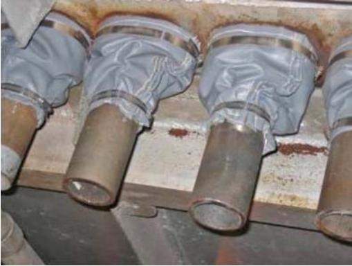
Figure 9.9. Radiant floor penetration and sealing. (Courtesy Thorpe Specialty Services Corporation; Houston, Texas. Used with Permission.)
