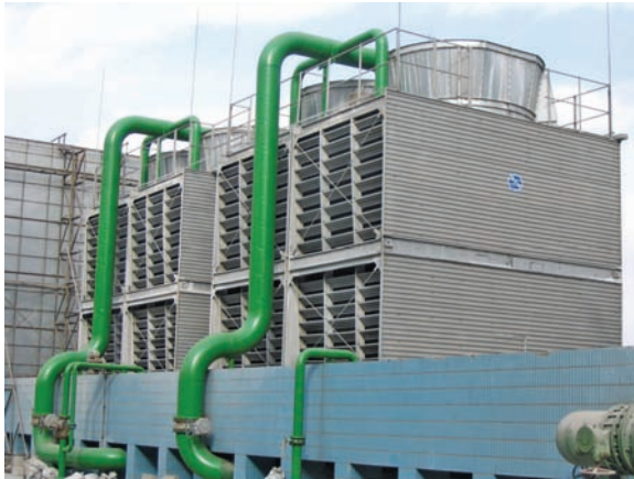
Figure 21.6. VR stacks installed on cooling towers increase airflow for the same energy input. (Courtesy Baltimore Aircoil Company. All rights reserved.)
