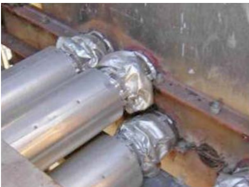
Figure 9.7. Convection tube penetration and sealing. (Courtesy Thorpe Specialty Services Corporation, Houston, Texas. Used with Permission.)
