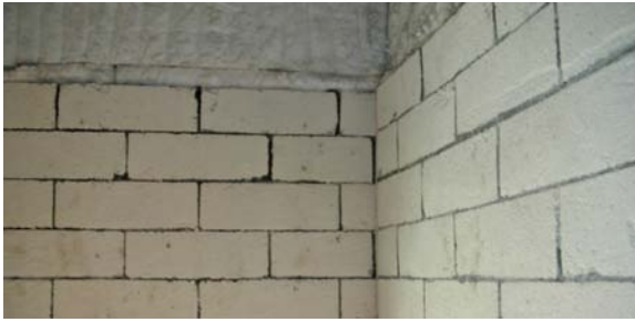
Figure 9.5. Lower wall of firebox with firebrick with ceramic fiber in the upper section. (Courtesy Thorpe Specialty Services Corporation, Houston, Texas. Used with Permission.)
