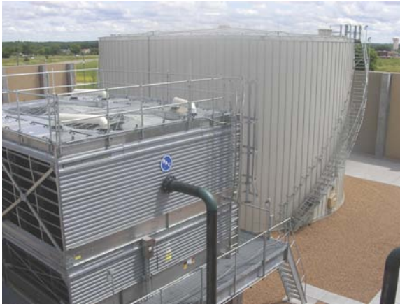
Figure 21.1. Induced draft cross-flow cooling tower. (Courtesy Baltimore Aircoil Company. All rights reserved.)
