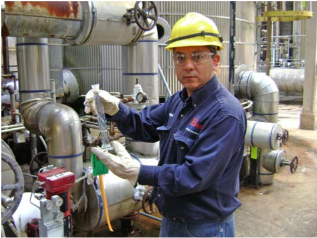
Figure 16.2. Octavio Torres, Energy Solutions Group Leader, measures condensation from iced-up surfaces in a chemical plant.
