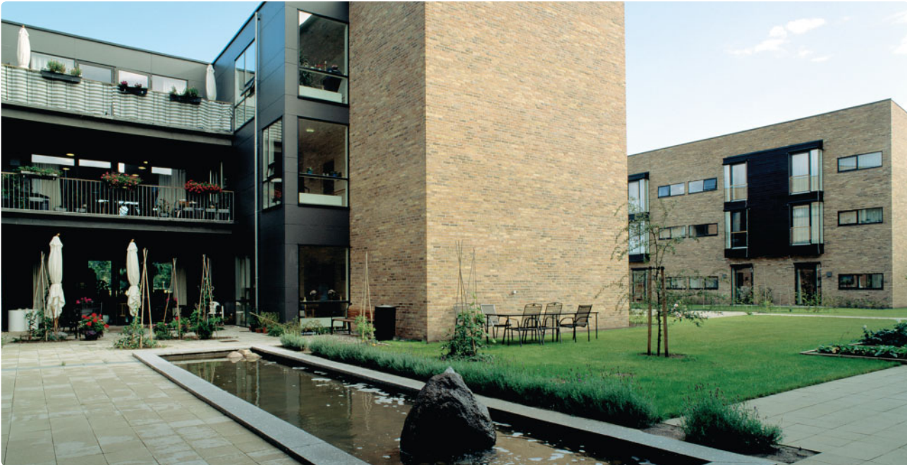
Arkitema, Christians Have Care Center, Solrød, Denmark, 2010
