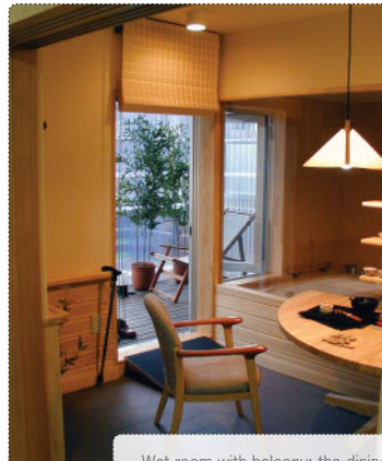
Wet room with balcony; the dining table in the foreground folds down to allow the sliding partition doors to close between the dry and wet spaces.
