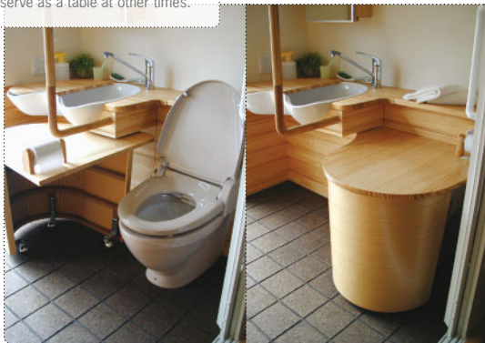
The toilet includes a wheeled cover which slides under the handrail when the toilet is in use and can serve as a table at other times.
