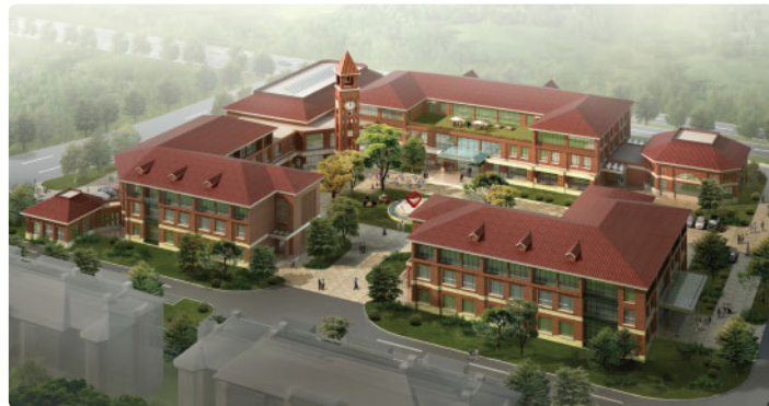
below bottom: Aerial view of the entire site showing the southern portion in the foreground and northern portion behind.
