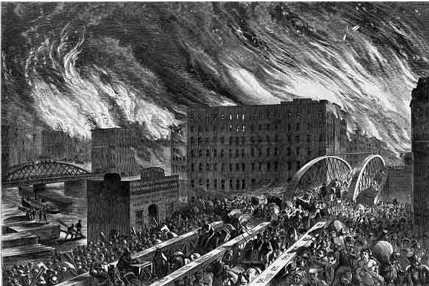
Figure 7.1 An artist's rendering of the Great Chicago Fire of 1871 that triggered ad hoc legislation by Congress for disaster relief. (Source: Harper's Weekly .)
