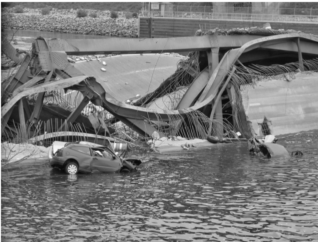
Figure 11.2 Incidents like the 2007 Minneapolis bridge collapse make the public aware of local struggles to maintain aging physical infrastructure in many communities. (Source: FEMA/Todd Swain.)
