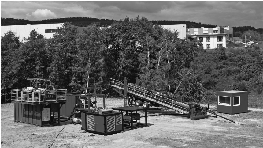
Figure 5.88 Example of a large HDD rig and associated facilities, pumps and mud recirculation system (courtesy of Prime Drilling HDD-Technology)
