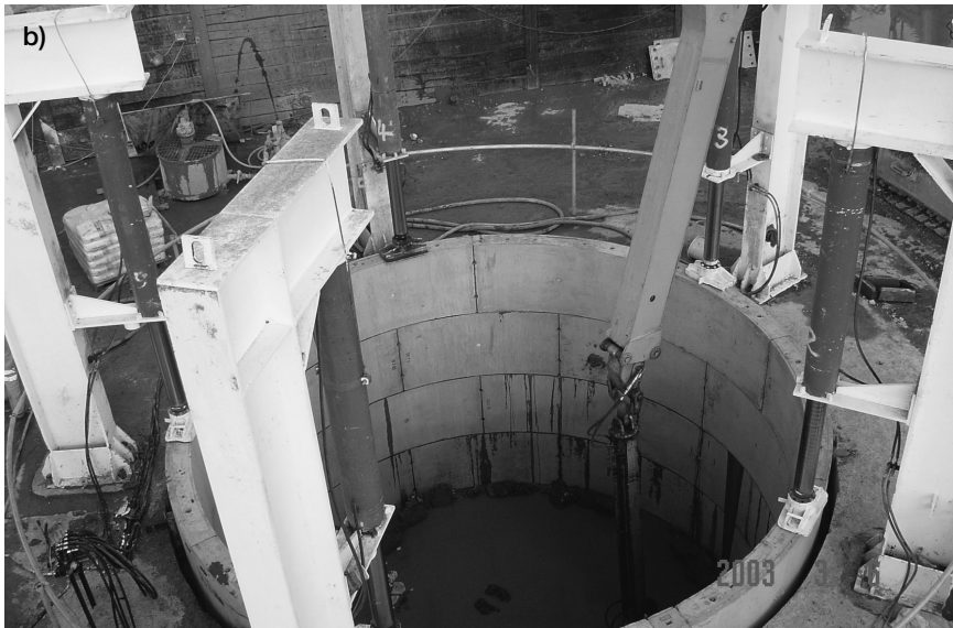
Figure 4.27 a) Caisson-sinking method to construct shafts (after BTS/ICE 2004, used with permission from Thomas Telford Ltd), b) shows the construction of a reception shaft for a pipe jacking operation as part of the Terminal 5 project at Heathrow, UK
