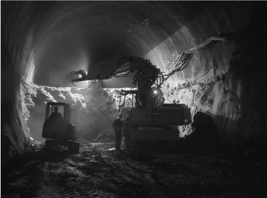
Figure 5.47 Example of a NATM crown and bench excavation during the construction of the Katschberg Tunnel, Austria
