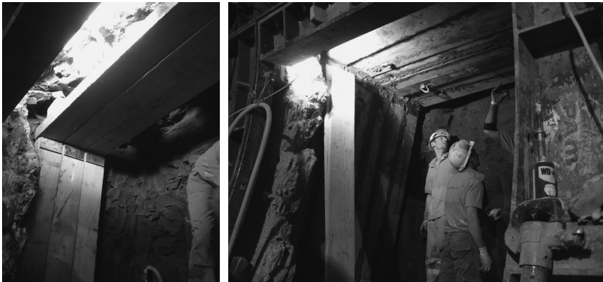
Figure 5.1 Timber heading as used in London Clay for constructing a connecting passage between two other tunnels (approximately 30–80 m 2 ), King's Cross Station upgrade, London (construction period 2002–2008) (courtesy of ALPINE BeMo Tunnelling GmbH Innsbruck)
