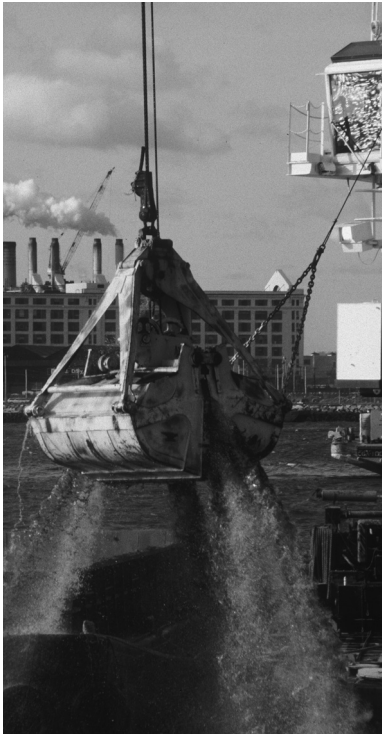
Figure 5.67 The trench was excavated using floating cranes with grab excavators (courtesy of Massachusetts Turnpike Authority)
