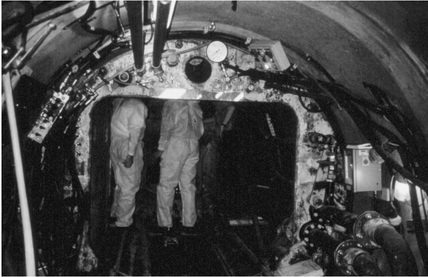
Figure 4.16 Airlock arrangement on a pipe jacking project for a new sewer in Germany (see section 5.11 for a description of pipe jacking)
