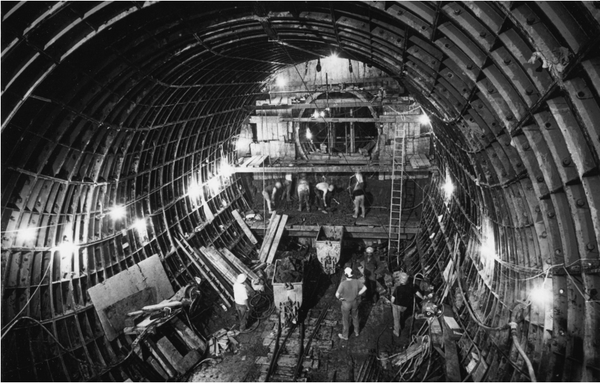
Figure 5.2 Construction of an escalator tunnel at The Angel Islington Station, London Underground, UK (completed in 1990). The tunnel was constructed at an angle of 30^\circ to the horizontal and used a pilot bore (3.7 m in diameter), which was then enlarged to the final diameter of 7.5 m (courtesy and copyright London Underground)
