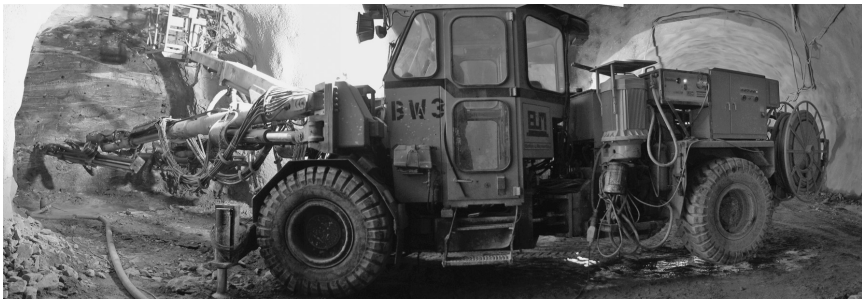
Figure 5.34 Example of a rubber tyred drilling carriage 'jumbo' as used on the 2nd tube of the Katschberg Tunnel, Austria (details are provided in section 4.3.3)
