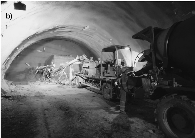
Figure 4.19 a) Manual spraying and b) Spraying equipment used during the construction of the Lainzer Tunnel LT31 in Vienna, Austria
