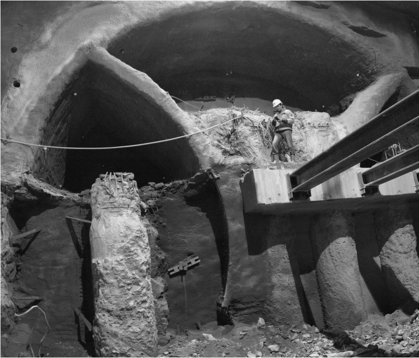
Figure 8.19 Crown excavated, and enlargement of leading side wall drift started. Remaining bracing still in place
