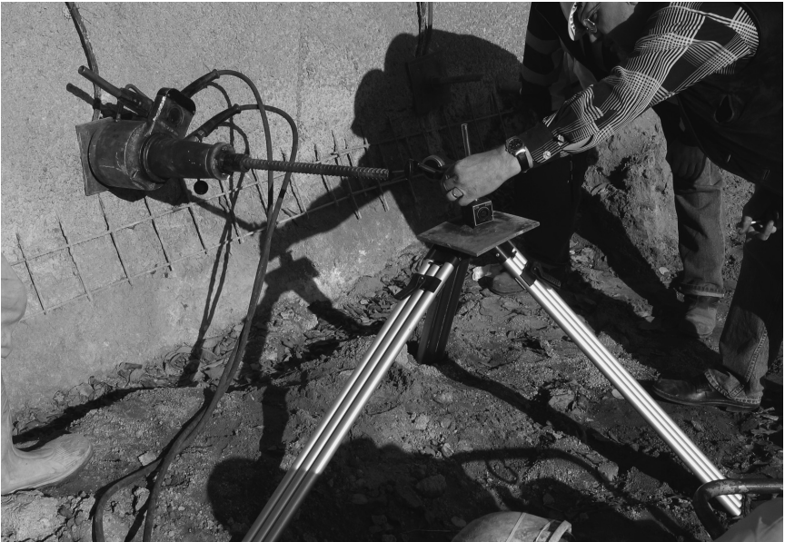
Figure 4.10 Load testing of an anchor, Lainzer Tunnel LT31, Vienna, Austria
