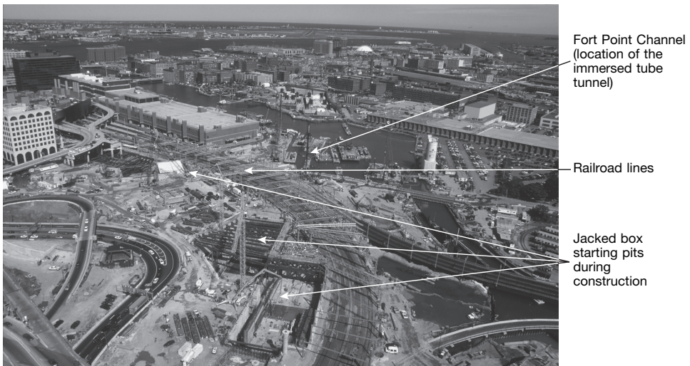
Figure 5.77 An overview of the jacked box sites in Boston showing the railroad lines and Fort Point Channel (courtesy of Massachusetts Turnpike Authority)
