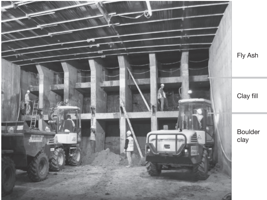
Figure 5.74 Rear view of the cellular reinforced concrete shield (annotation indicates the ground strata) (Allenby and Ropkins 2004, courtesy of BAM Nuttall Ltd and John Ropkins Ltd)
