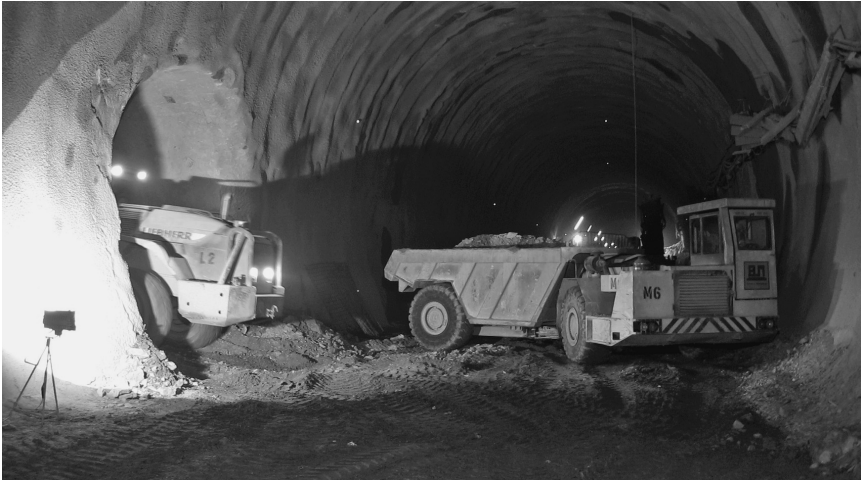
Figure 5.49 Example of mucking equipment used during the construction of one of the emergency cross passages of the Katschberg Tunnel, Austria
