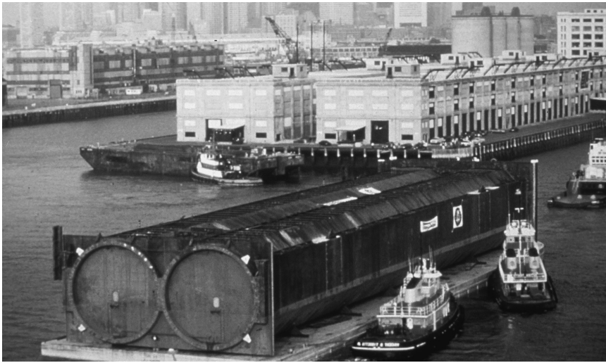
Figure 5.66 One of the tunnel elements for the Ted Williams Tunnel being towed prior to additional outfitting work (courtesy of Massachusetts Turnpike Authority)
