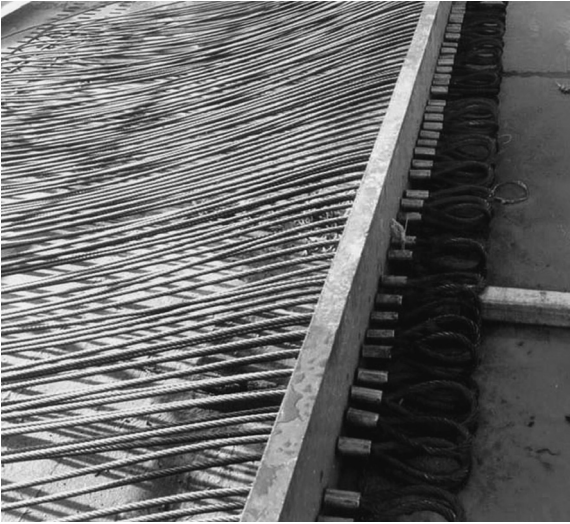
Figure 5.72 Top anti-drag system as used in the proprietary Ropkins™ system (Ropkins and Allenby 2000, courtesy of BAM Nuttall Ltd and John Ropkins Ltd)
