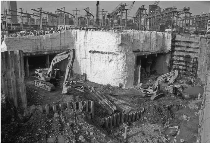
Figure 5.79 Breakthrough of two of the jacked tunnels, showing the freezing operation at the ground surface (courtesy of Massachusetts Turnpike Authority)
