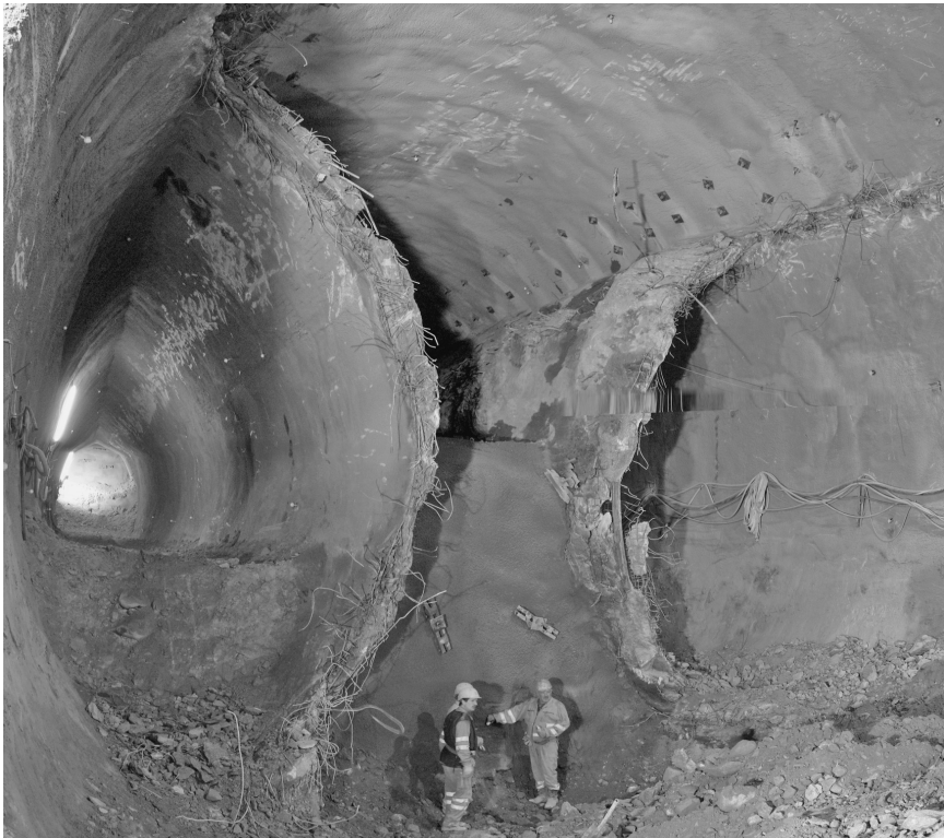
Figure 8.23 Construction of the invert at the total cross section (excavation Kern2 and demolition of inner walls of side wall drift)
