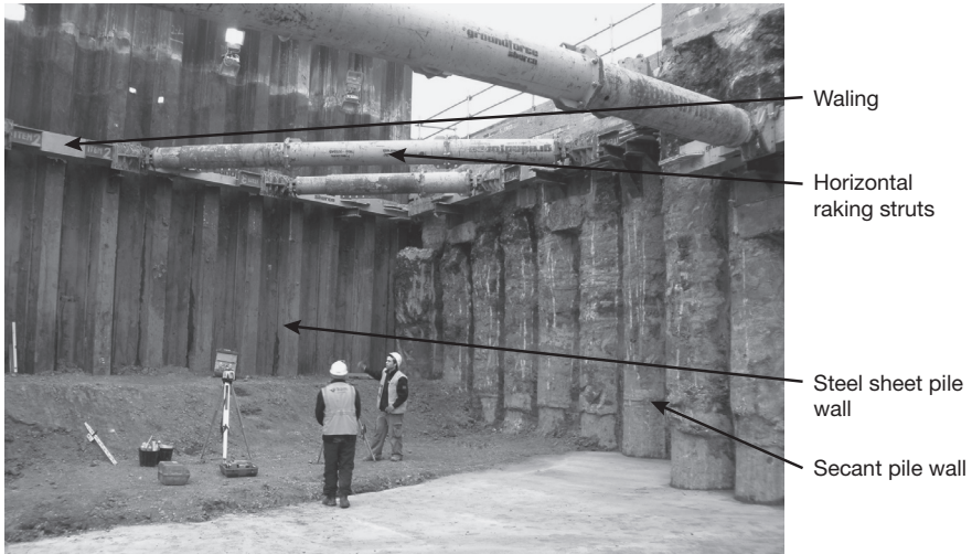
Figure 5.59 Secant pile wall as used as part of the jacking pit for a jacked box tunnel at Owen Street, Tipton, UK (see section 5.10 on jacked box tunnels). The photograph also shows the steel sheet pile headwall with its waling and horizontally raking struts transferring the headwall loading into one of the secant piled sidewalls (courtesy of BAM Nuttall Ltd and John Ropkins Ltd)
