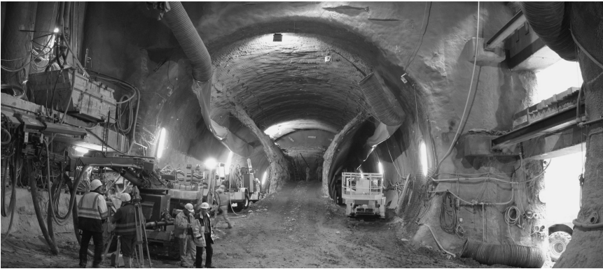
Figure 8.20 30 m of total cross section (on the RHS, the open oval section, the remainder of the lower most bracing can be seen still in place)
