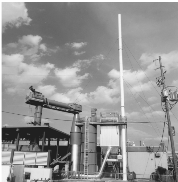
Figure 7.1 Baghouse with preconditioner (Bundy Environmental, Inc.).
