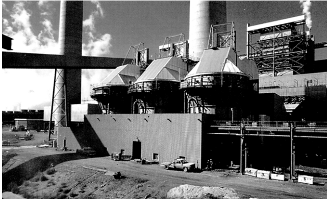
Figure 14.2 Utility FGD system (Babcock & Wilcox Company).
