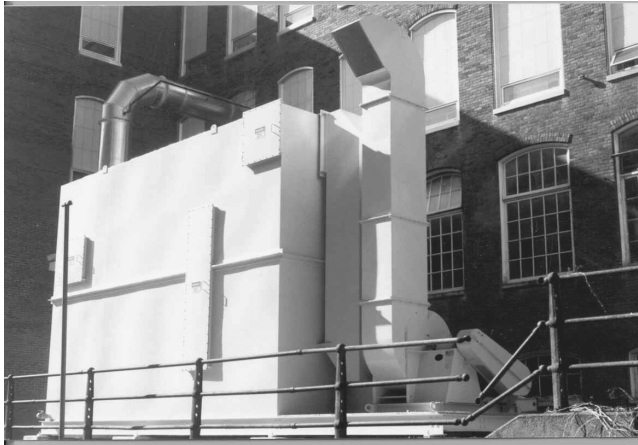
Figure 8.5 30,000 ACFM system on tenter frame (Advanced Environmental Systems, Inc.).
