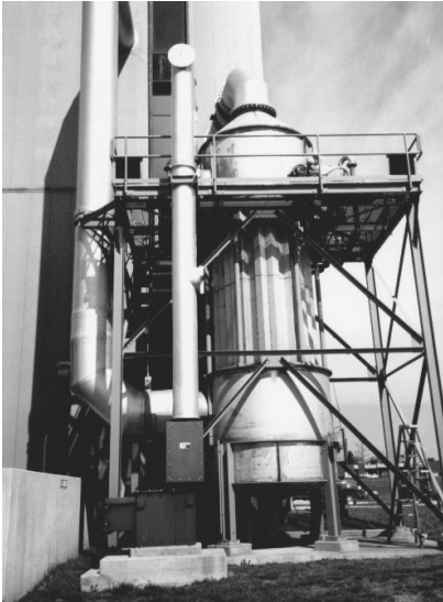
Figure 20.6 Picture of sonic development WESP designed and serviced by Wayne T. Hartshorn.
