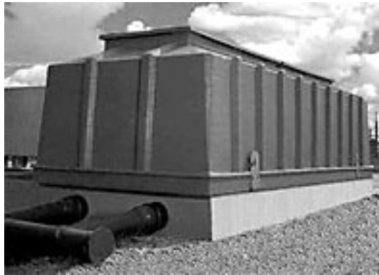
Figure 3.4 Modular biofilter (Envirogen).
