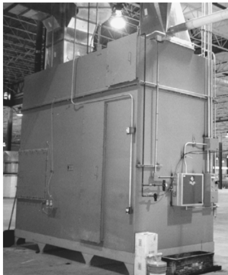
Figure 8.3 10,000 ACFM system with prefilters (Advanced Environmental Systems, Inc.).
