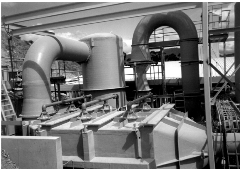
Figure 9.2 Crossflow meshpad type scrubber (Bionomic Industries Inc.).
