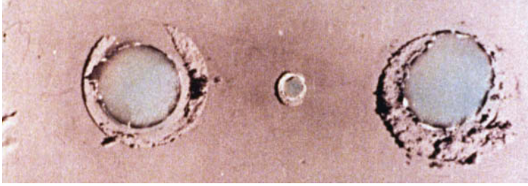
Figure 16.15 On this plate, which was immersed in seawater, crevice corrosion has occurred at the regions that were covered by washers.
