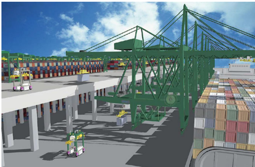
Fig. 1.20 Multiple access points for loading/unloading containers by quay cranes
