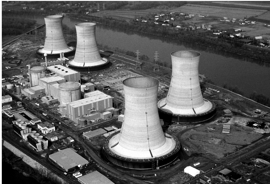
FIGURE 14-23 Three Mile Island nuclear power station near Middletown, Pennsylvania, after the accident at the TMI-2 plant, whose cylindrical (silo-type) reactor containment building and two cooling towers are in the foreground. From Pierce, William C., “A Nuclear Nightmare.” Time , April 9, 1979. Used by permission of TimePix, a department of Time Inc.
