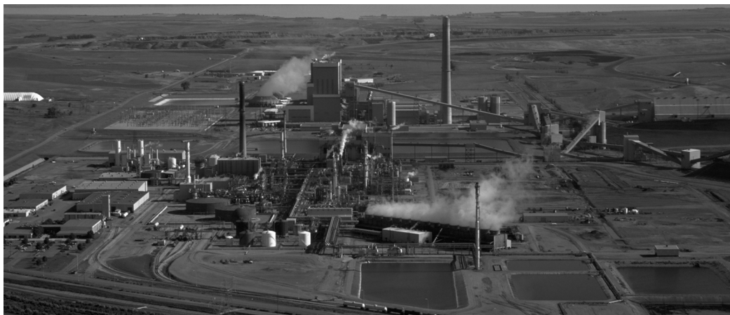
FIGURE 15-4 The Great Plains Gasification Facility in Beulah, North Dakota, for the generation of methane from coal. The gasification facility is in the foreground. Electricity is generated from the coal fines, which are not suitable for methane synthesis, in the power plant shown in the background next to the large smokestack. Photograph provided by Fred Stern at GPGE.
