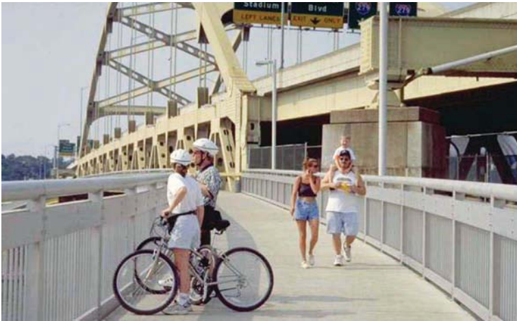
Figure 5-12. Example of Bridge Structures (Photo courtesy of Jennifer Toole of Toole Design Group.)
