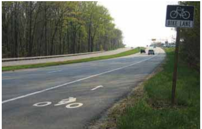
Figure 4-10. Example of Paved Shoulder Designated as Bicycle Lane (Photo courtesy of Michael E. Jackson.)
