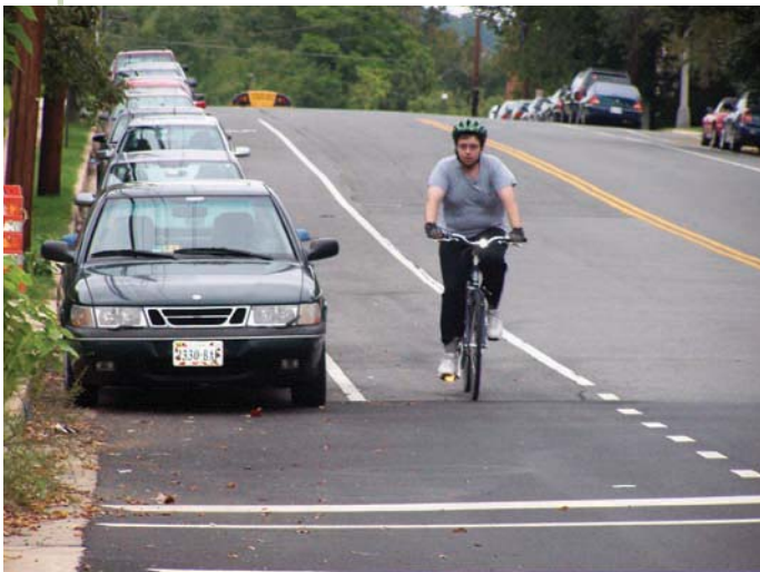
Figure 4-14. Example of Bike Lane Adjacent to Parallel Parking (Photo courtesy of Jennifer Toole of Toole Design Group.)
