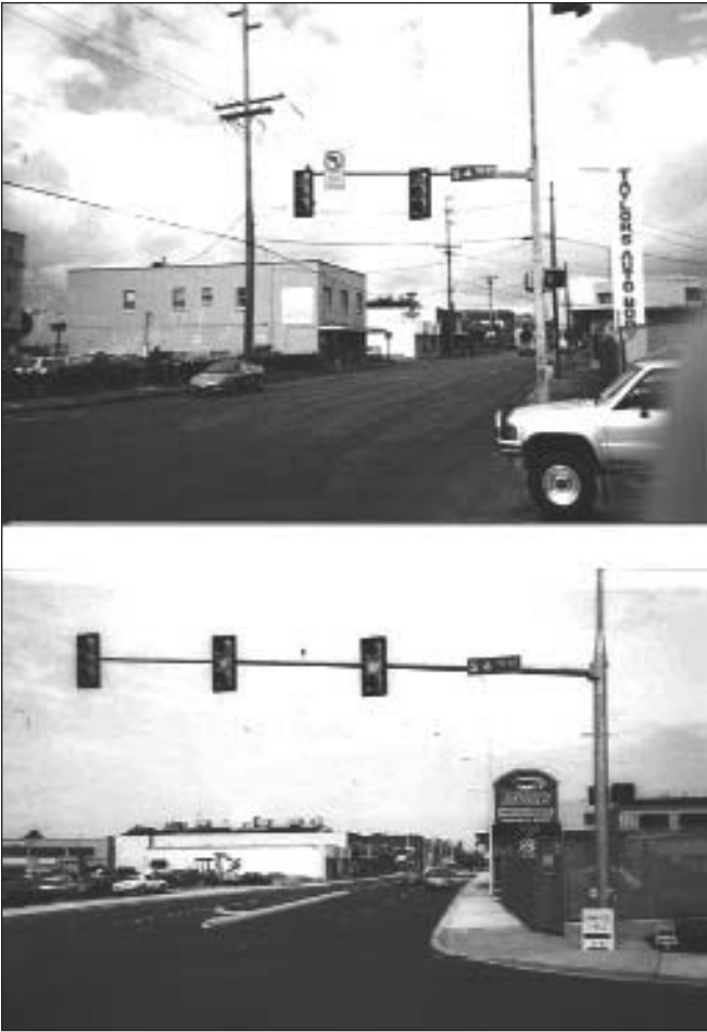
FIGURE 3-5 Placing Utilities Underground Improves Urban Clear Zones and Corridor Aesthetics
