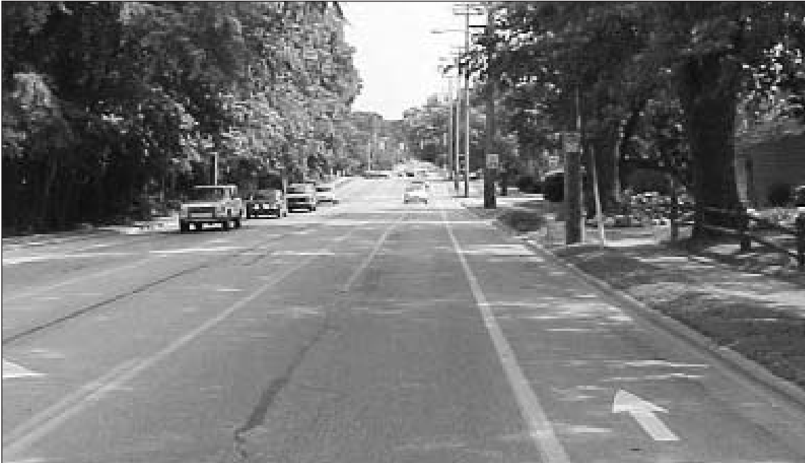
FIGURE 3-9 Conversion of Four-Lane Roadway to Two-Lane Roadway with Center Turn Lane and Directional Bike Paths
