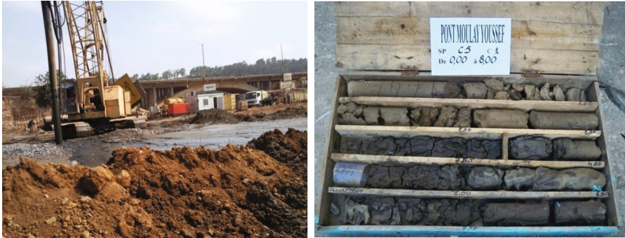
Fig. 1. Soil reinforcement of the Bouregreg Valley and removal of samples for laboratory tests
