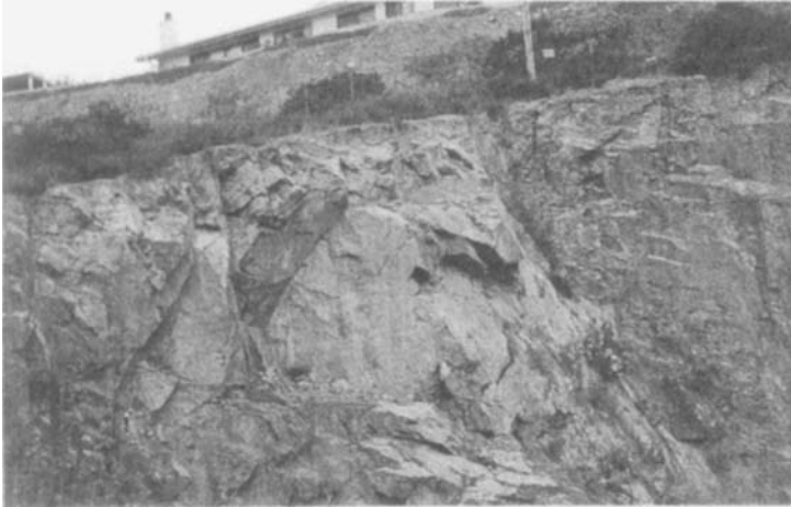
Figure 9-22 Rock wedge fallout.
