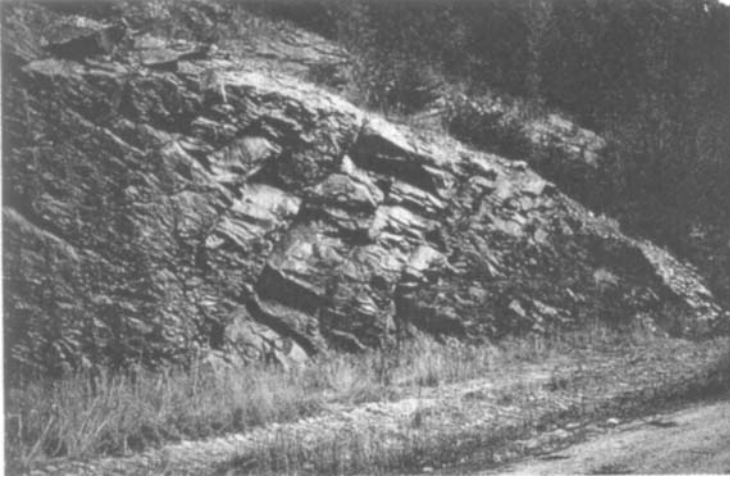
Figure 9-25 Toppling failure conditions.
