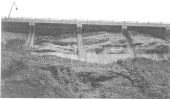
Figure 9-34 Rock slope buttress.
