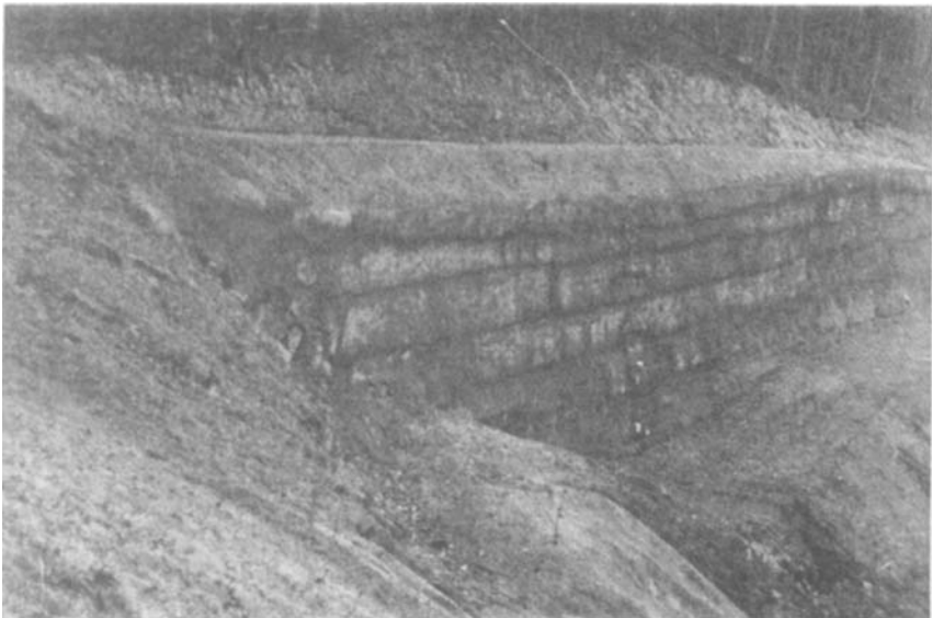
Figure 5-11 Nail support of the Cumberland Gap wall.
