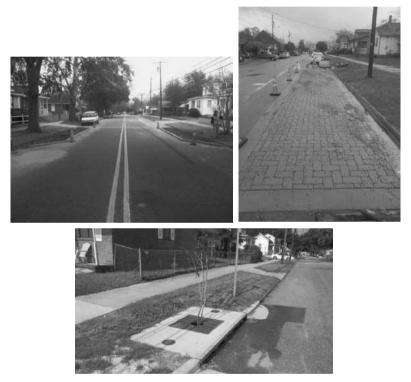
**Figure 1:** Clockwise from top: BRC bumpouts along Dock Street, permeable pavement parking stalls on 12<sup>th</sup> Street, and atree filter device at intersection of 12<sup>th</sup> Street and Dock Street.
