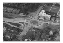
Figure 7. The Morgan Street Roundabout included lower construction and life cycle costs compared to a signaled intersection.
