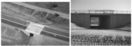
Figures 3 and 4: Wildlife crossings under construction on the SR 76 middle segment
