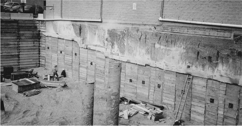
**FIG. 5. Hand dug underpinning, Denver, CO**
