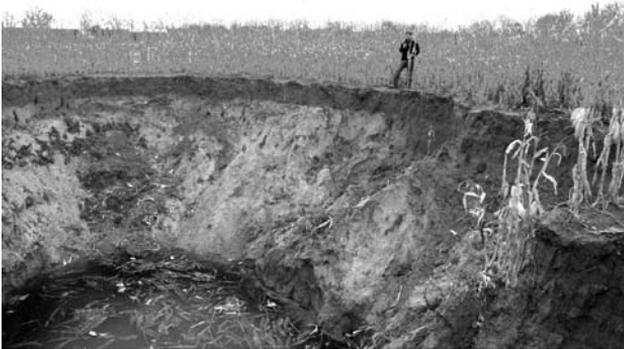
**FIG. 1. Large mine-induced sinkhole in Erie, Colorado**
