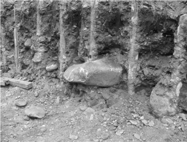
**FIG. 9. Soil Arching between Grout Columns and Pre-Splitting Boulders**
