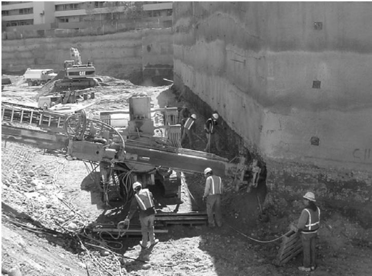
**FIG. 6. Drilling Bottom Row of Soil Nails**
