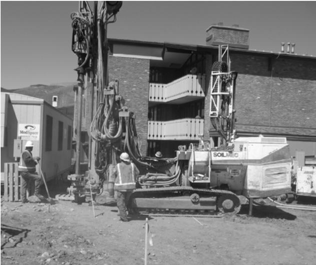
**FIG. 2. Drilling Grout Columns for Soil Nail Earth Retention**
