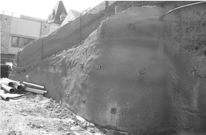
**FIG.3. Temporary soil nail wall**
