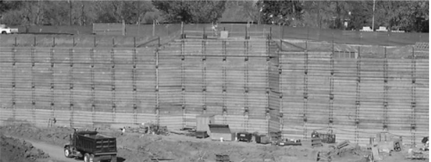
**FIG. 4. 12.2 meter (40 foot) deep excavation with 100mm (3 inch) lagging, Colorado Springs, CO**
