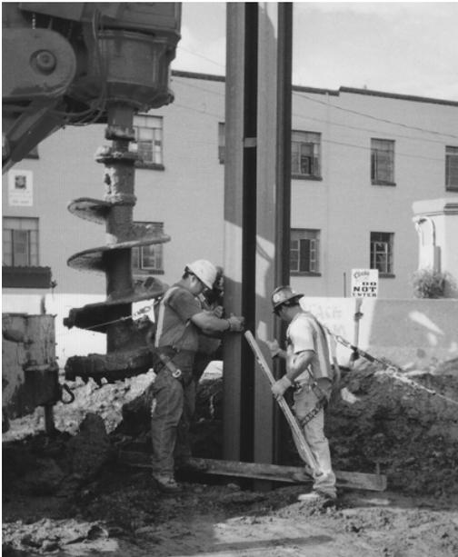
**FIG. 3. Setting drilled soldier beam, Denver, CO**
