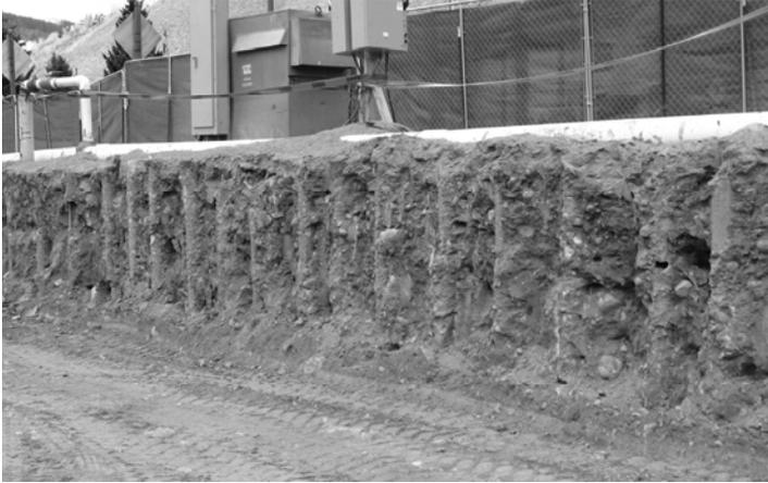
**FIG. 3. Initial Excavation and Exposed Grout Columns**
