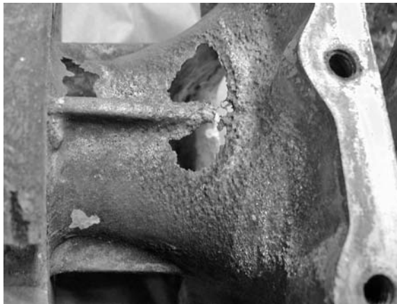
PHOTO 7.17 The heavily pitted surface caused by elevated temperatures.
