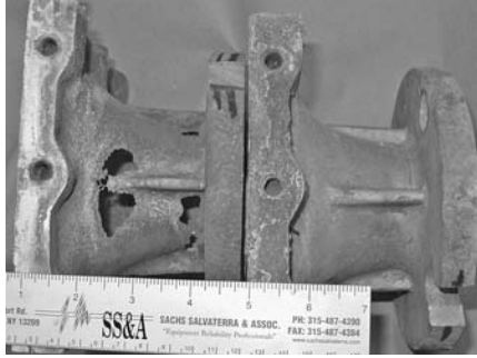
PHOTO 7.16 Pitting corrosion on one of two aluminum castings.
