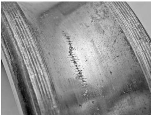
PHOTO 10.36 This pump bearing was rotating when the welding arc left this tell-tale track.
