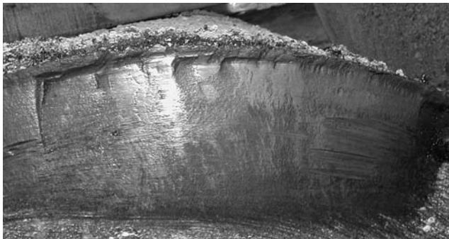
PHOTO 5.6 These multiple ratchet marks result from many crack origins — either from high stress and/or from high stress concentrations.
