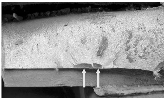
PHOTO 4.16 A close up view of the fracture origins showing the block, oxide-coated casting defect that hastened the failure.
