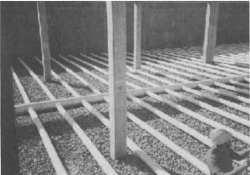
FIGURE 9.2 Underdrain installation.
