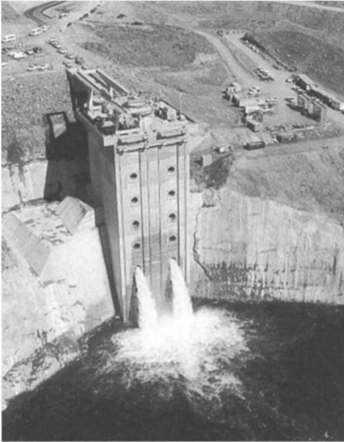
FIGURE 4.7 Diamond Valley Lake inlet/outlet tower.
