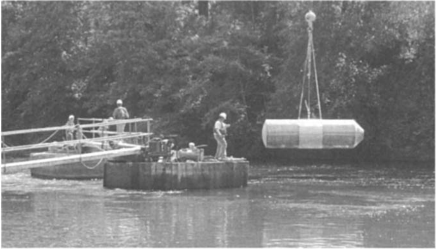
FIGURE 4.17 T screen used to modify intake to improve fish protection.
