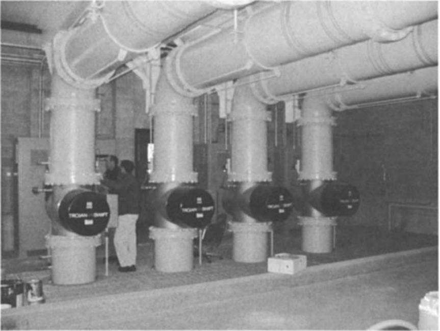
FIGURE 29.13 UV reactor oriented vertically. (Photo courtesy of City of Albany, New York.)
