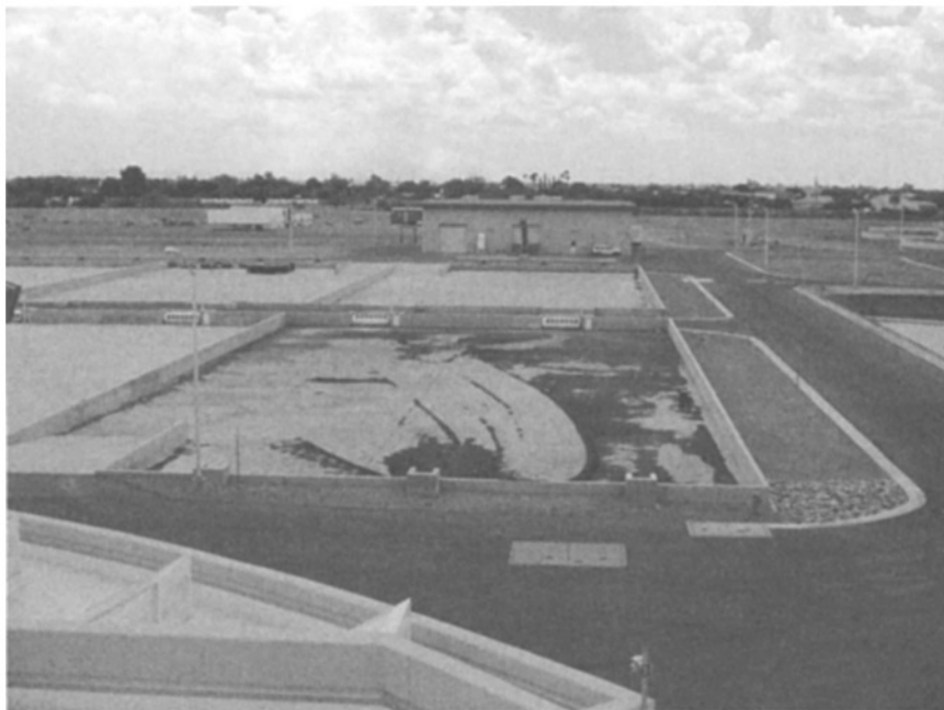
FIGURE 17.13 Solar drying bed. (Courtesy of City of Phoenix Water Services Department.)
