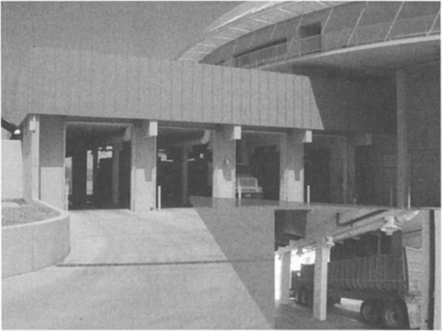
FIGURE 17.26 Truck unloading system. (Courtesy of City of Phoenix Water Services Department.)
