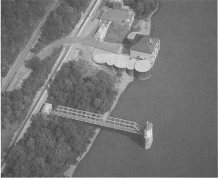
FIGURE 4.3 Ohio River intake (shore structures).
