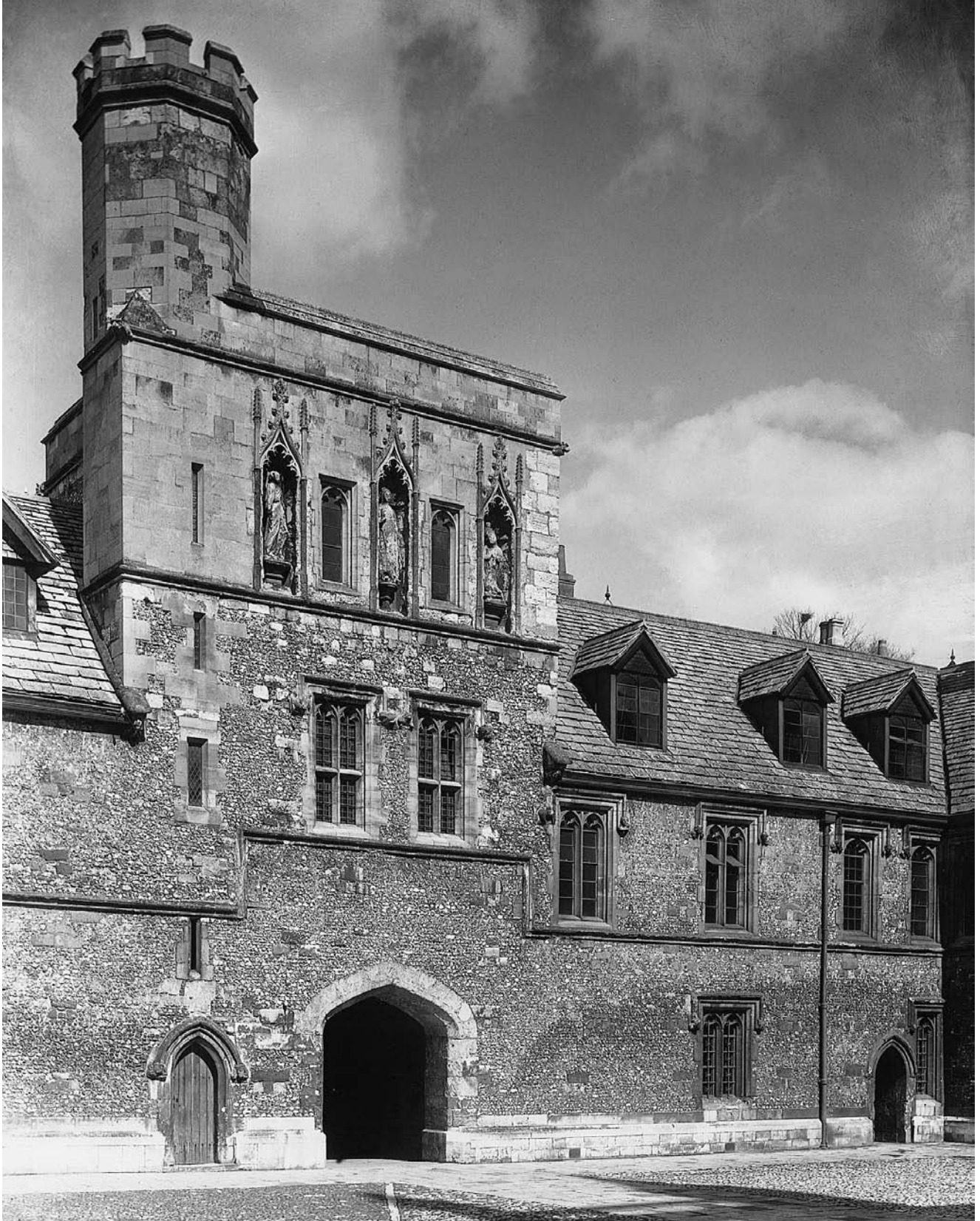
PLATE 103 Winchester College: inner gate to Chamber Court
