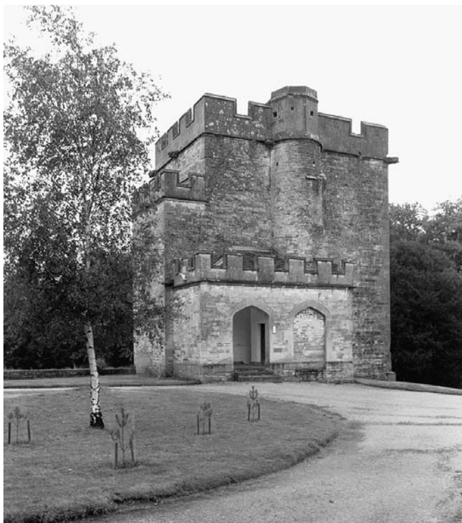
PLATE 259 Newton St Loe Manor: tower from the west
