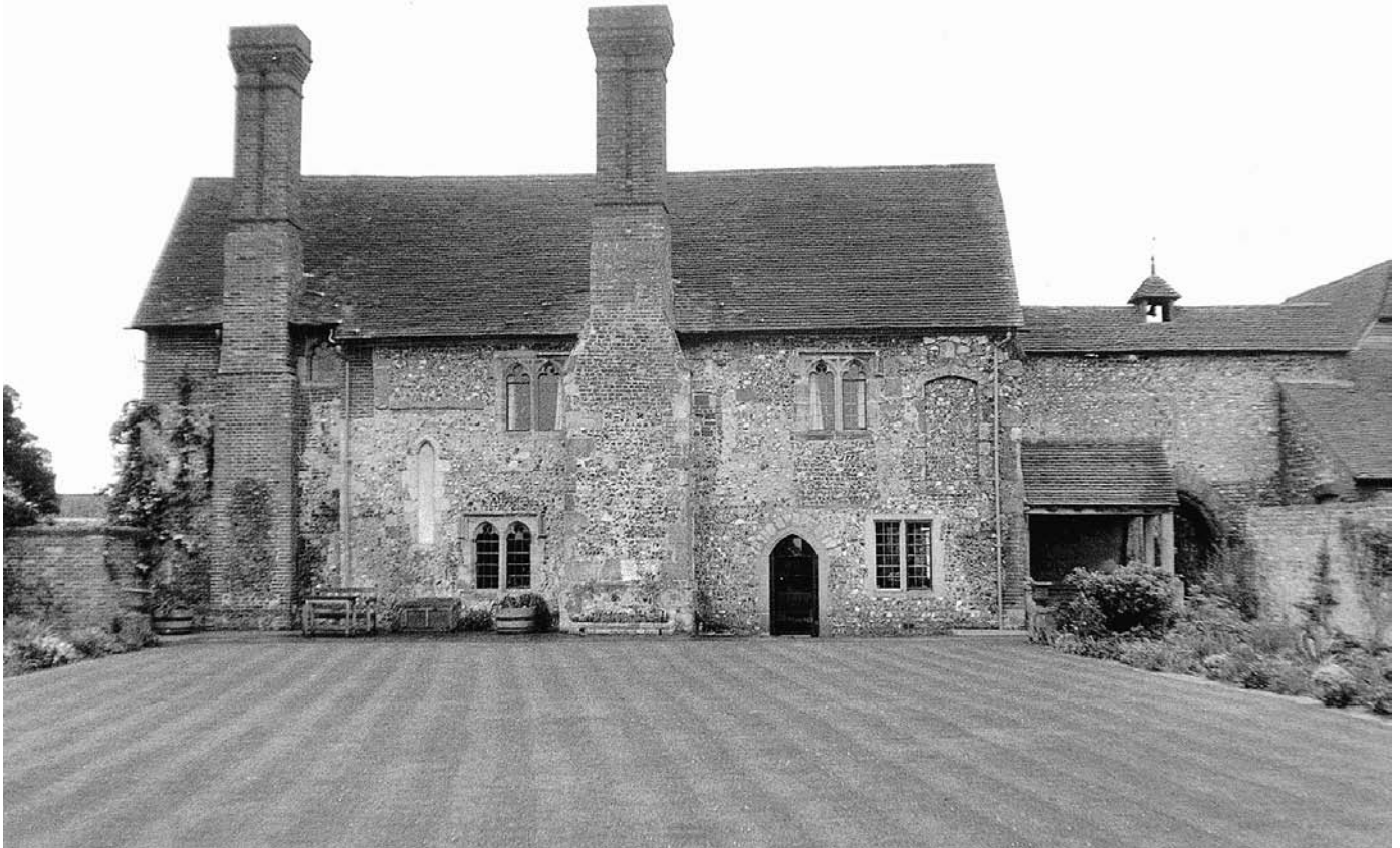
PLATE 170 Swanborough Manor: hall range from the north
