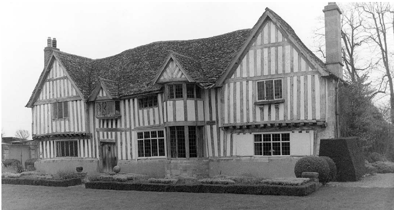
PLATE 84 Yelford Manor: from the south-west
