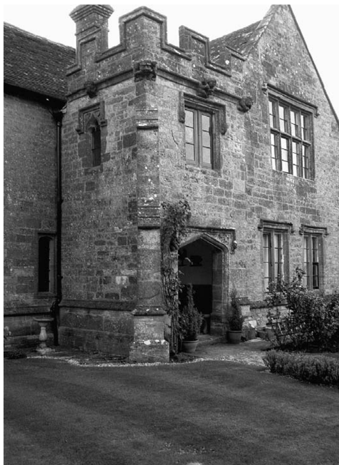
PLATE 186 Childhay Manor: hall porch
