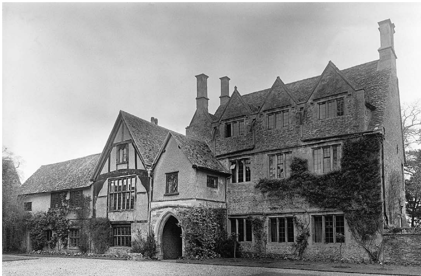
PLATE 42 Fyfield Manor, south front
