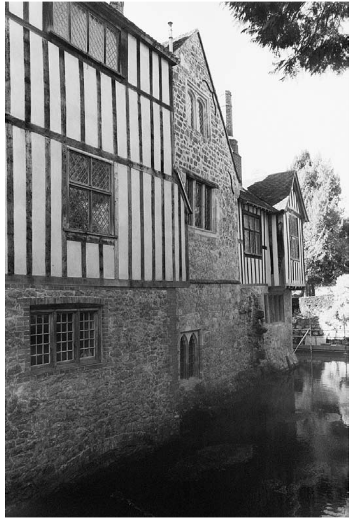
PLATE 148 Ightham Mote: from north-east showing stone chapel block, garderobe chute of additional residential block, and post-medieval framed additions
