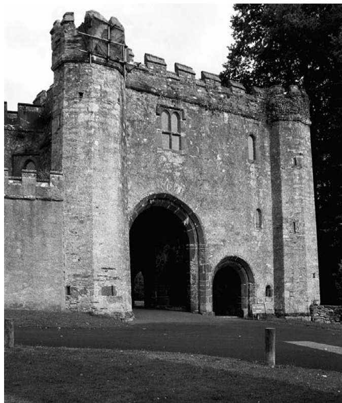
PLATE 283 Torre Abbey: inner gate
