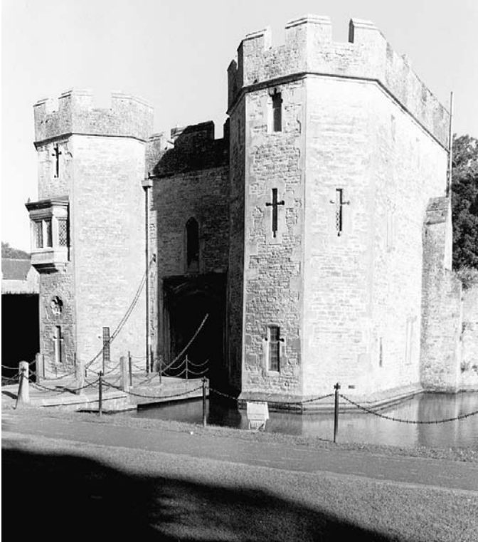
PLATE 196 Wells, Bishop's Palace: Bishop Ralph's entry gate (c.1340)
