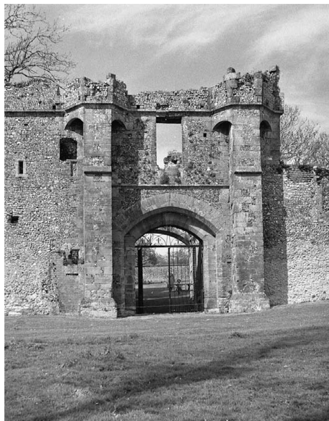
PLATE 140 Halnaker House: gatehouse from the south
