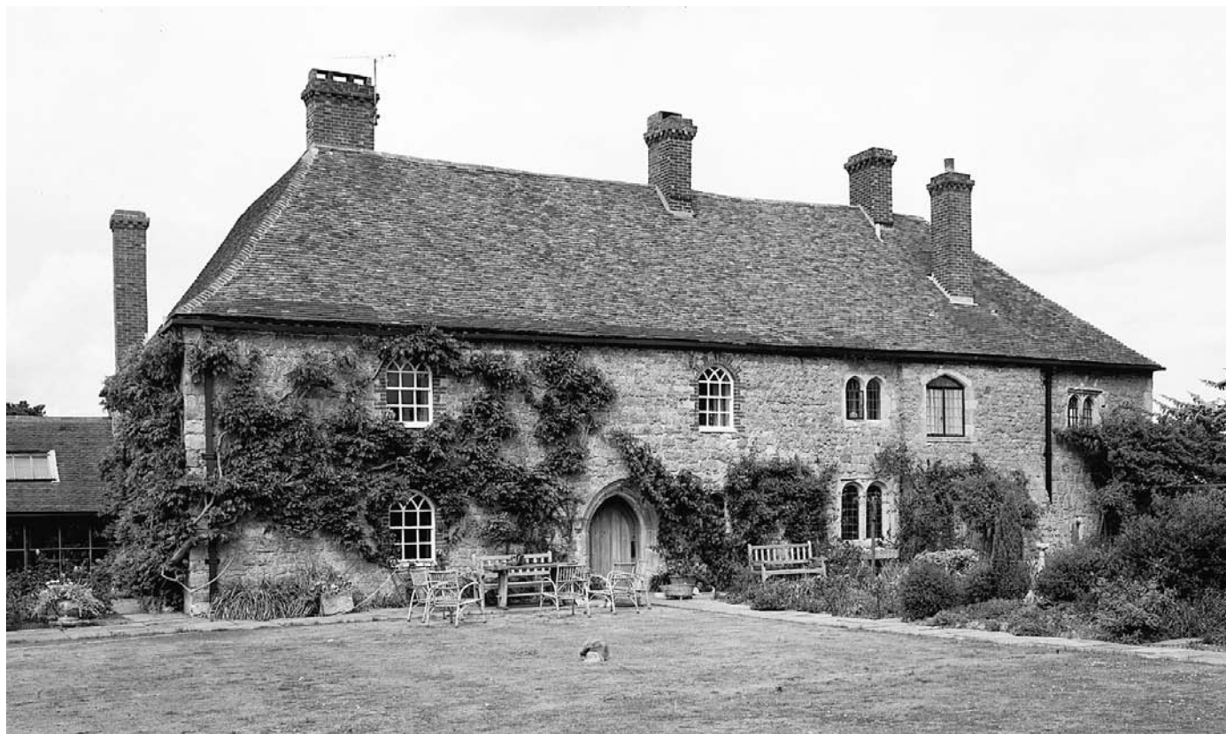
PLATE 119 Battel Hall: from the east
