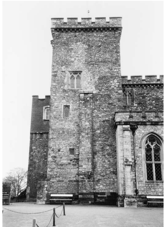
PLATE 267 Powderham Castle: north-west tower from present entry court
