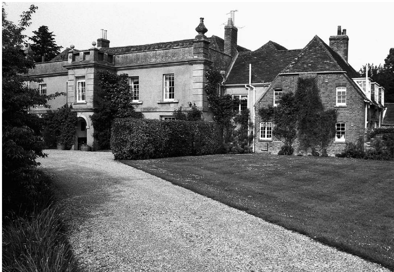
PLATE 182 Wonston Old House: from the south-west
