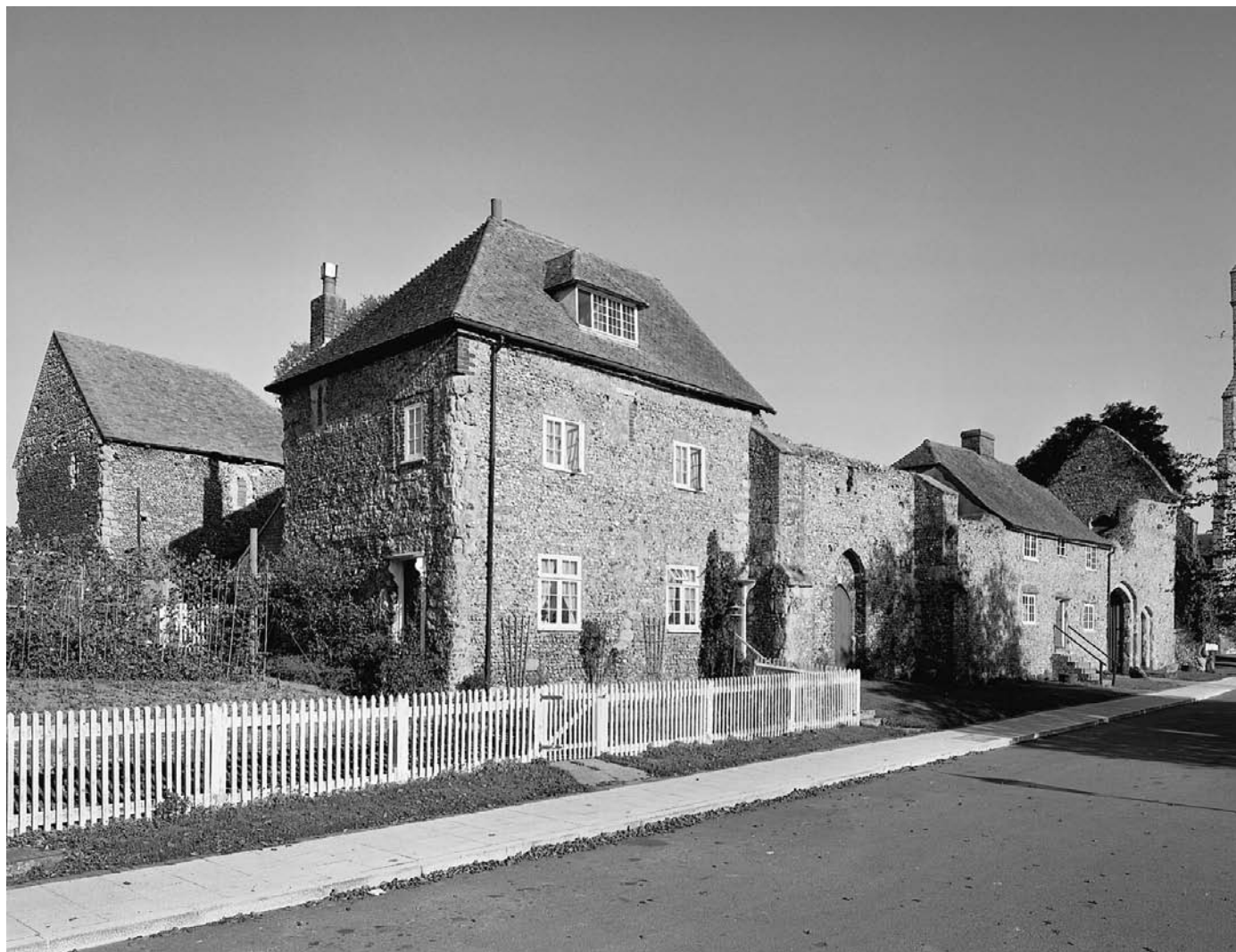
PLATE 130 Charing Palace: garderobe projections, lodging ranges, and gatehouse from the Market Place
