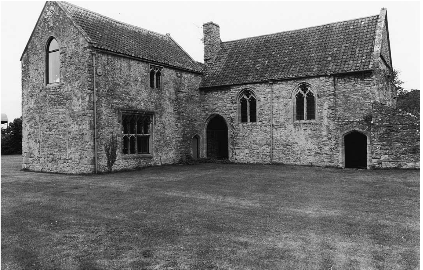
PLATE 280 Tickenham Court: hall and parlour wing from the east
