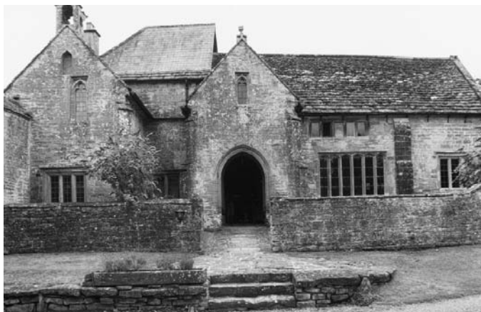
PLATE 277 Stoke Sub Hamdon Priory: hall range from the forecourt
