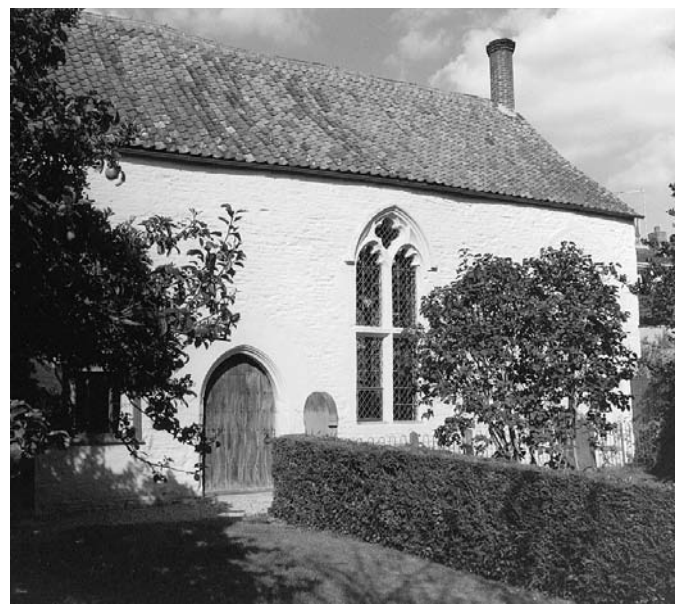
PLATE 227 Croscombe Hall: from the south
