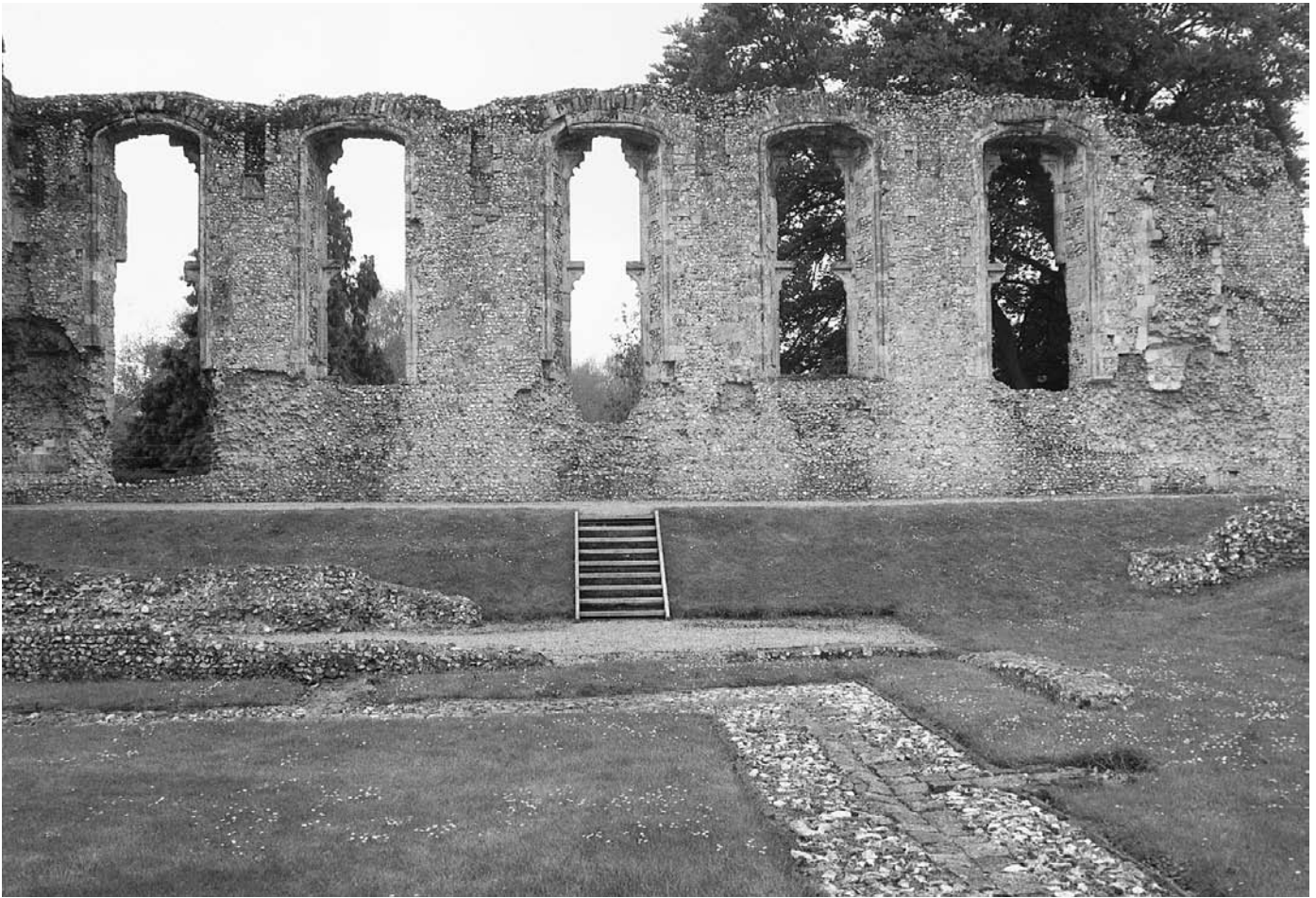
PLATE 125 Bishop's Waltham Palace: hall interior towards windowed outer wall
