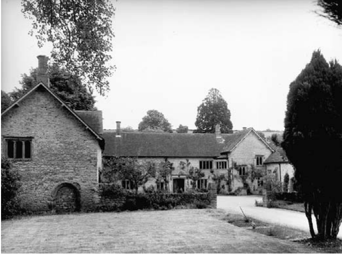
PLATE 268 Poyntington Manor: entrance range, residential range, and hall
