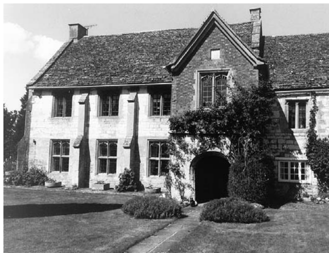
PLATE 18 Ashbury Manor: entry frontage
