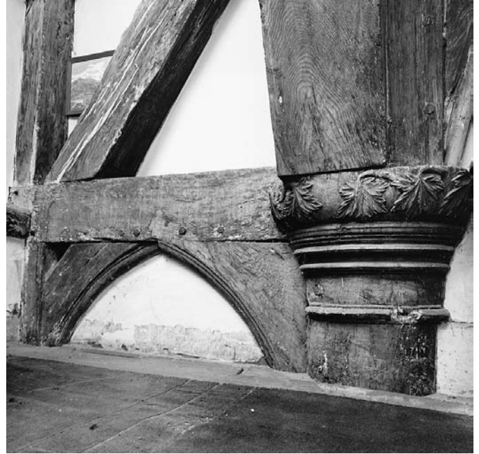
PLATE 157 Nurstead Court: hall aisle column and capital
