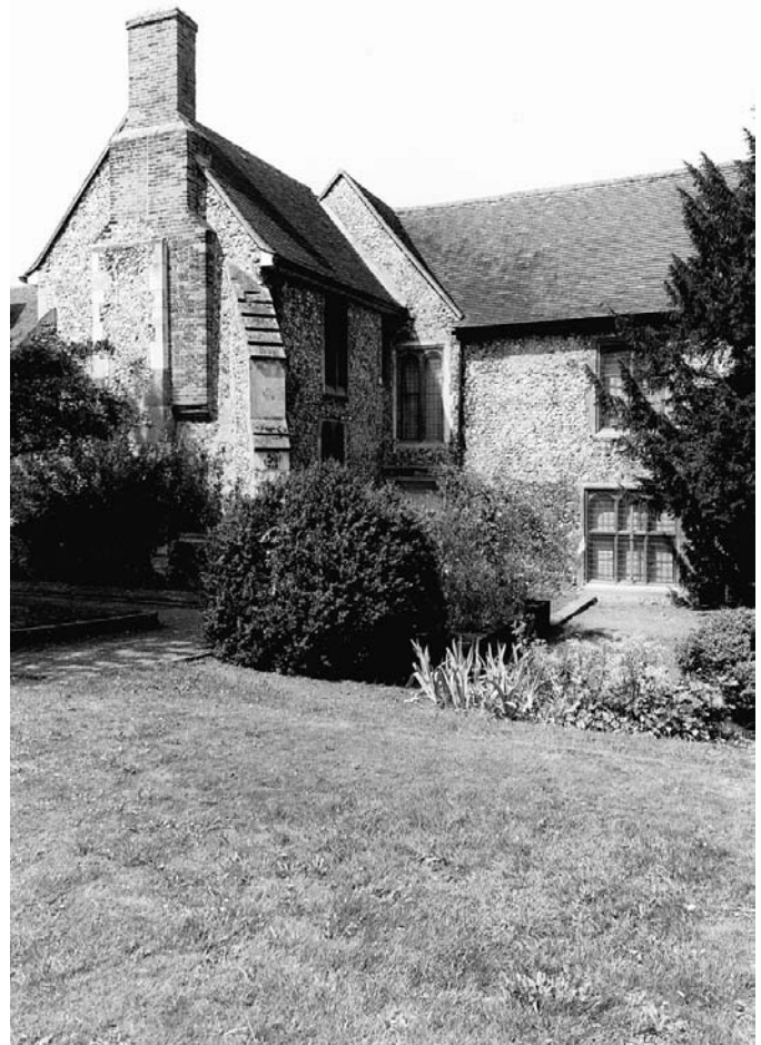
PLATE 159 Orpington 'Priory': camera and upper chamber blocks from the east
