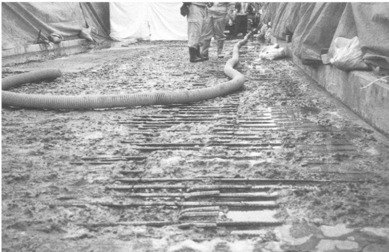
Figure 5.18 'Standing water' during a hydrodemolition job (Photograph: Aquajet AB, Holsbybrunn)
