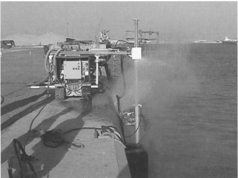
Figure 1.3 Modern hydrodemolition robot (photograph: Aquajet A.B., Holsbybrunn)
