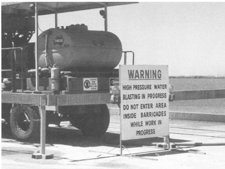
Figure 4.14 Warning sign for a hydrodemolition site
