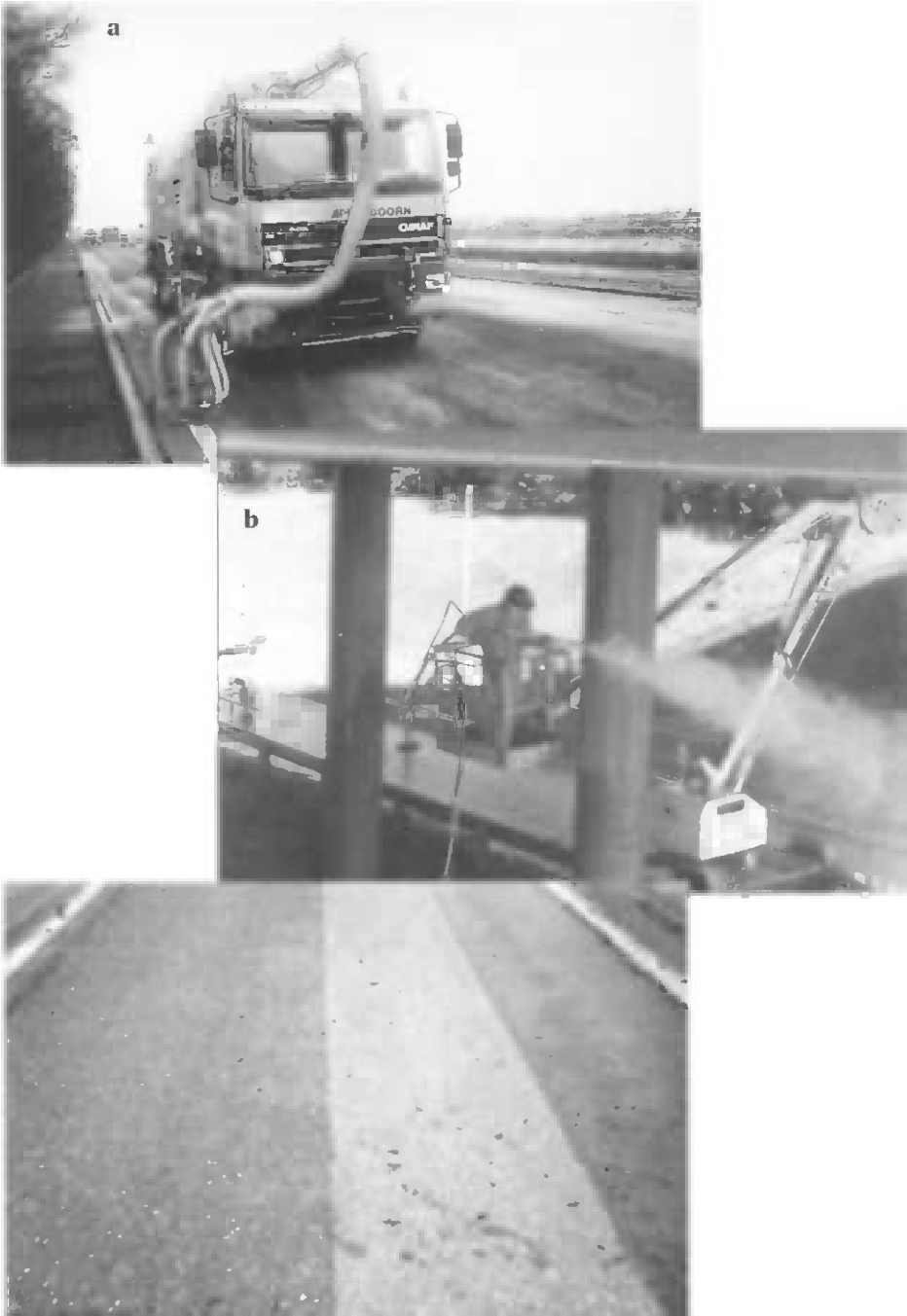
Figure 4.1 Applications of water jets to concrete substrates (photographs: WOMA Apparatebau GmbH, Duisburg) a – removal of paint b – removal of coatings c – roughening
