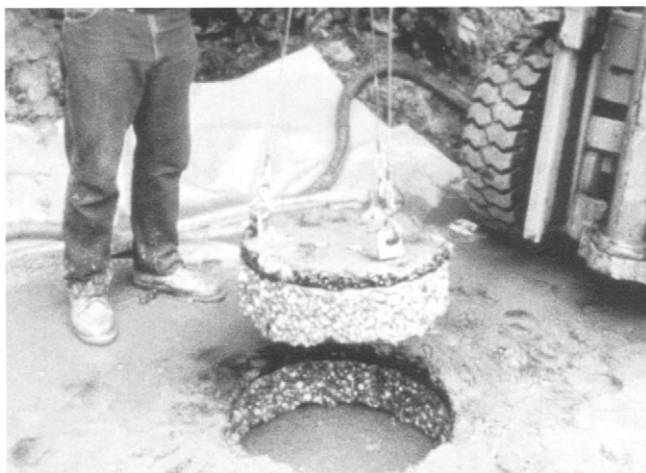
Figure 7.31 Pavement element cut with cavitating water jets (photograph: Dynaflo, Inc., Jessup)
