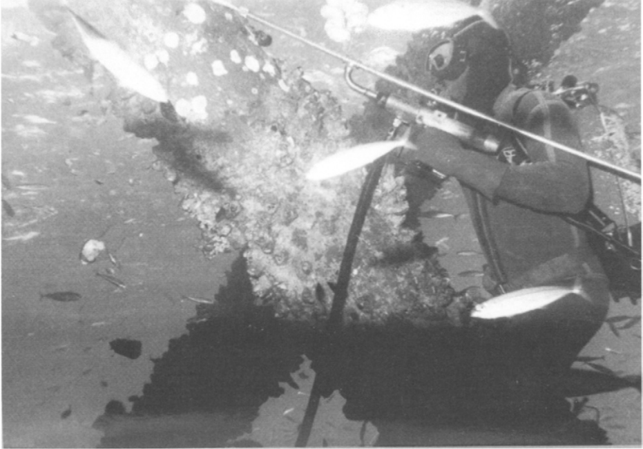
Figure 4.10 Submerged cleaning of a concrete column (photograph: WOMA Apparatebau GmbH, Duisburg)
