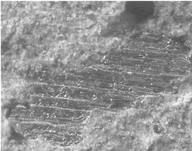
Figure 6.37 Steel-fibre in reinforced concrete cut during hydro-abrasive erosion (Hu et al., 2002)
