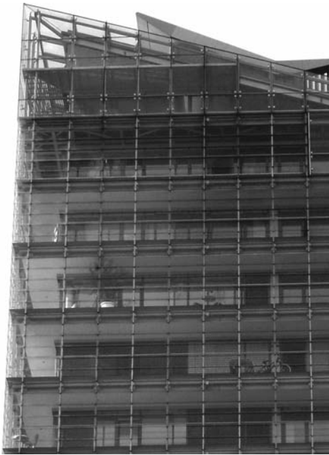
Figure 17 Double-skin glass louvered façade for an apartment building in Manchester, U.K. (architect: Ian Simpson Architects)
