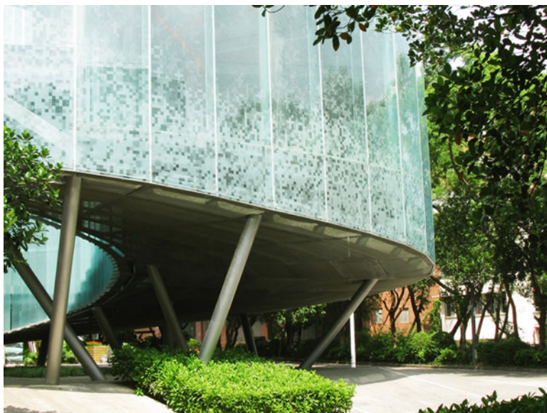
Fig. 14.6 Corridor and landscape parergon design of the second stage of OCT (Liao H 2012)
