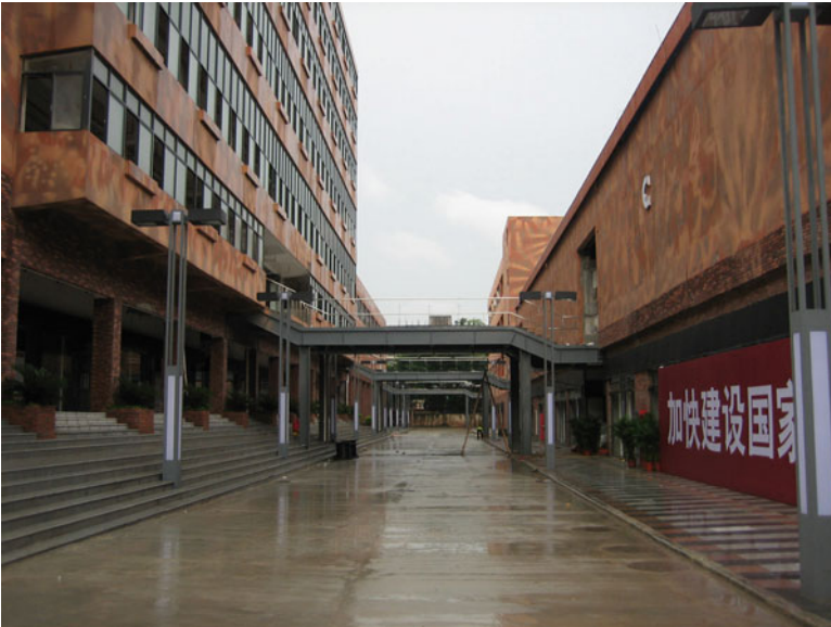
Fig. 9.10 Reused buildings in Wuyang-Honda Factory complex, Guangzhou, with paint simulating brick and corrugated iron façades (Uwe Altrock 2012)
