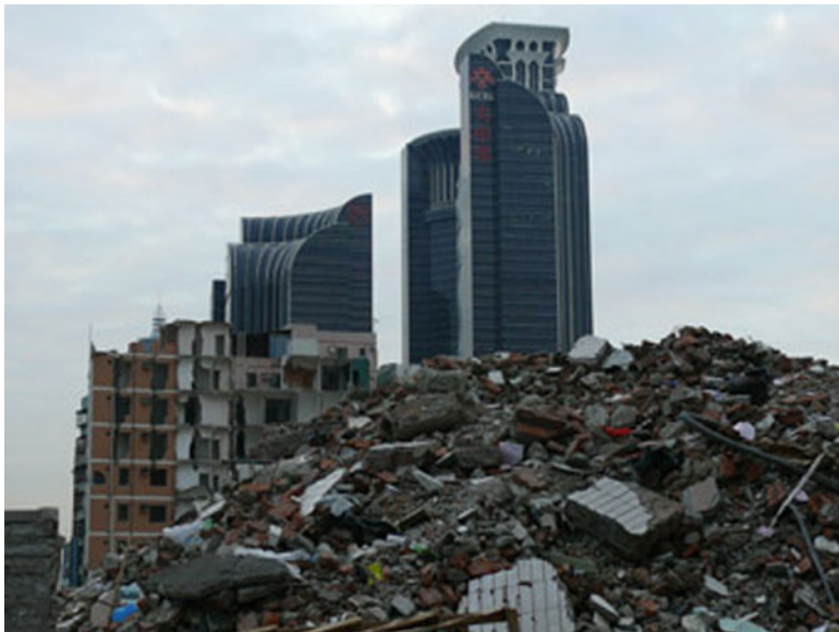
Fig. 1.5 Demolition of the urbanized village of Gangxia in Shenzhen (Uwe Altröck)
