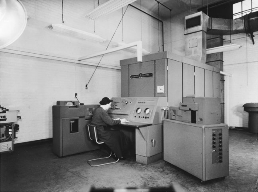
The DEUCE, the production model of the Pilot ACE, manufactured by the English Electric Company. This DEUCE, photographed in 1956, was installed at the National Physical Laboratory in 1955.
