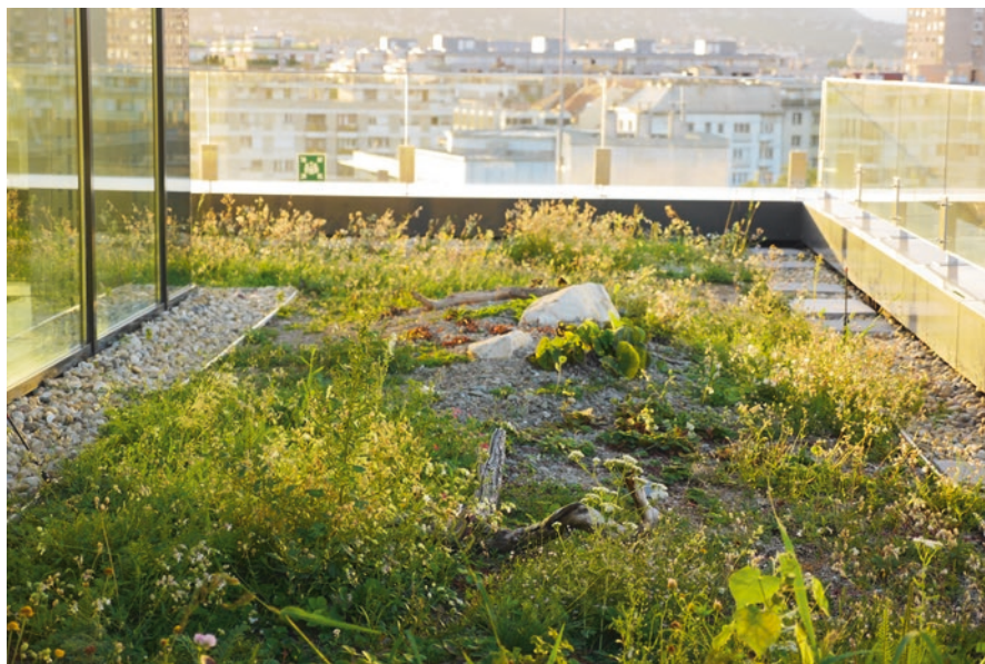
Fig. 10.16 A new and old concept for Biodiversity: LEED Platinum certified “Green House” Budapest, biodiverse hybrid Green Roof 7th floor (Source: Peter Dezsényi).
