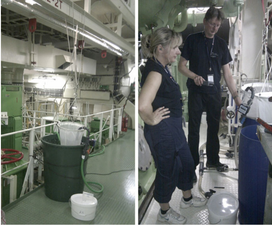
Fig. 14 Sampling arrangements for in-line sampling on vessels, on the left in a more open space, and on the right in more confined space of the engine room
