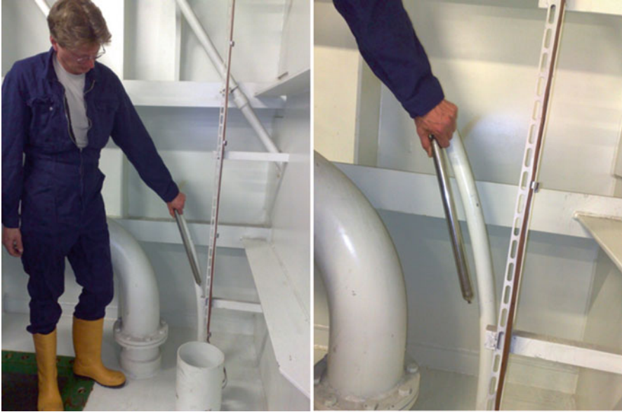
Fig. 12 Slightly bended sounding pipe on a car carrier which would not enable all sampling equipment described above to be lowered to the tank bottom
