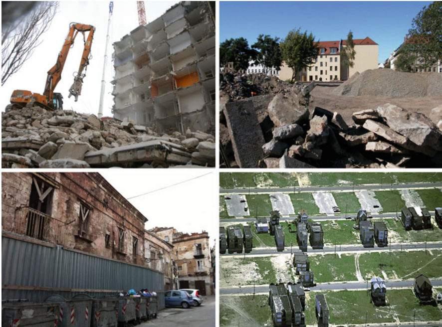
Fig. 12.3 Typical features of urban shrinkage affecting built space: under-use and vacancy of built infrastructure, demolition of buildings, creation of residential and commercial brownfields, and emergence of land-use perforation. Examples are shown from cities in Eastern Germany ( upper photos ), Poland ( lower left ) and the United States ( lower right ) (Photographs published with kind permission of © Google Earth 2013. All Rights Reserved)
