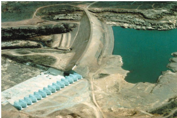
Fig. 7.6 Picture of an earth dam
