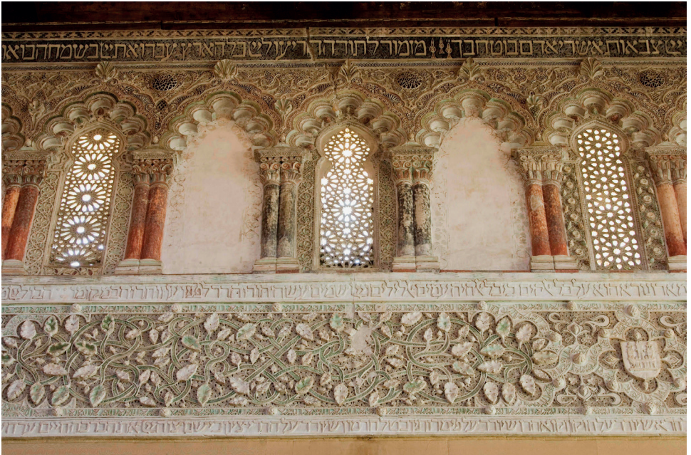
26. Stucco work in the interior of the El Transito synagogue, with monumental Hebrew inscriptions. The elaborate interior decoration is strongly influenced by Islamic artistic styles.
