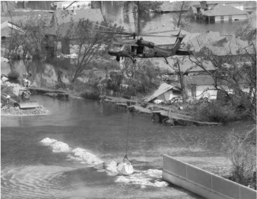
Closure of 17th Canal levee breach following Hurricane Katrina (After Seed, et al. [2005]; US Army Corps of Engineers Photograph)
